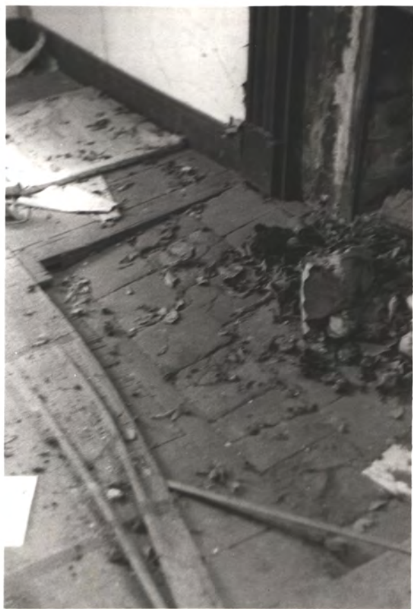
FL. 2 N.E. RM., E. WALL NOTE \pm 8^{\circ} NORTH BRICKS, HALF-BOND
