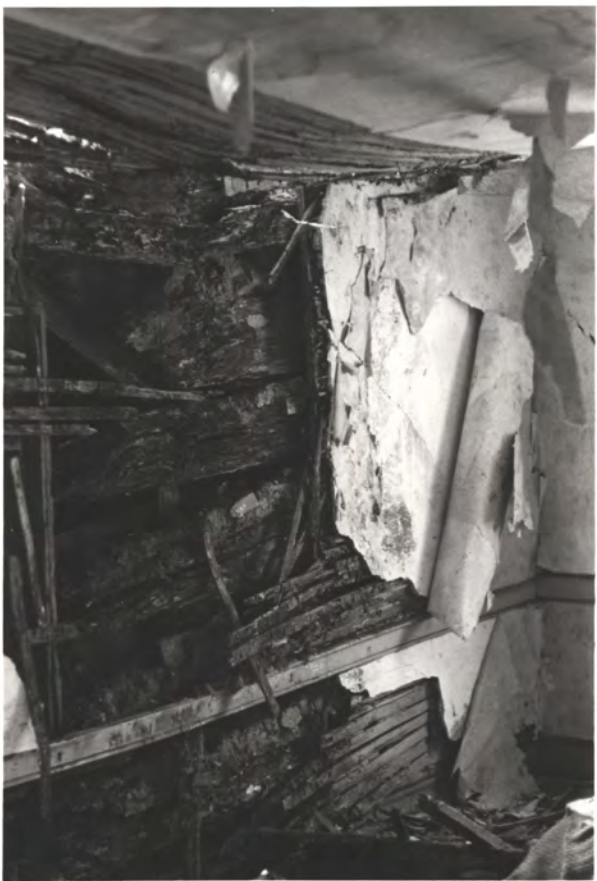
S. WALL OF N.W. RM, FL. 1 (logs, split lath, plaster)
