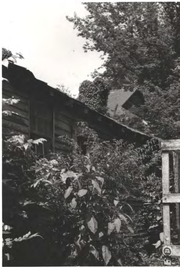
SEEN. BLDG. S. WALL - APPARENTLY NO BOX-CORNICE EVER (?)
