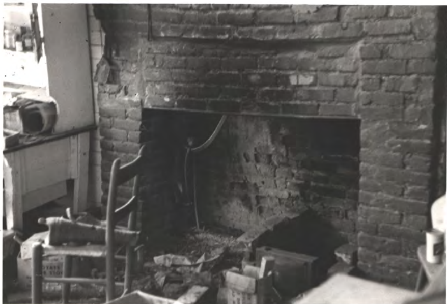
KIT. FIREPLACE in serv. bldg
