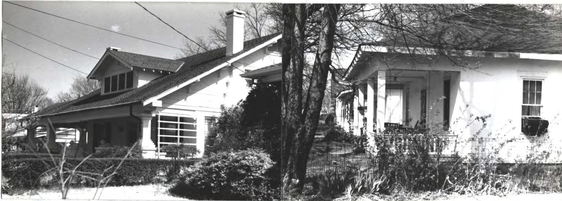
9. This 418 Locust Avenue 1922 bungalow exhibits the Swiss influence (long, low swooping roof, large dormer, stucco, false half-timber) but not in a literal manner. (3) Notice the "missing" porch columns - a deliberate design feature. It would be an error to "replace" them. This house was built by Fisk & Hopper, contractors. Its design probably came from a "bungalow book" of stock plans.
