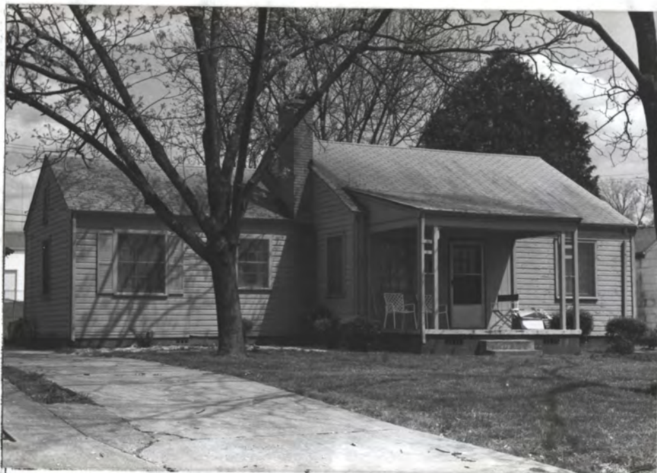
13. A large subdivision of houses similar to this one on Sewanee Road were built in the early 1940's during World War II to house Redstone and Huntsville Arsenal workers. Its style is derived from old New England cottages, except with a front porch added, and thus could be called a "Cape Cod Cottage" revival style.
