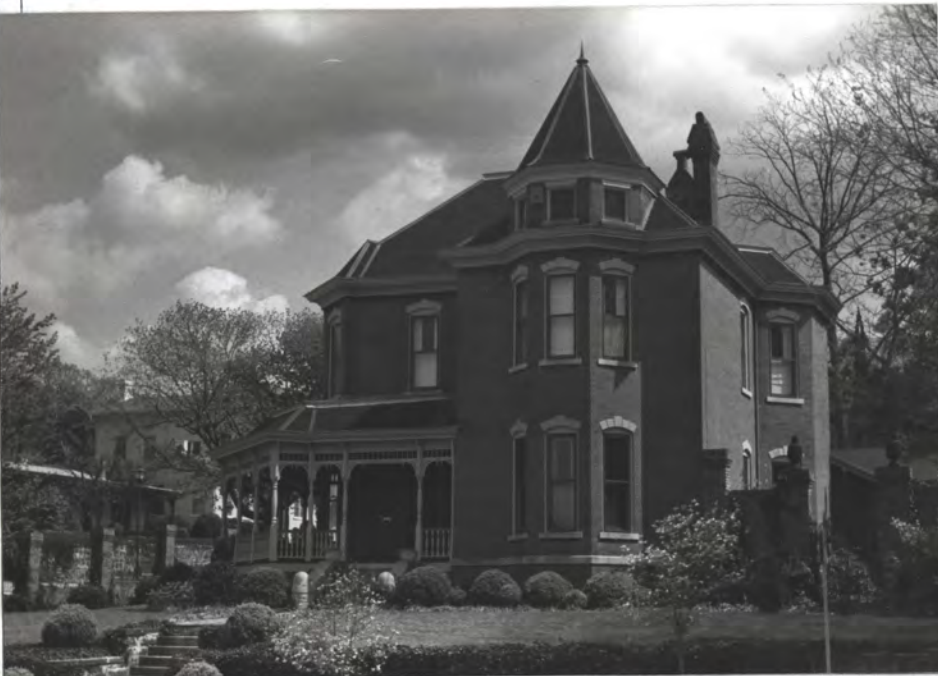
1. This 1899 house at 308 Eustis Avenue illustrates that the Victorian styles held sway right up to, and partly into the 20th century. This Eastlake-style house is of unusually fine detailing and workmanship. The pressed-brick walls have extremely tight, barely visible mortar joints, for the objective in brickwork of this period was for the wall to appear as monolithic. The architect is unknown.
