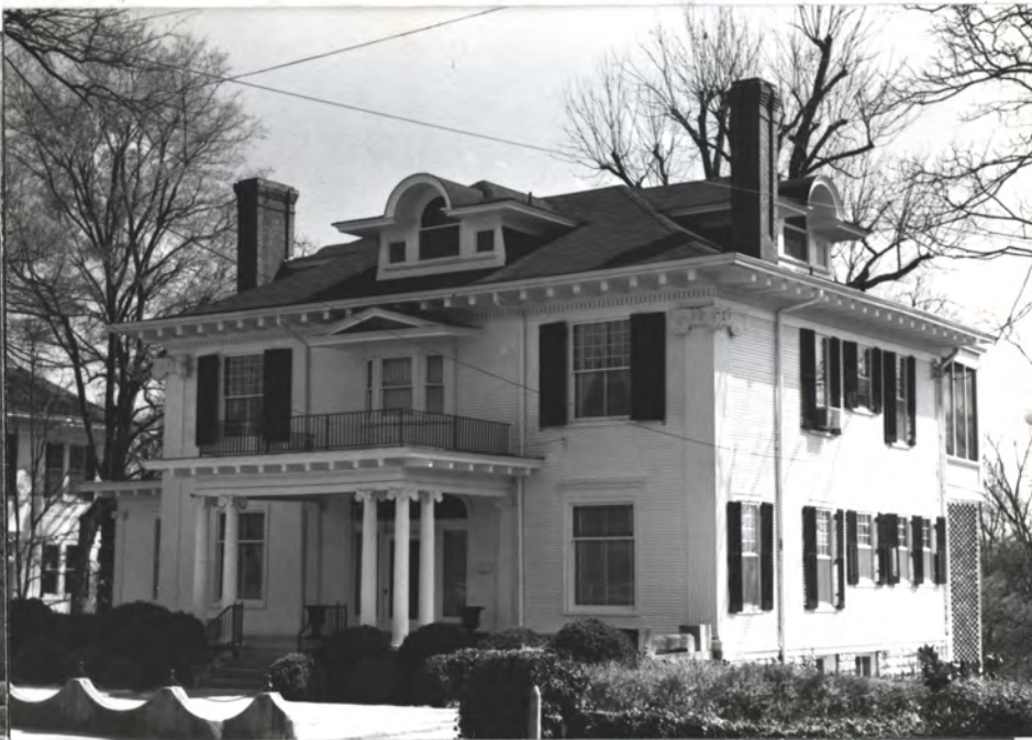
4. This 1907 house at 418 McClung Avenue is a free adaptation of the Colonial Revival style. While the basic design is technically Colonial Revival (boxy shape, hipped roof, fanlighted & sidelighted entry, modillions, Palladian dormer, sash-blinds, etc.) the proportions are vastly different from the late-Georgian ancestors of this fine house. The roof eaves are about three feet wide-over three times as wide as those of an 18th century Georgian house. The modillions at the eaves are gargantuan in comparison to 18th century ones. On the other hand, the clapboards are extremely narrow, about one-third as wide as in the Georgian period. All this disregard for academic "correctness" comes off splendidly, and the result is an excellent early 20th century house instead of a pale copy of an 18th century one.
