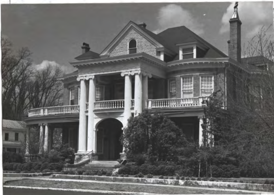
3. This finely-detailed, well-constructed ca. 1902 house at 501 Franklin Street was designed by the architect Herbert Cowell. It is an amalgam of mostly classical elements such as Ionic fluted columns, Adamesque frieze, modillioned cornice, balustrades etc., with some holdover influence of the Victorian period as seen in the broken flowing massing and the chimneys with vertical inset ribs - a Queen Anne device, as is the pebble-finish tympanum and use of stained glass. This house is a very free, unacademic expression of predominantly Colonial Revival elements which might best be called "Free Classic" in style, a recognized term of the period.
