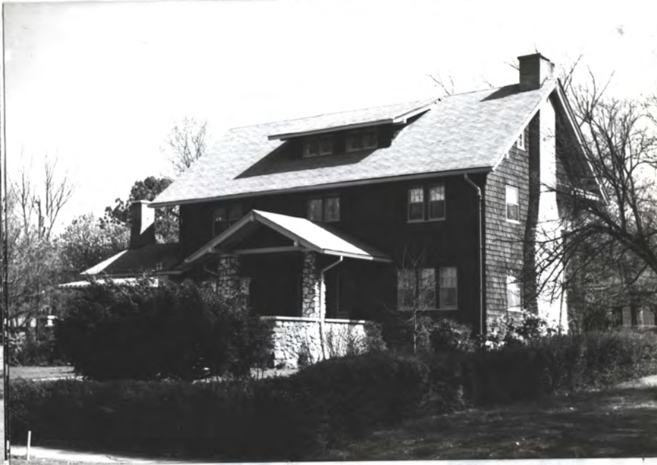
6. This 1914 house at 612 East Holmes Avenue could be termed a "Swiss style bungalow". It bears a strong family resemblance to many 17th and 18th century Swiss rural houses, with its use of fieldstone, natural wood shingles, and steep gabled roof. The wide, low shed-roofed dormer is also found on old Swiss houses. (3) These Swiss forms, including the use of rough-cast stucco and false half-timber, are found on many bungalows and it would be fair to say that old Swiss houses were a major influence on the bungalow style.
