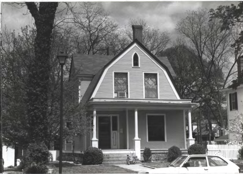
2. This 1901 house at 603 Franklin Street by the architect Herbert Cowell has a Dutch-Colonial Revival gambrel roof combined with late-Victorian massing (vertical, narrow, irregular). A small "Gothic" vent is in the gable. The windows are quite wide and squarish in proportion, unlike those in the Victorian styles. A balustrade once ran along its porch roof, as evidenced by the base for it, and there may have been a balustrade also at the porch floor level that ran between the masonry piers which support the porch columns.
