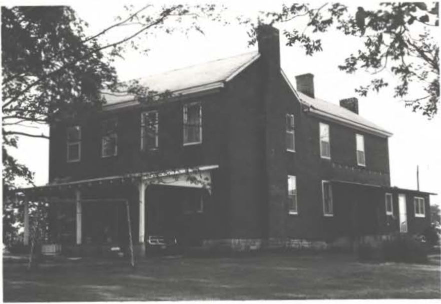
S. FRONT (ADDED PORCH)
