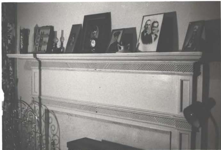
1ST FL. S. E. (PARLOR) MANTEL = FED.
