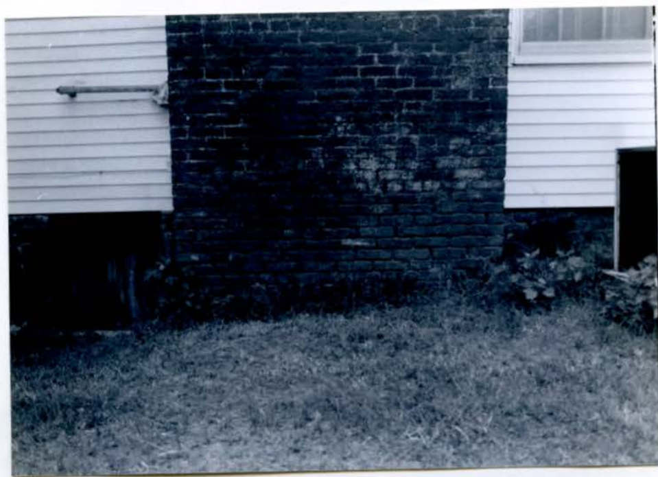
VIEW OF SOUTH FOUNDATION SHOWING CELLAR DOOR CHIMNEY AND BRICK FDN
