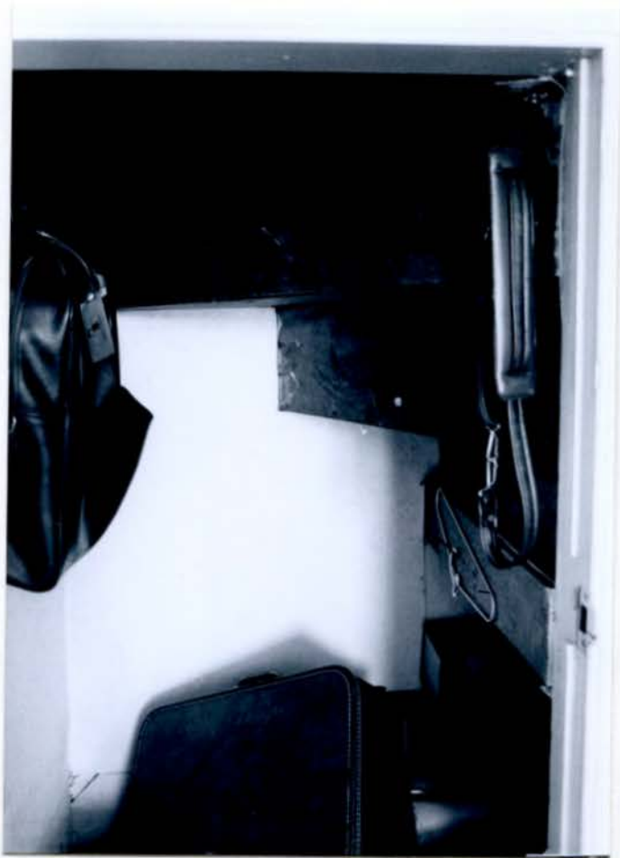
CLOSEUP OF CLOSET UNDER ATTIC STAIRS SHOWING STAIR CONFIGURATION
