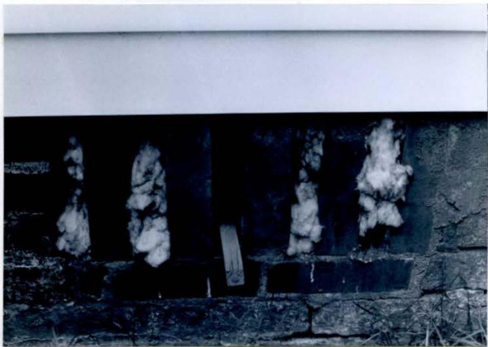
DETAIL OF VENTS IN FOUNDATION - NOT ORIGINAL
