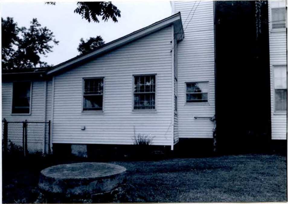
CLOSEUP OF ADDITION (NOW LAUNDRY ROOM)
