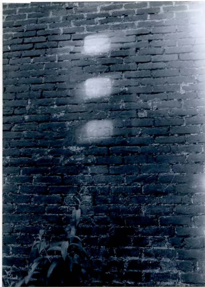
CHIMNEY SHOWING COMMON BOND PATTERN
