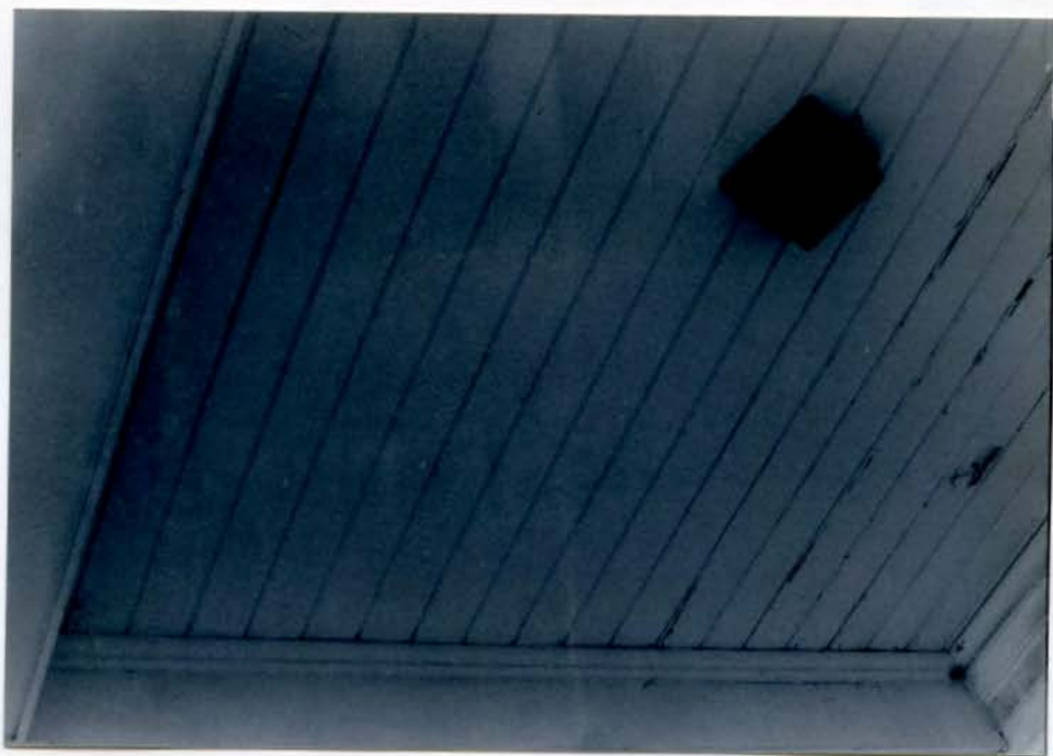
DETAIL OF CEILING OF FRONT PORCH (NOT ORIGINAL TO HOUSE)
