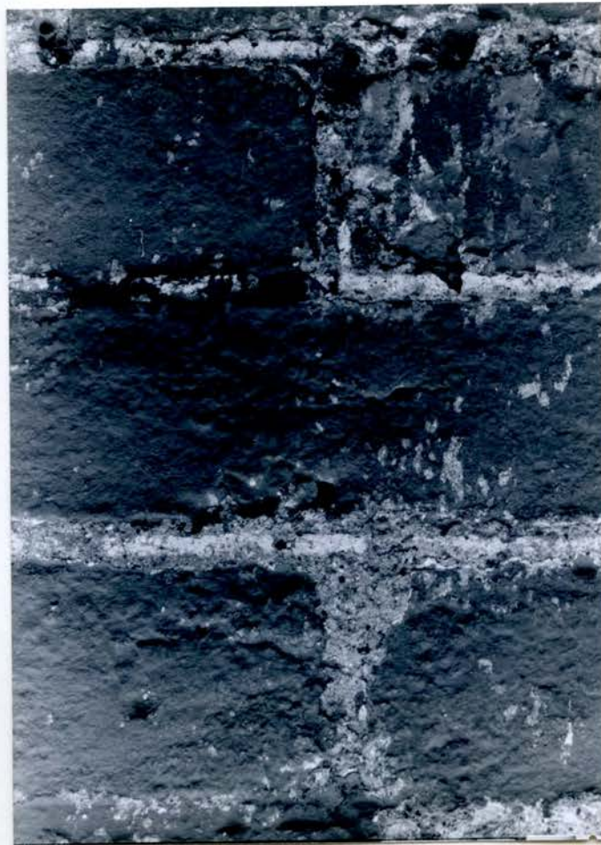
← BRICKS SHOW RED, WHITE, AND GREY-BLUE PAINT LAYERS
