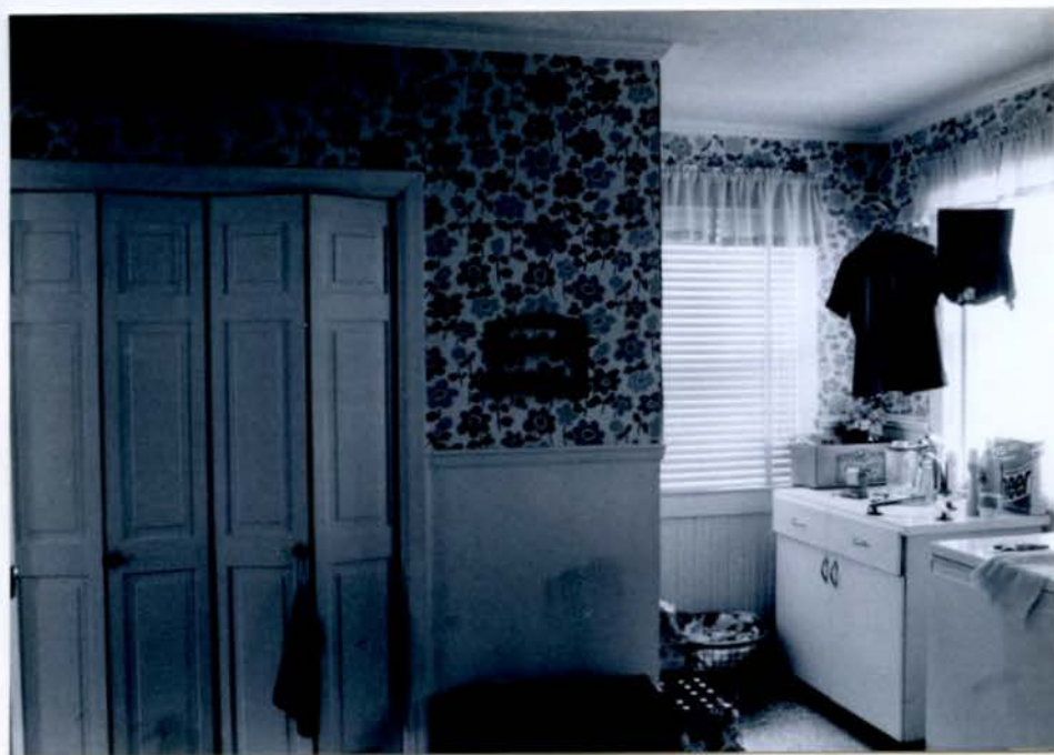
LAUNDRY ROOM - EAST WALL - CLOSET IS LATER ADDIT ON
