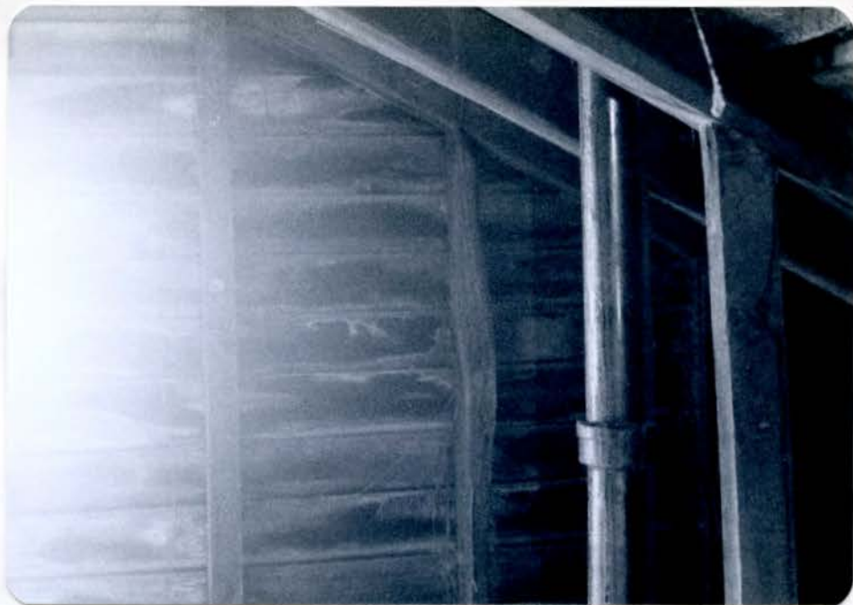
ATTIC - SOUTH WALL SHOWING CEDAR STUDS AND SHEATHING
