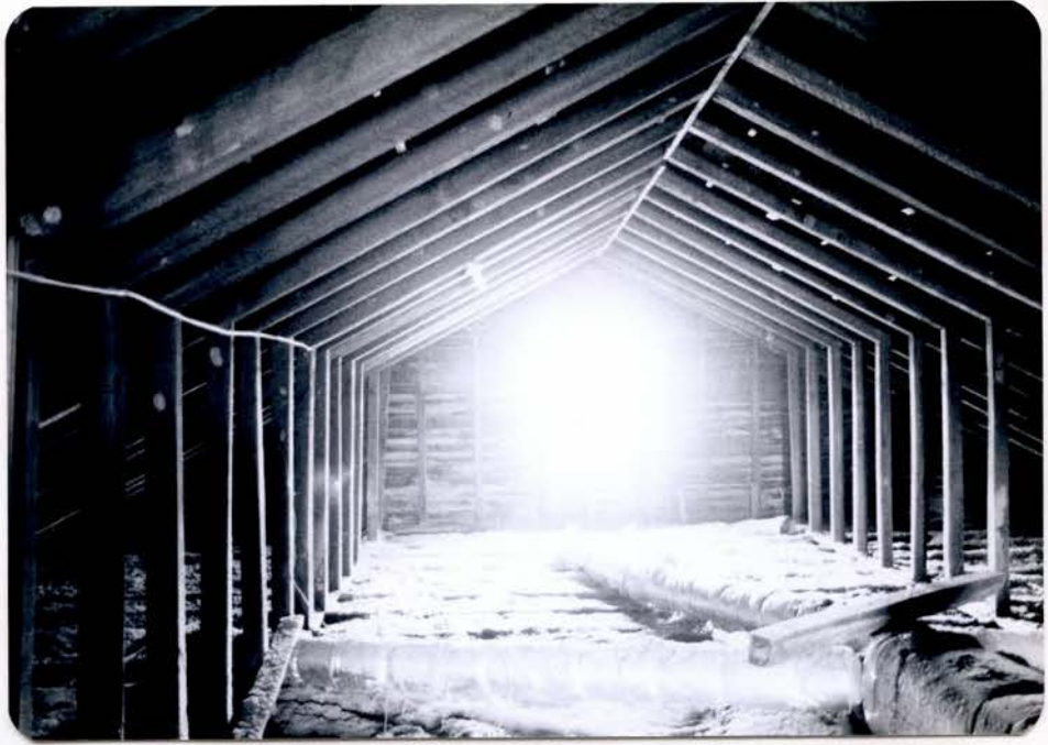
↑ ATTIC - NORTH WALL AND RAFTERS ↓
