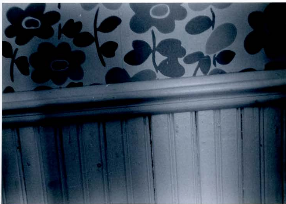
CLOSEUP OF WAINSCOTING
