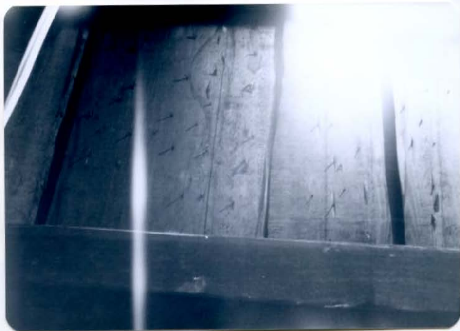
ATTIC - RAFTERS, SHEATHING AND ROOFING NAILS
