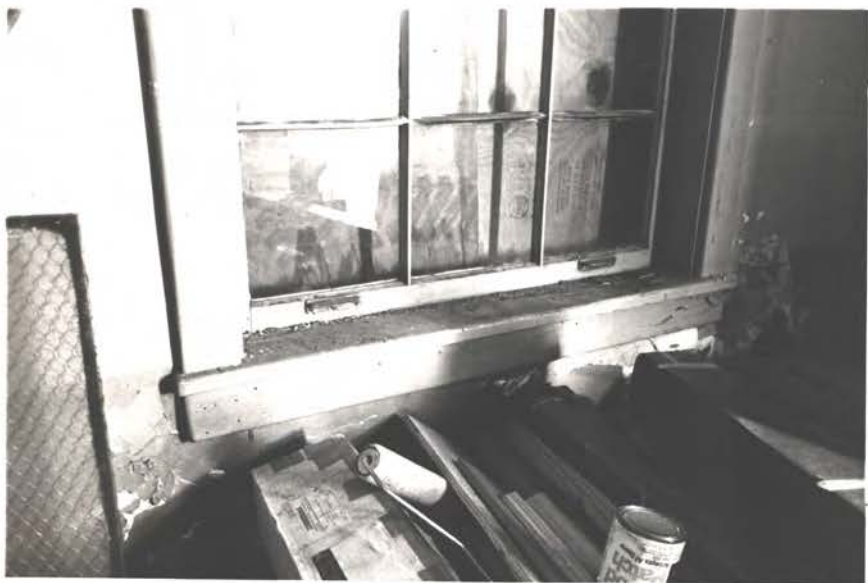
Window @ East Wall
