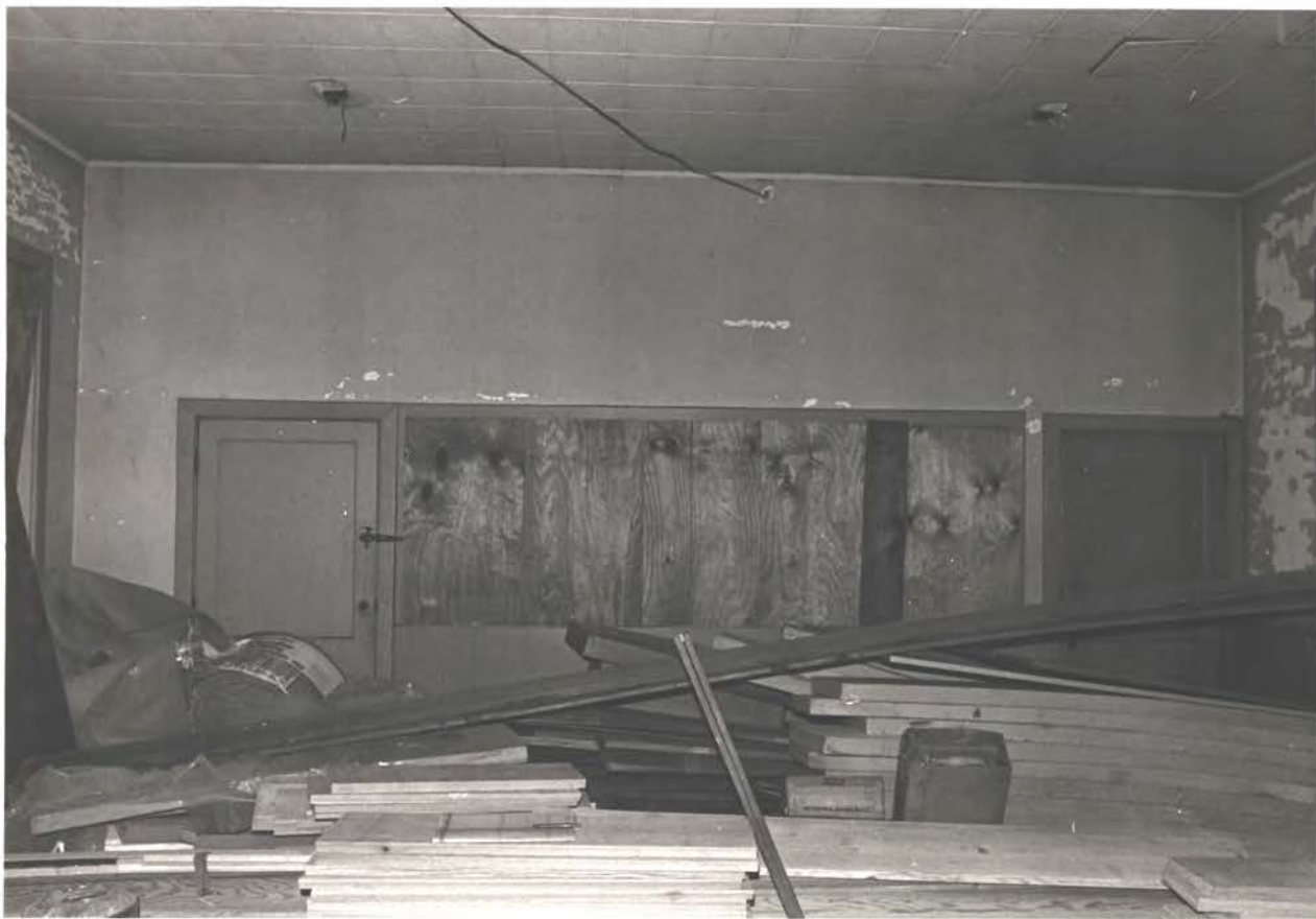
↑ EXPRESS BLDG., EAST ROOM, THE WEST WALL
