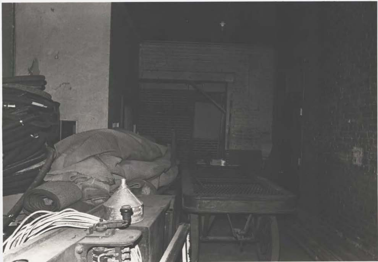
↑ EXPRESS BLDG., WEST ROOM, WEST WALL
