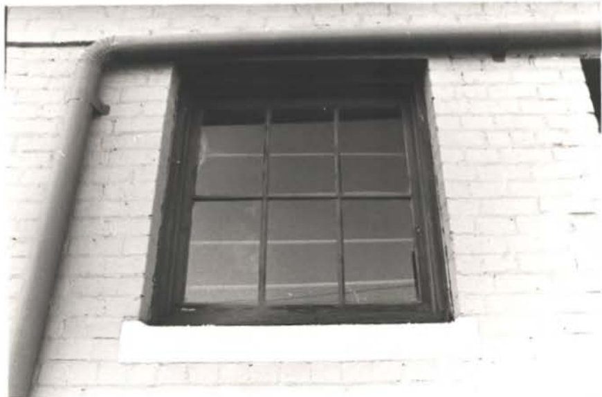
Window @ South Elevation
