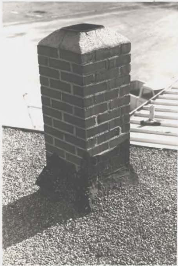
Brick flue from kitchen @ South wall. ← ↓
