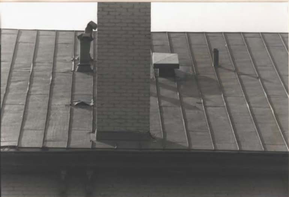
↑ S. CENTRAL CHIM. (REBUILT W/ VERT. STL. REINF. + CONC. CORE IN 1976)
