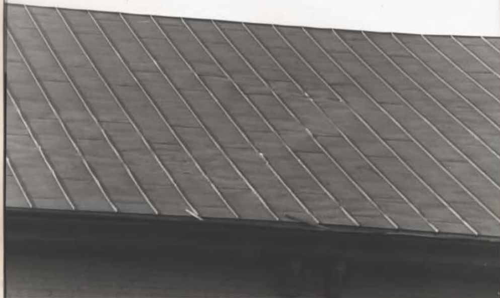
↪ DIMPLED & BENT SEAMS AT S. ROOF (TYPICAL)
