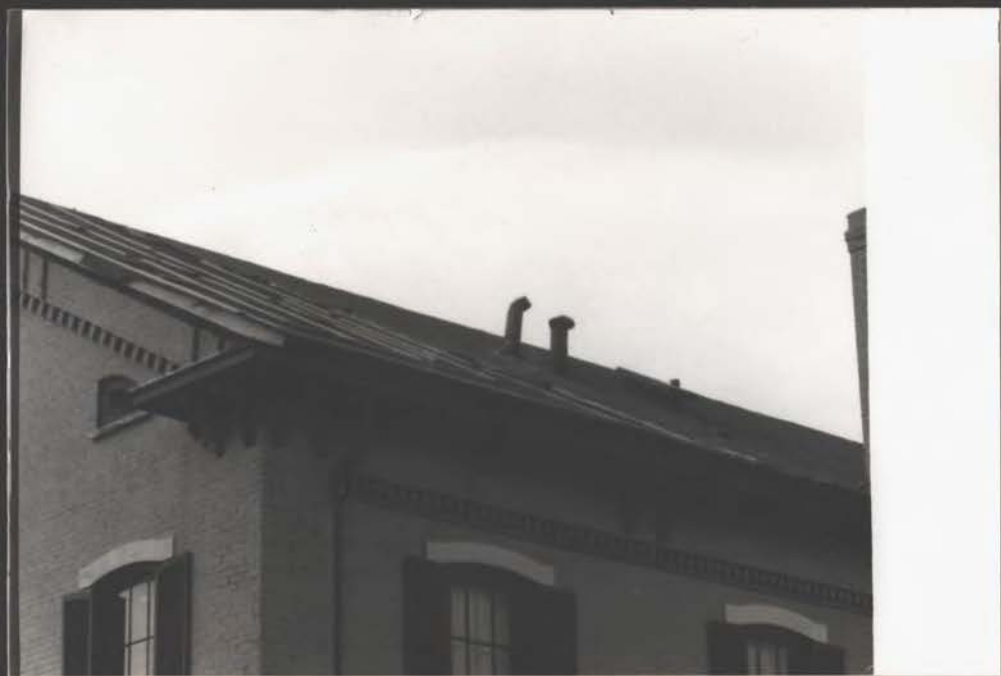
N ← S.W. CORNER ROOF PITCHED, WEST CORNICE HALF-BLOWN OFF
