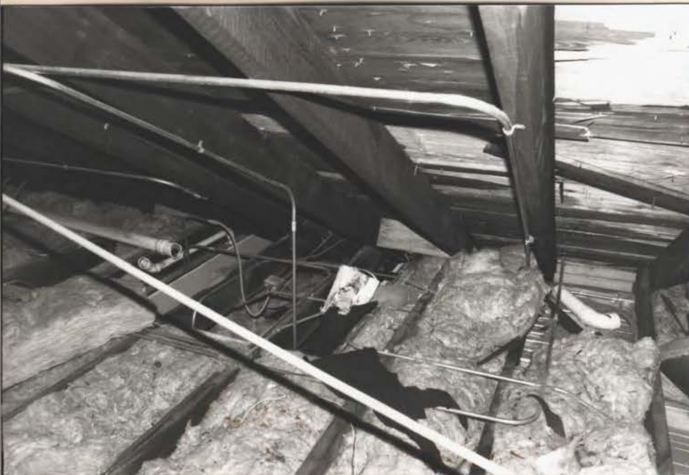
two pipes broken (vents)
