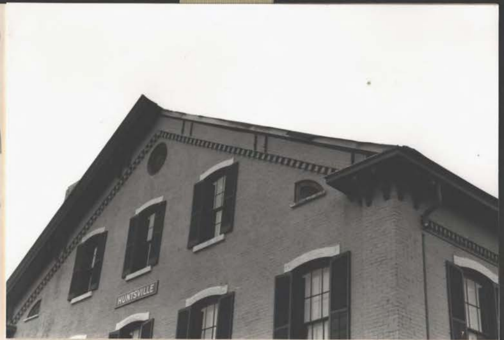
N ← CORNICE BLOWN OFF CORNICE BACKED BY WIND S.W. CORNER
