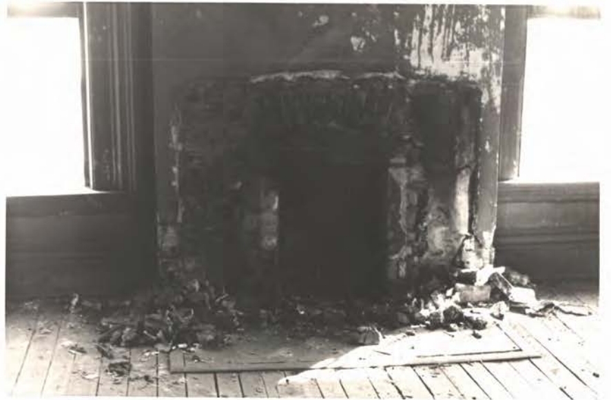
FIREBOX IN S.E. 2ND FLOOR ROOM JULY 80 →
