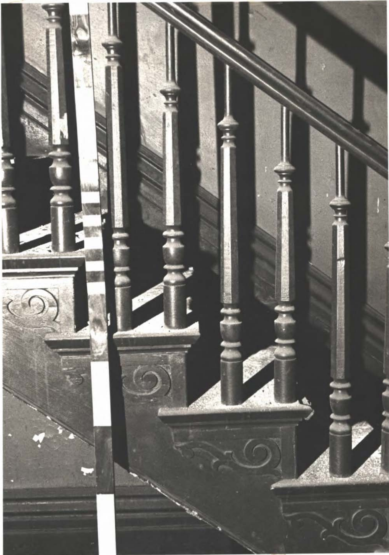
PHOTO #10 HUNTSVILLE DEPOT - 1978 Stair Detail
