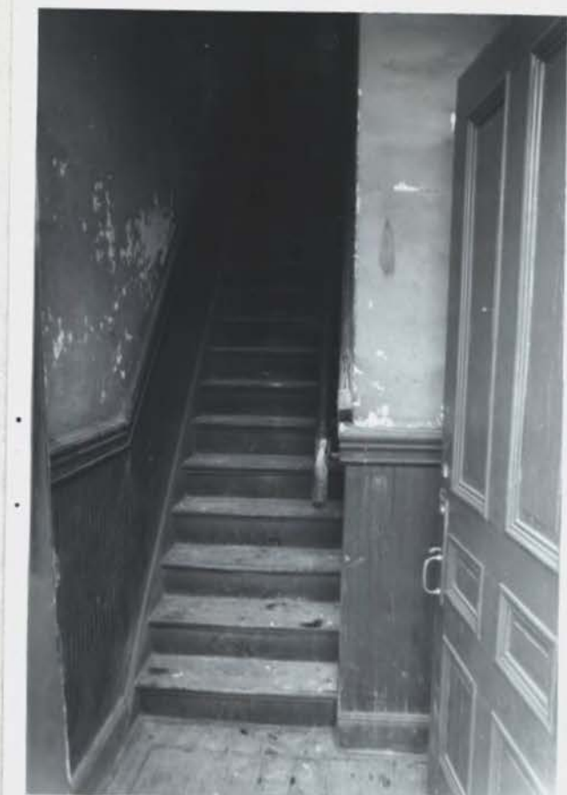
PHOTO #26 HUNTSVILLE DEPOT - 1978 Upstairs entry - Looking West
