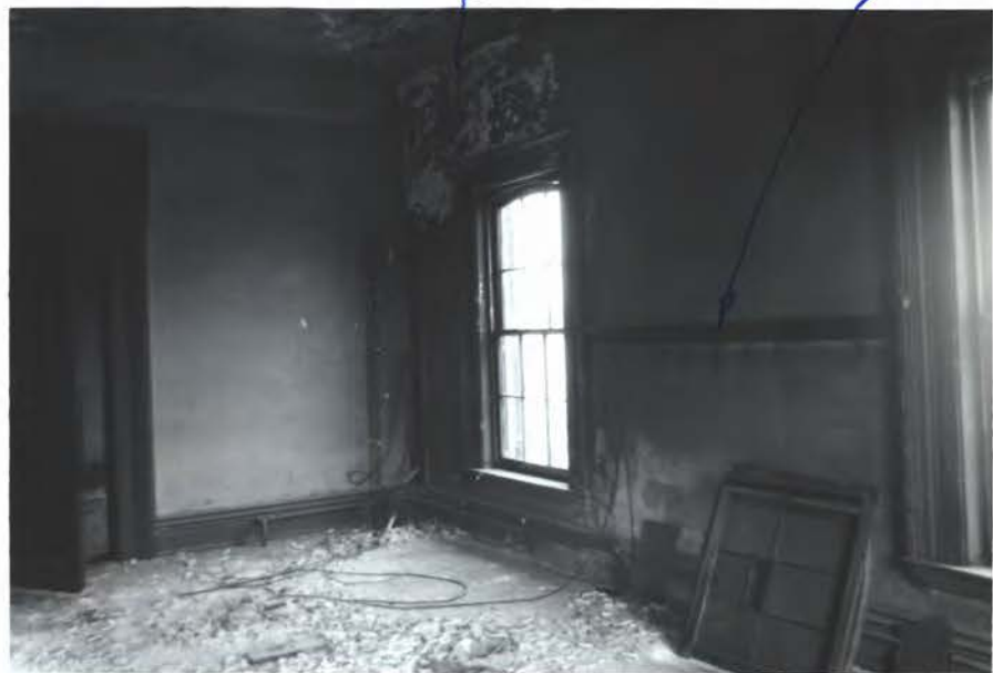
PHOTO #29 HUNTSVILLE DEPOT - 1978 Business Office One - Looking NW
