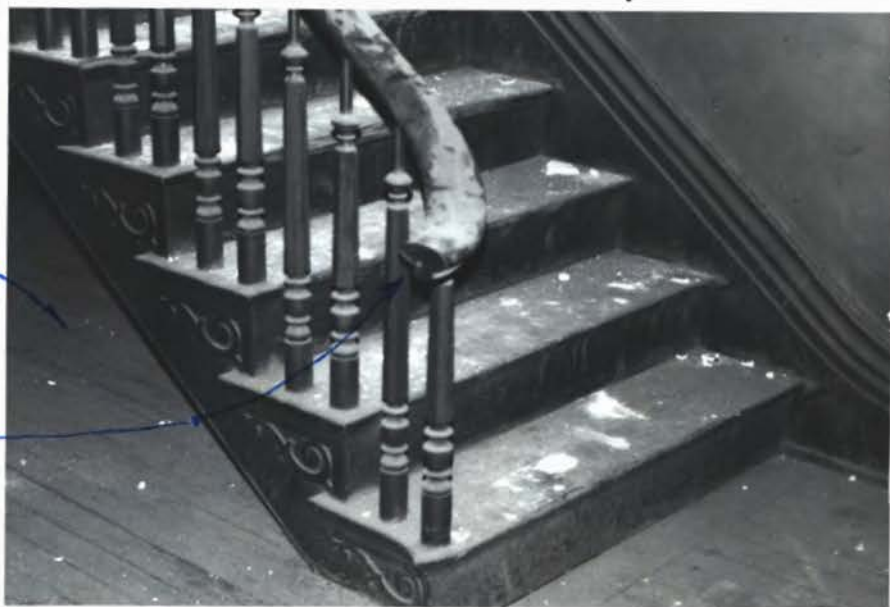
PHOTO #9 HUNTSVILLE DEPOT - 1978 End of rail at 2nd. Floor Stair
