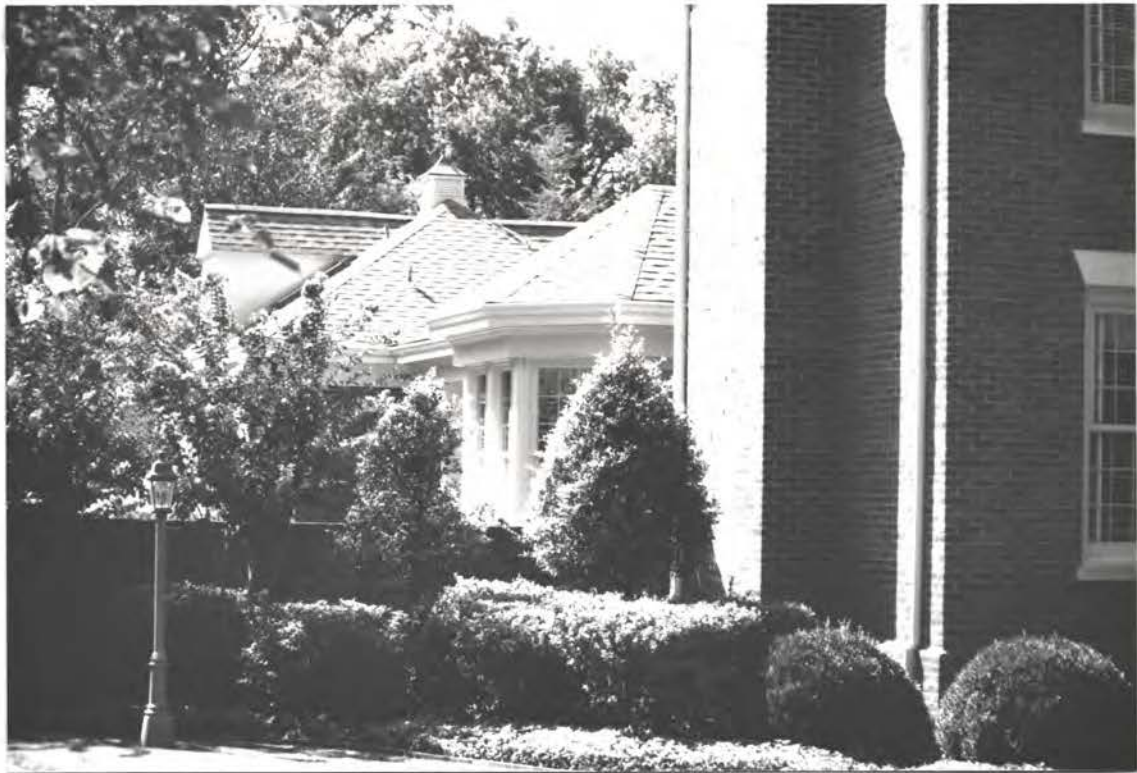
c.1995 hse at No. 8 Cruise Alley, Huntsville Al. Sept. 1997 photo after gar. roof raised for guest BR+Bath above gm. - J & H Arch, HJms
