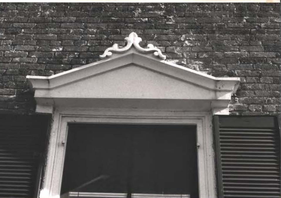
Hoods - metal (Ital) - no rust. Probably solid zinc.
