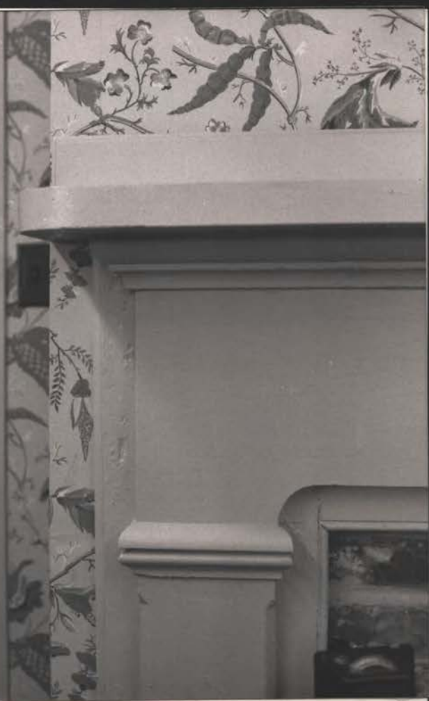
Fl. 2 stairhall - door to N.W. Rm - Ital. & (Fed. door, relocated from fl. 1)
