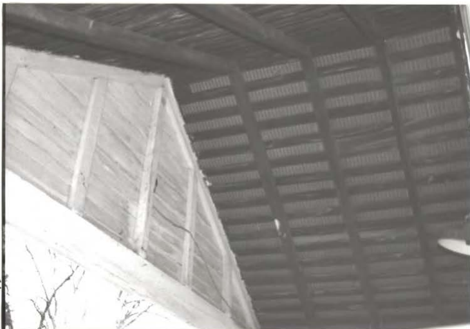
S. porch roof - framing could be early 19th c. (may be reversed) Dark strips are c. 1900 or later
