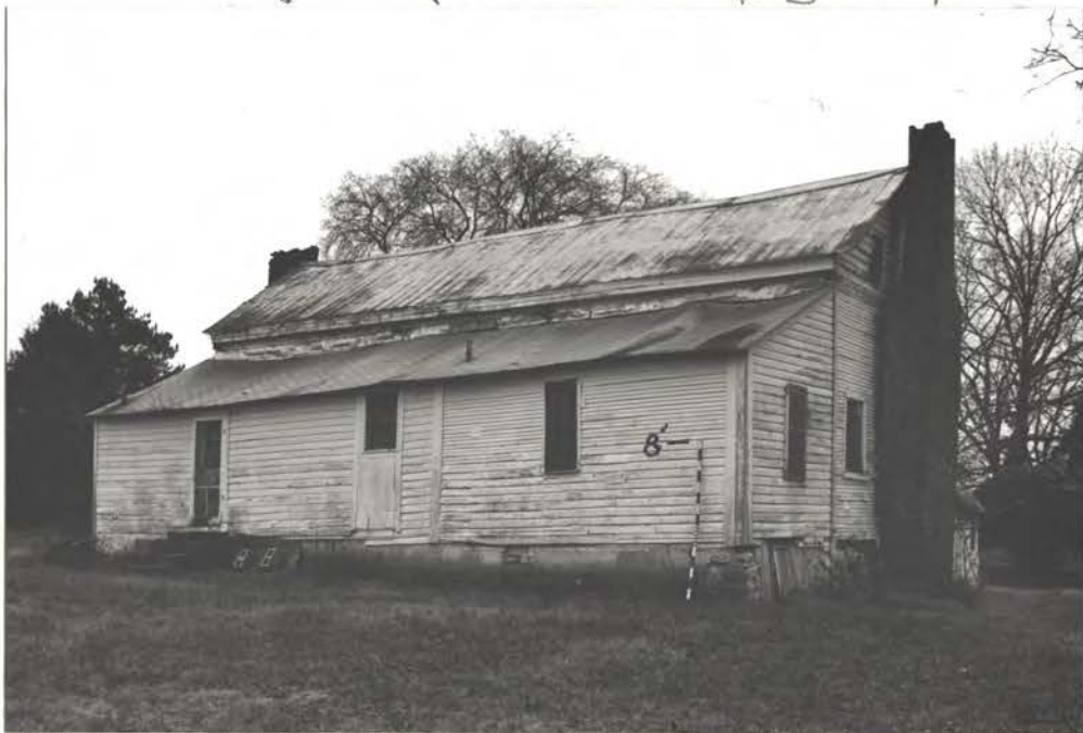
N. stack = small enclosure w. chim. leans ± 8'
