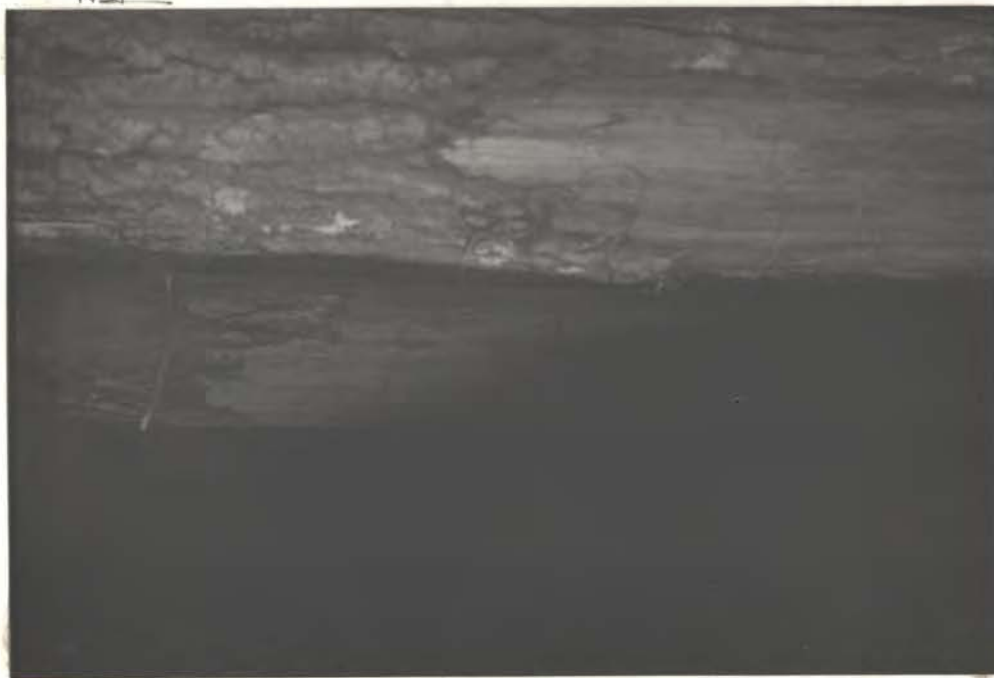
Punchon joists under W. per fl., ± 8'-10'
