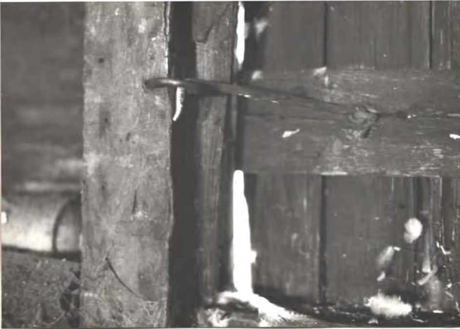
door to roof (at rear south wall) wrought iron handmade latch -note twist in shaft
