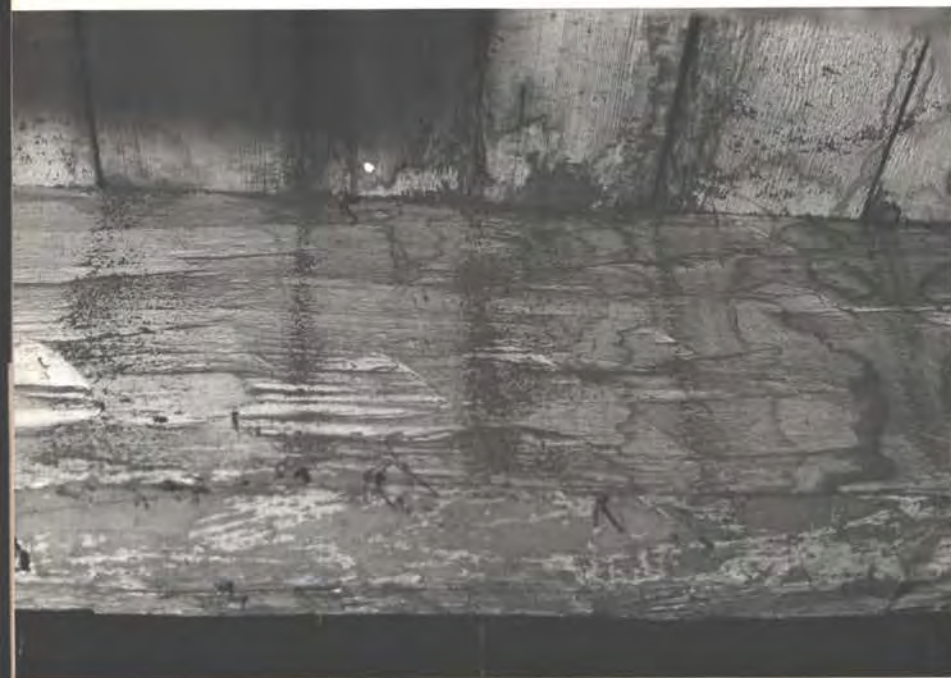
hewn joist face (broadaxe) opp. face is pitsawn
