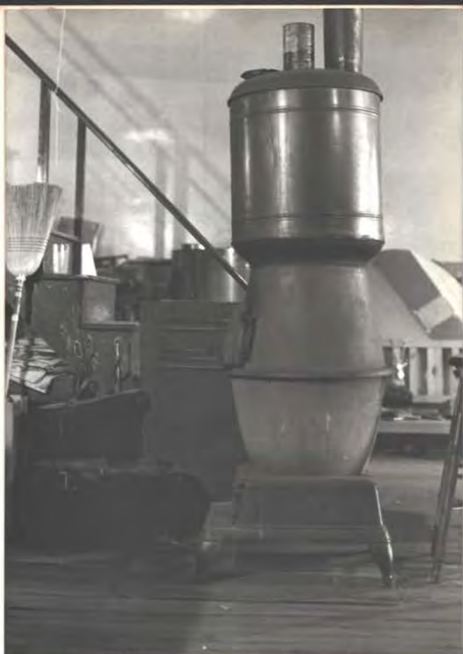
West bldg rear, look west (stove is near desk at left)
