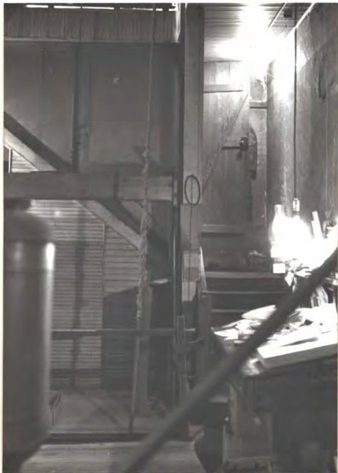
elevator + stair - look east Main fl. of east bldg.
