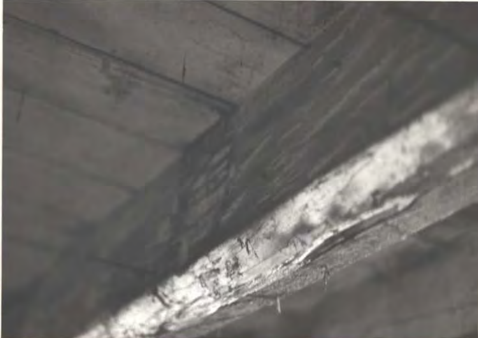
hewn joint, sashyawn fl., (other joint faces = pit-sawn.)
