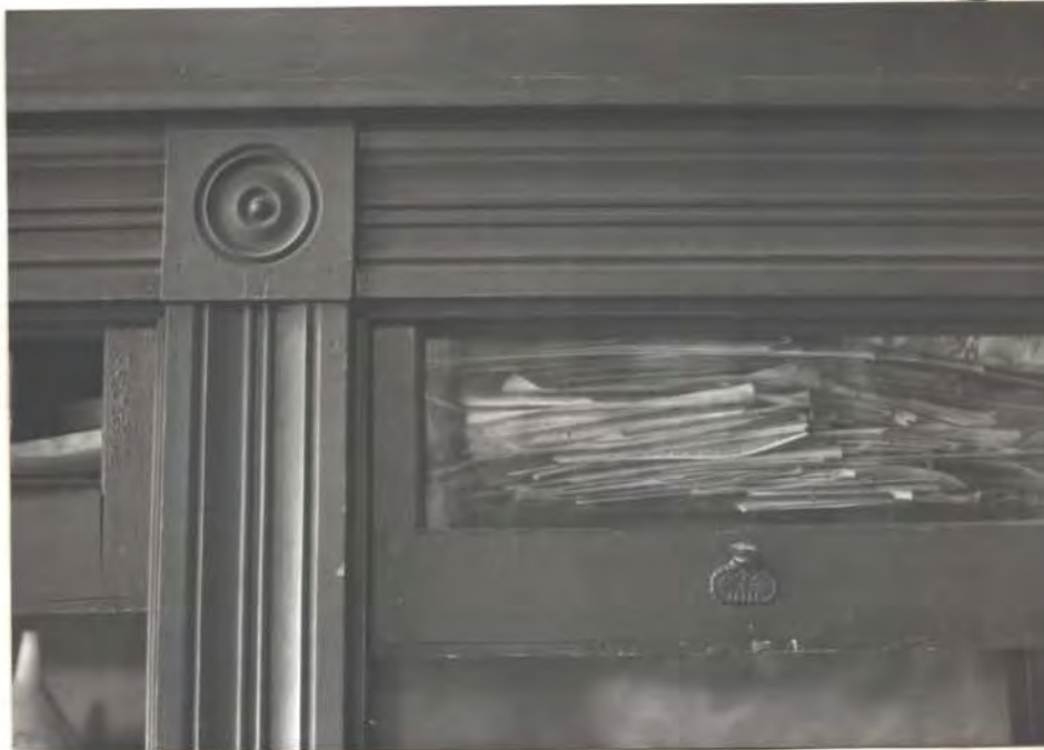
east wall cab.
