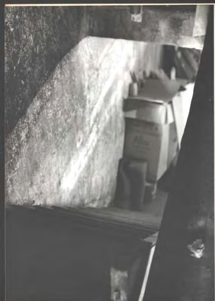
look dn stairs to 2nd fl. N at
