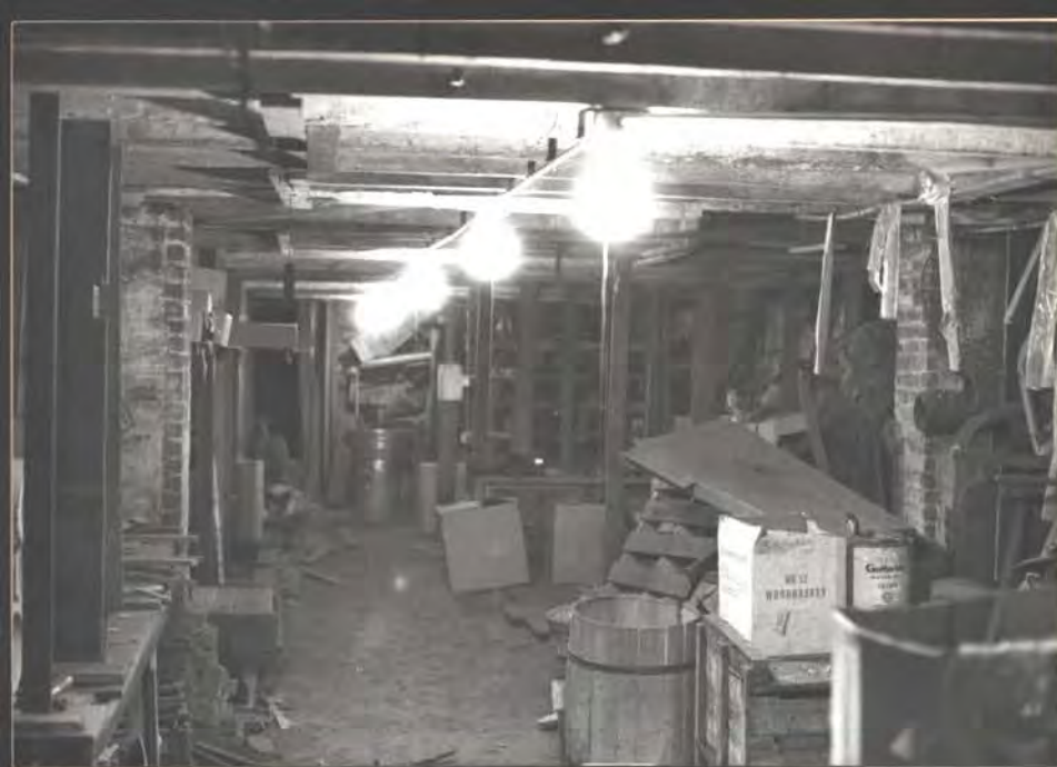
East (verify) basement looking N.
