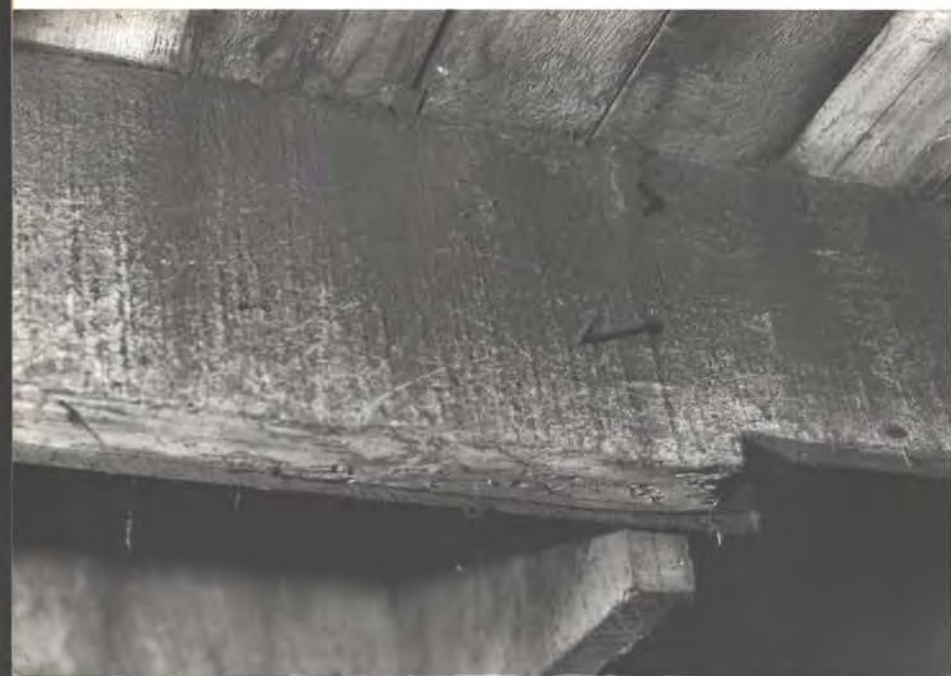
pitsawn joist + \frac{5}{4} " flooring is sash-sawn
