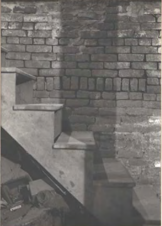
Stair, East basement (look E.)
