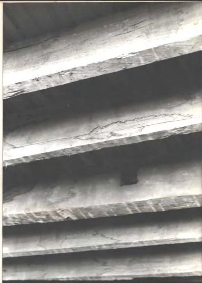
pit-sawn fl. joists + traces of lath & plaster cell.
