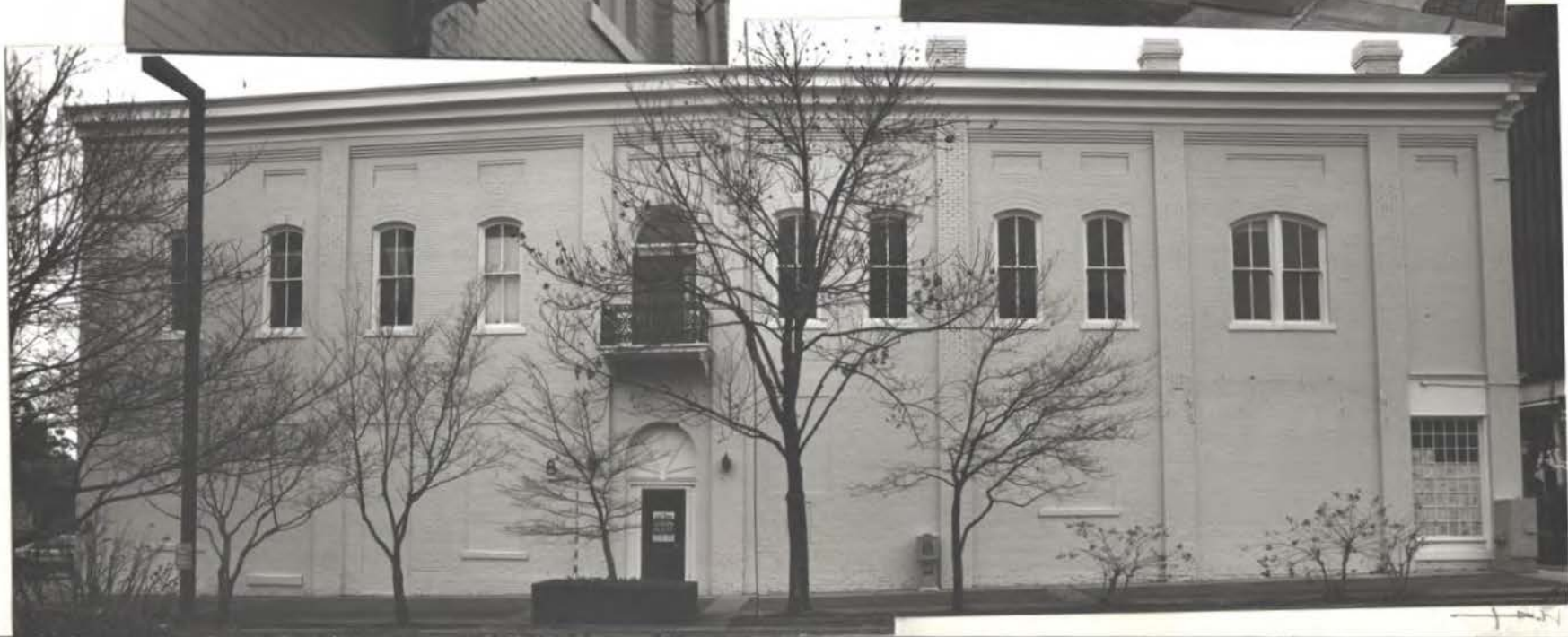
Note several windows & doors bricked-up in 1963 by bank ↓
