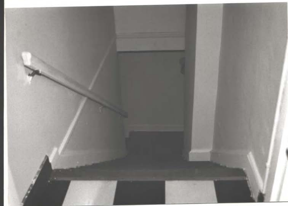
S.W. stairs, down from fl. 2 → S
