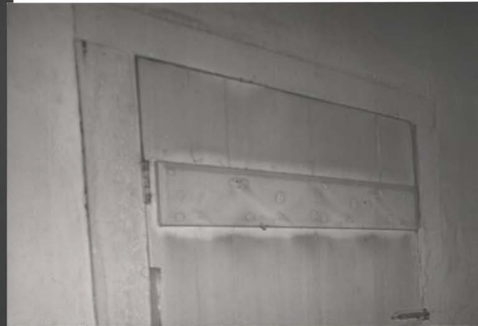
H → East door, Center rms. (original)
