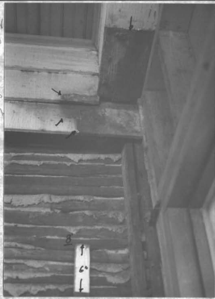
S.W. corner of enclosed porch
