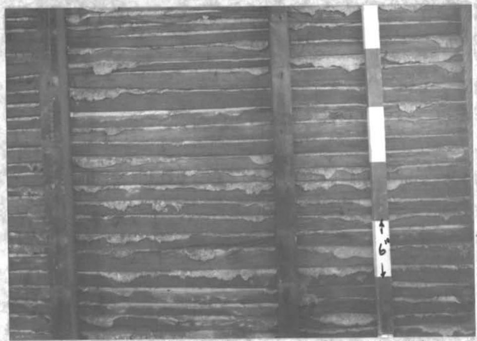
1850's N. Wall of N.W. Rm. (clapboards removed by Geo. King - mistake.)
