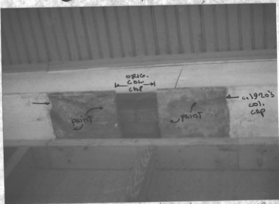
N. Wall of enclosed porch - LOOKING UP
