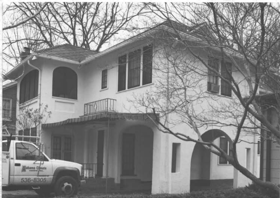
Feb. 1996 photo with ugly c.1950's metal awning (H Jones photo)
