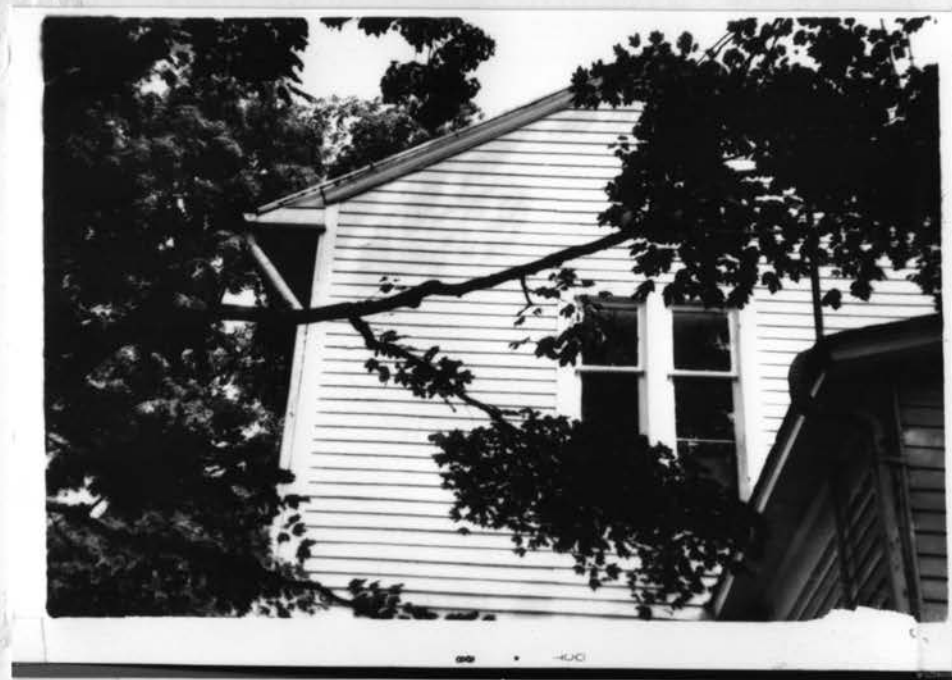
west rear gable
