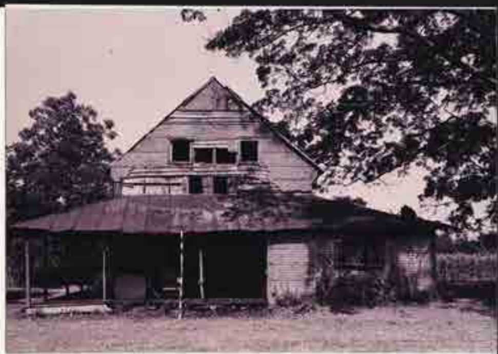
E. Chimney gone, doors put in chimney-hole -> N
