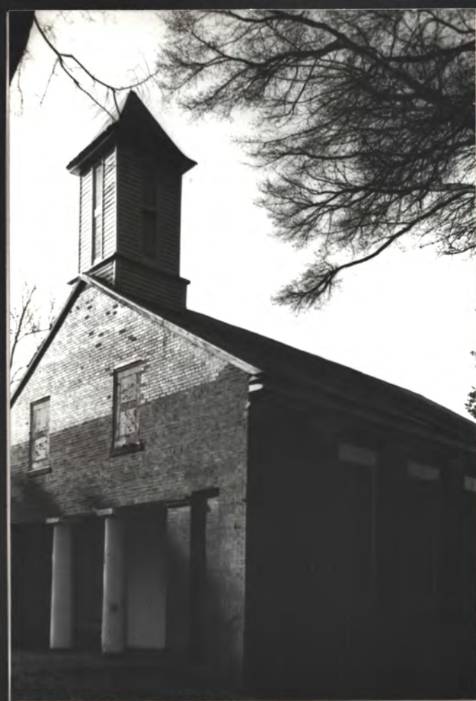
S. front & east side
