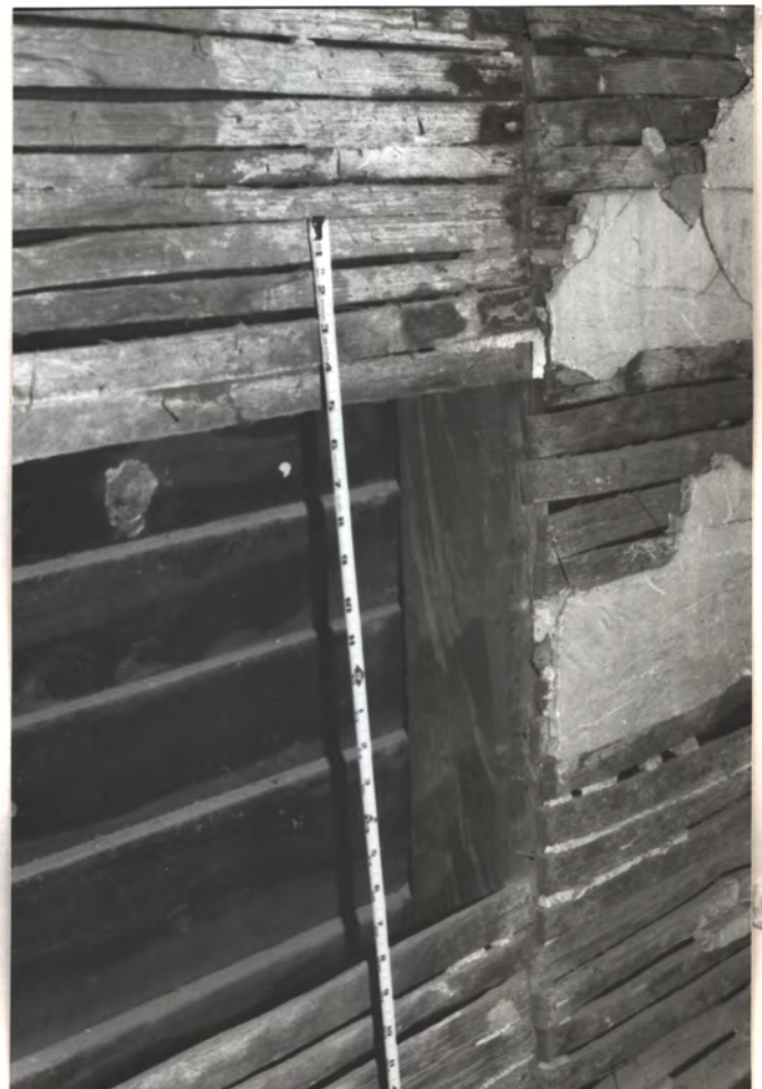
N. Handsplit bath, beam stud, hair plaster
