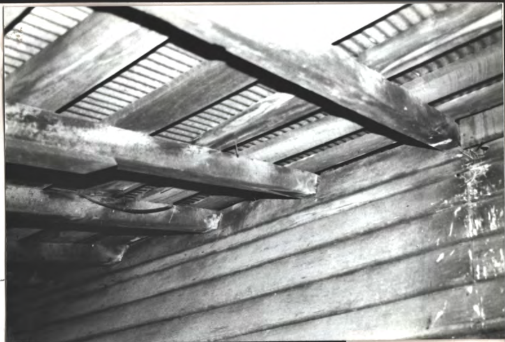
c. 1825 rafters = ± 3" x 4" + c. 1825 saw marks (plf sawn)
