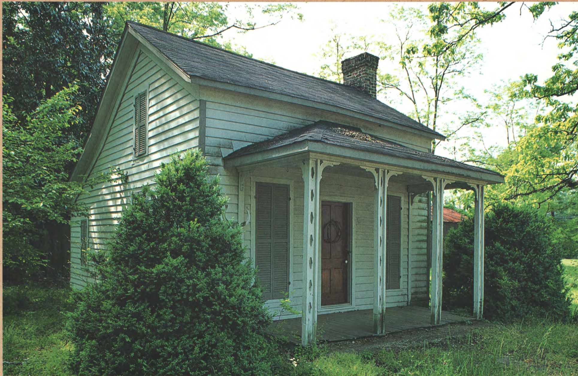
Simmons Cottage ca 1870 Limestone County
