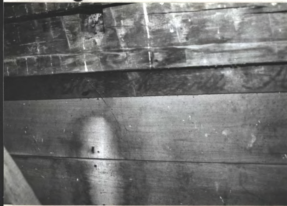
PEBBLES - MOORE'S VILLET, AL (reused packing - crate lumber)
