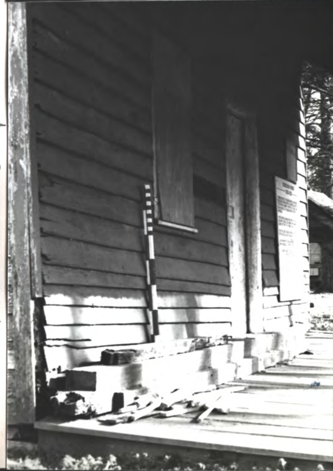
c. 1825 plf-sawn clapbds remain under porch only
