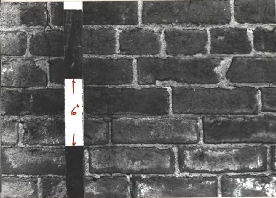
West wall ("NO. 2" quality bricks, common bond) (N. wall same)
