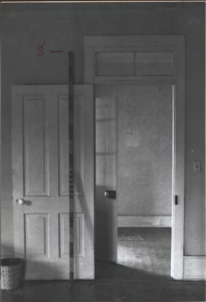
09- S.W. Rm Looking to entry
