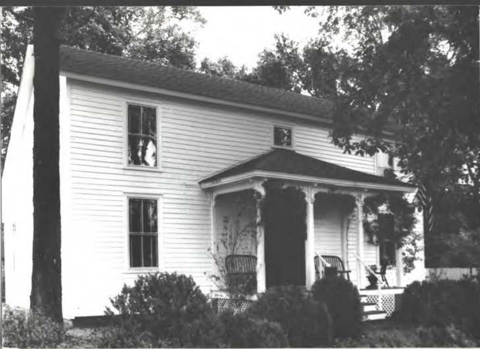
MAIN HSE, S. FRONT (restored by J&H, ARVH - Adams in c. 1986)
