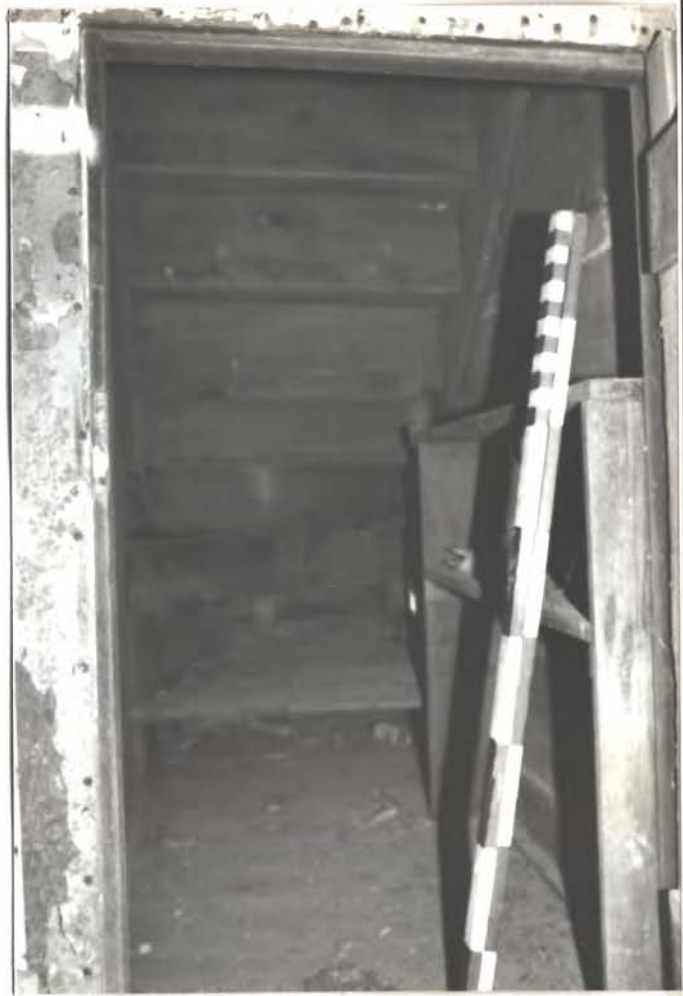
↖ Clos. under stair
