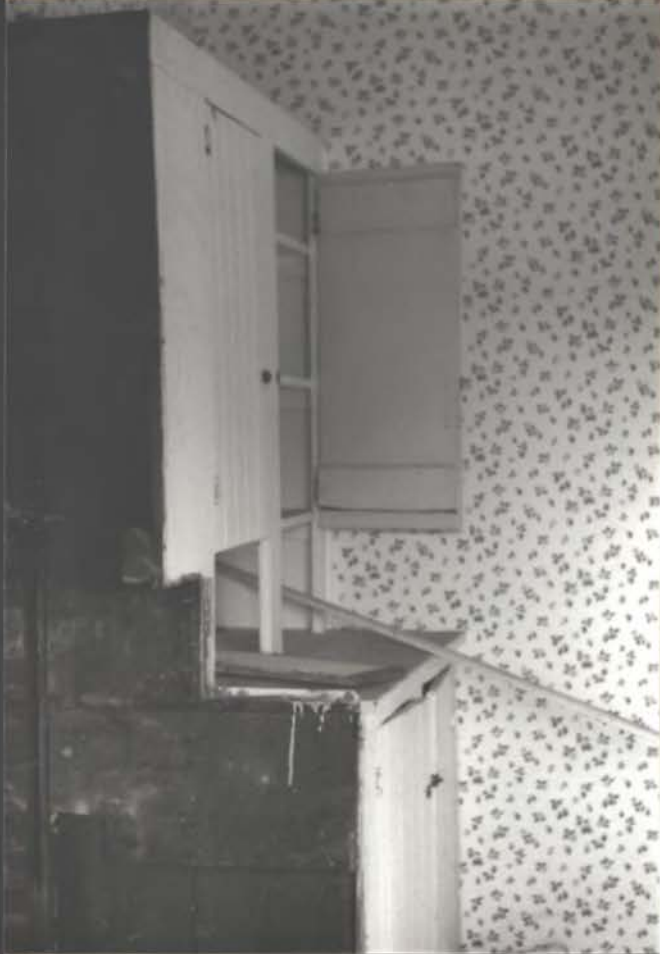
Original cabinets at S.W. corner, S. wall (no lath or plaster traces on studs behind)
