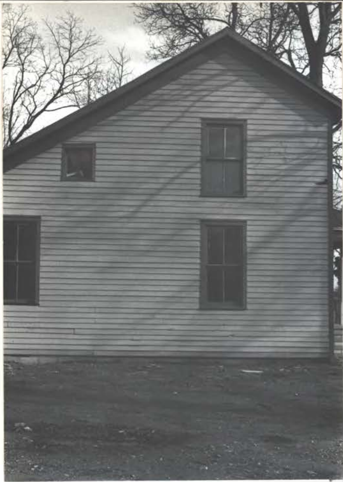
west - note clapboard exposure varies 1 inch or more = typical
