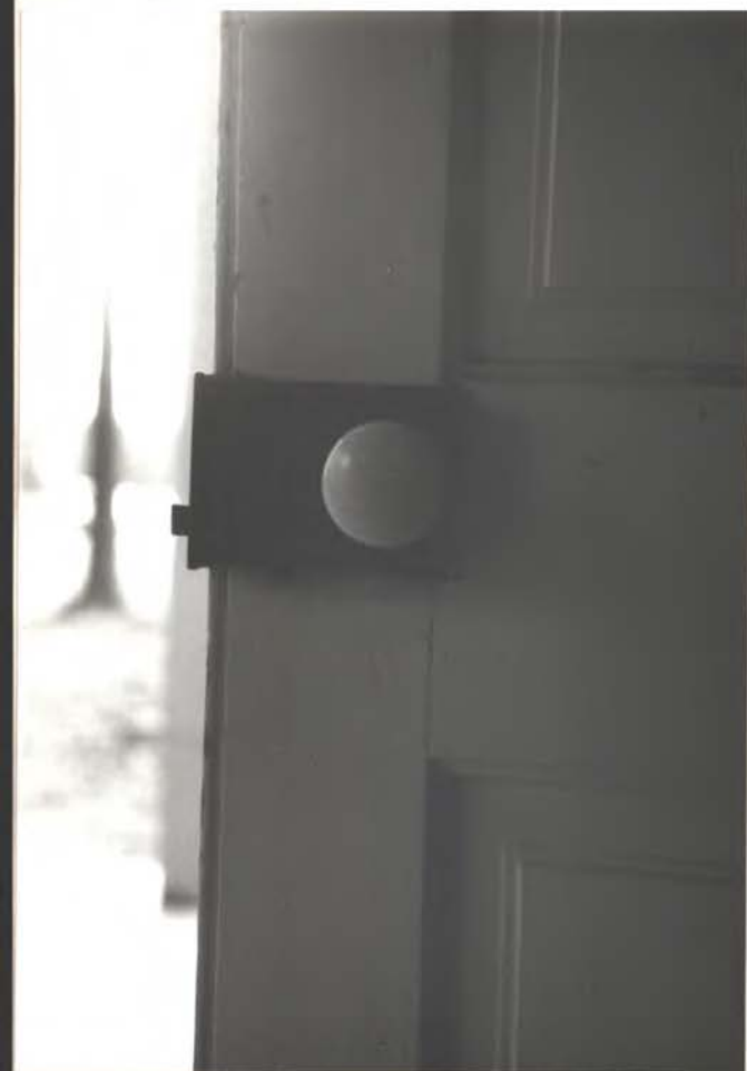
orig. rimlock on entry doors Patent-dated 186 - (2? 3?) - white cer. knob
