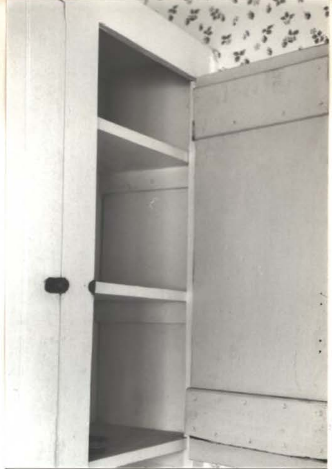
Original cabinets at S.W. corner, S. wall (no lath or plaster traces on studs behind)
