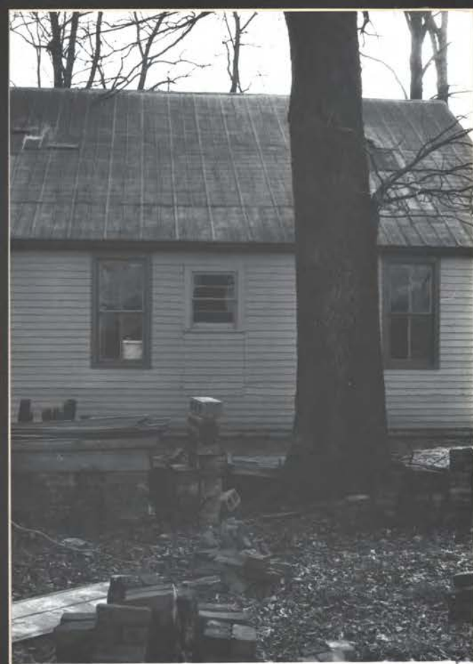
galv. iron roof = modern North Orig. = wd. shingles - see "descrip"
