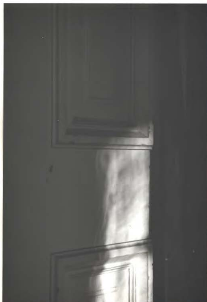
Hall side of door to 1st fl. S.W. room (Italianate details)
