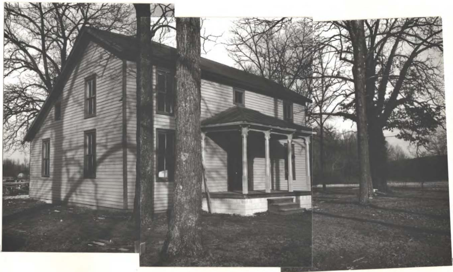
S. front 1982 conc. blk. fndn. ↓ wd steps (hse was raised) Chimneys removed
