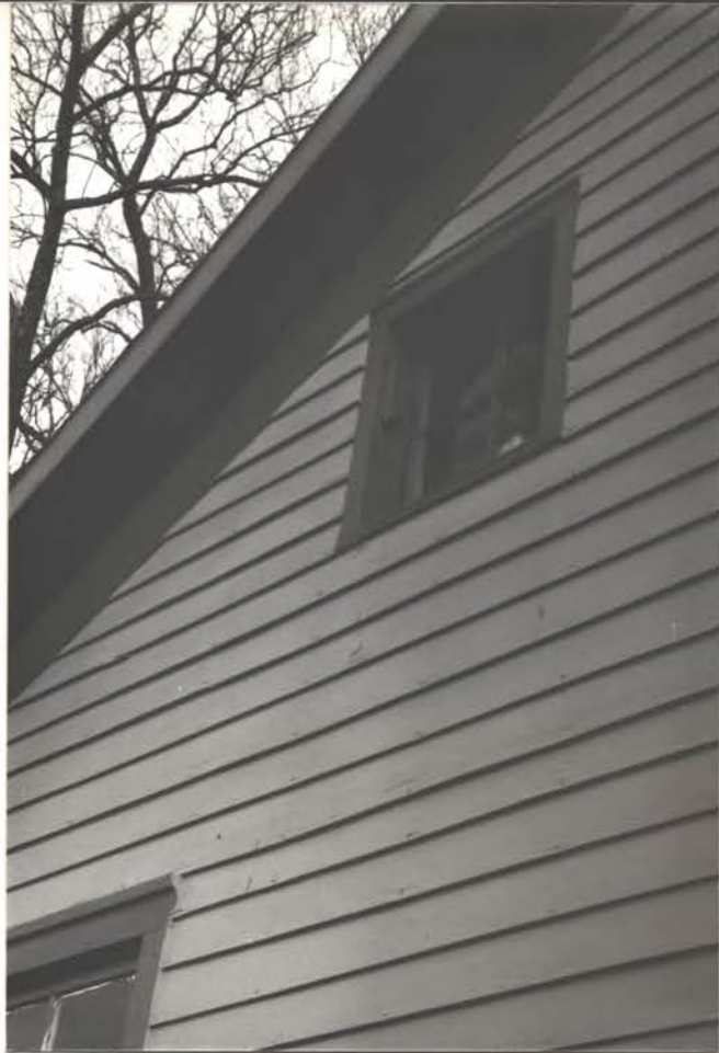
west gable - note pivoting attic sash
