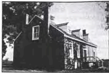
AFTER: Koger House — October 1992
