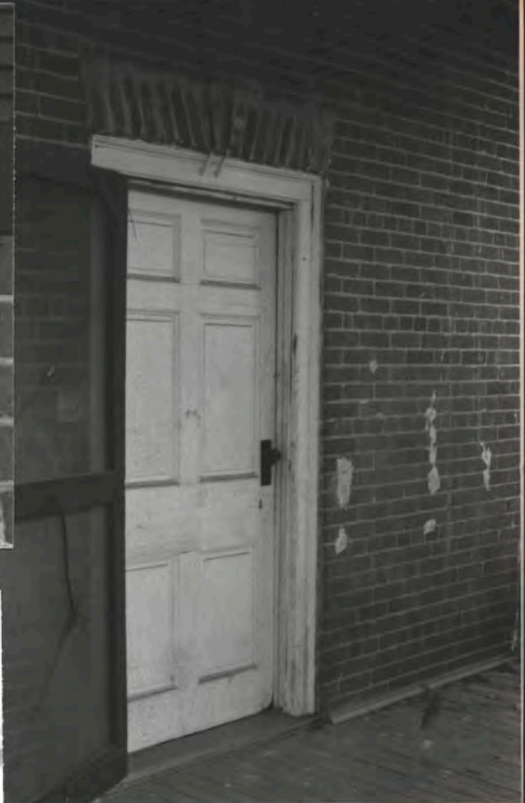
S. Front door - has no glass topl't or sidel'ts. = unusual (dark entry) Lock = 20th c. See orig. keyhole below the lock trace orig. col. ↓
