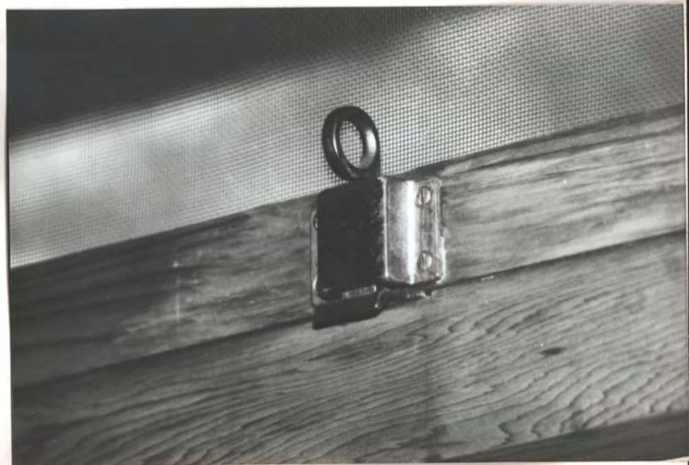
Cleveburn latch (operate w/ hooked rod)
