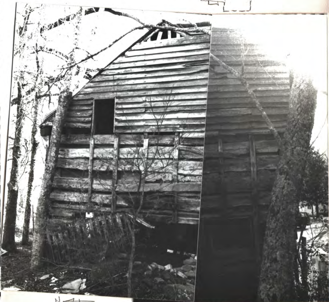
← N WEST WALL
