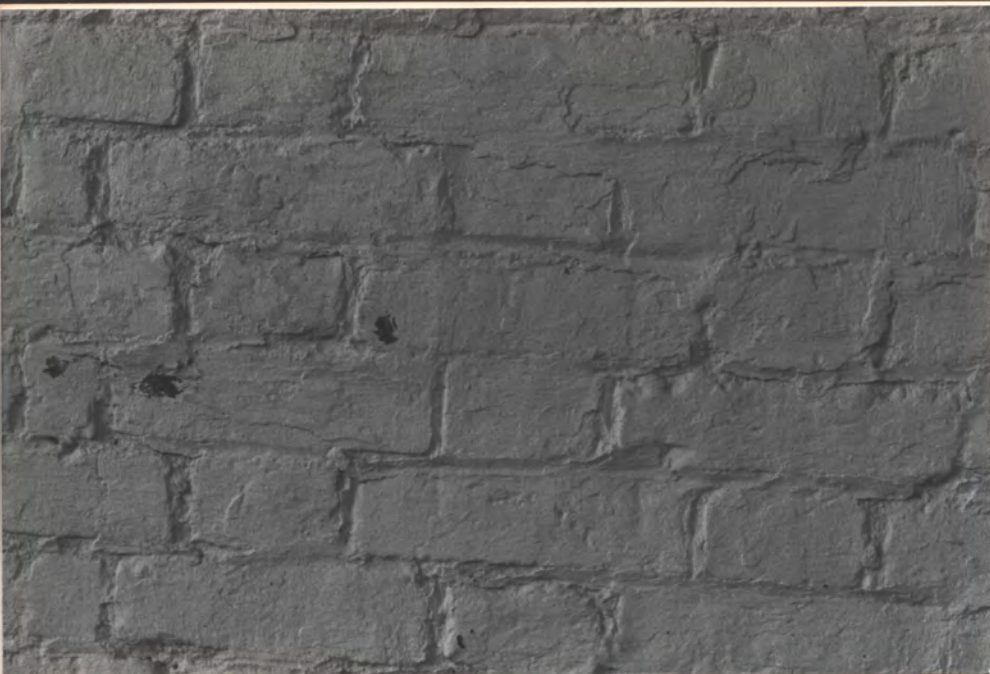
S. Front wall at west side (Flemish bond)
