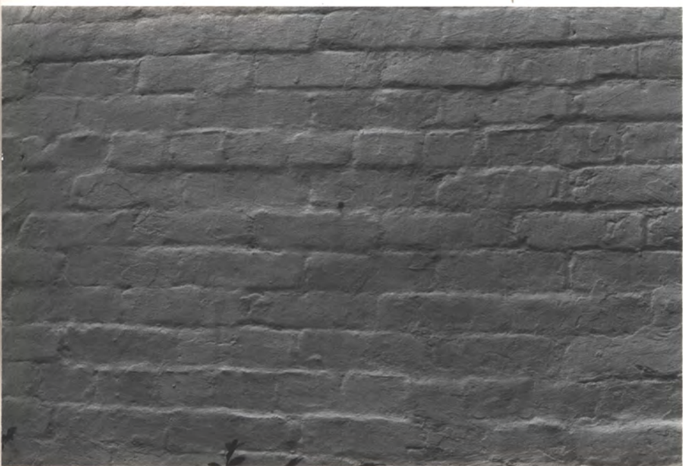
West wall near S.W. front corner Common Bond
