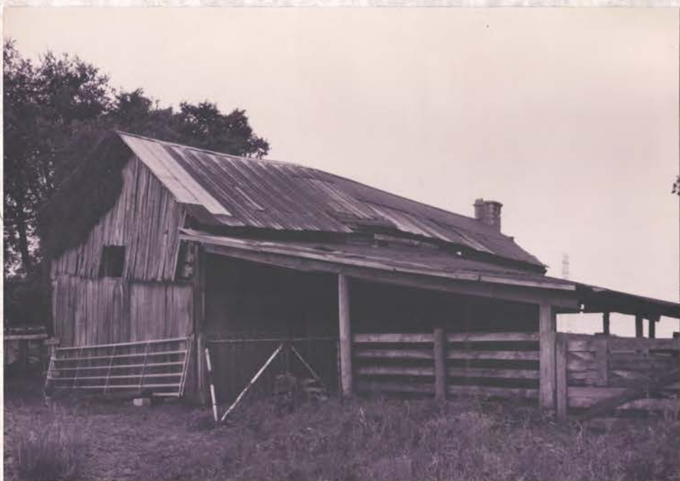
c. 1850's-70's log hse west of Florence, AL (most planks & rafters are rotary sawn) photos June 1997 H.P. Jones
