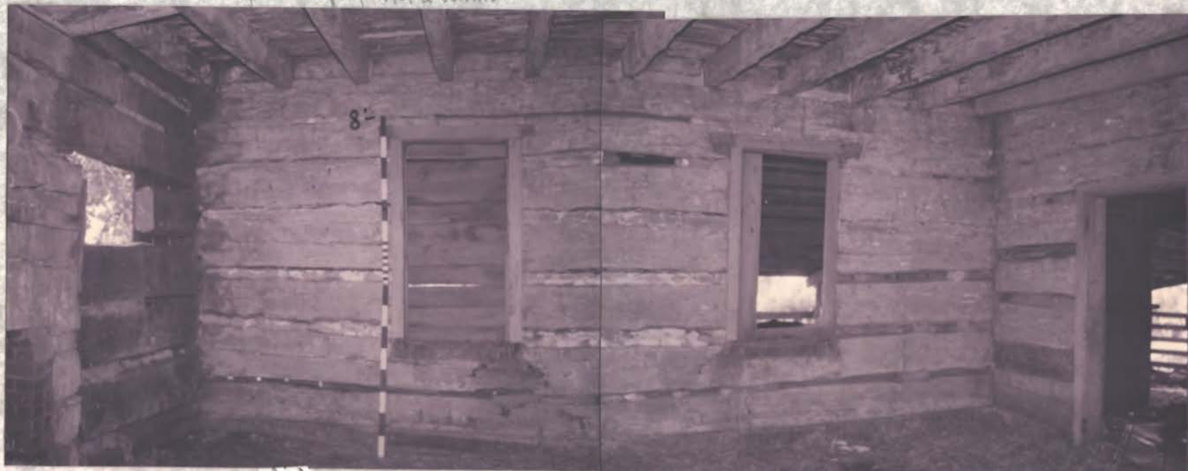
← EAST WALL later brick f. p. lining ↑ later make shift opng. - not a window EAST PEN, Fl. 1
