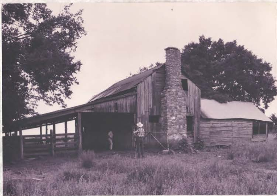
c. 1850's-70's log hse west of Florence, AL (most planks & rafters are rotary sawn) photos June 1997 H.P. Jones
