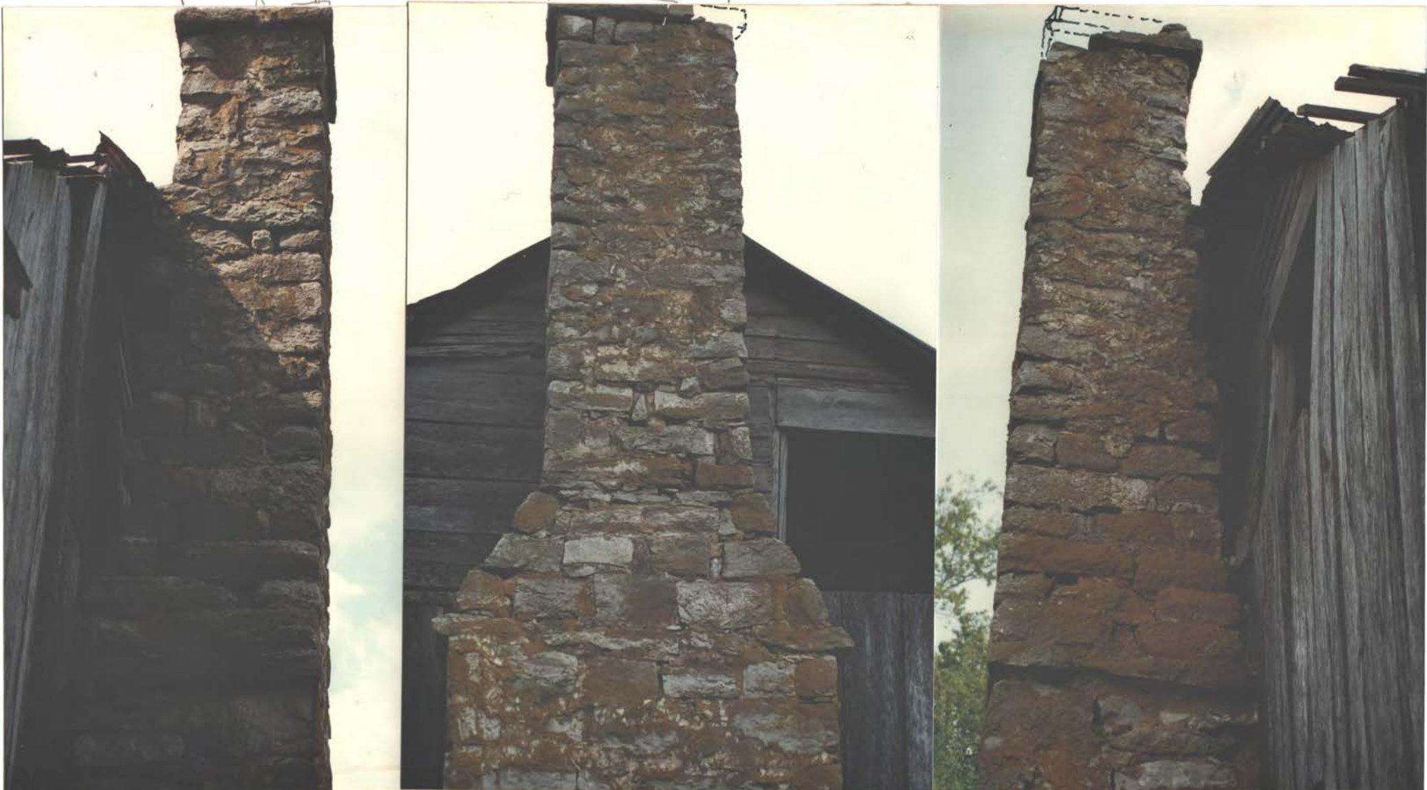
FRONT (EAST BT NEW SITE)
