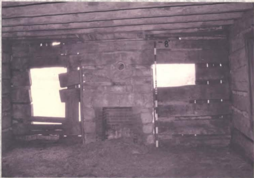
← EAST WALL later brick f. p. lining ↑ later make shift opng. - not a window EAST PEN, Fl. 1
