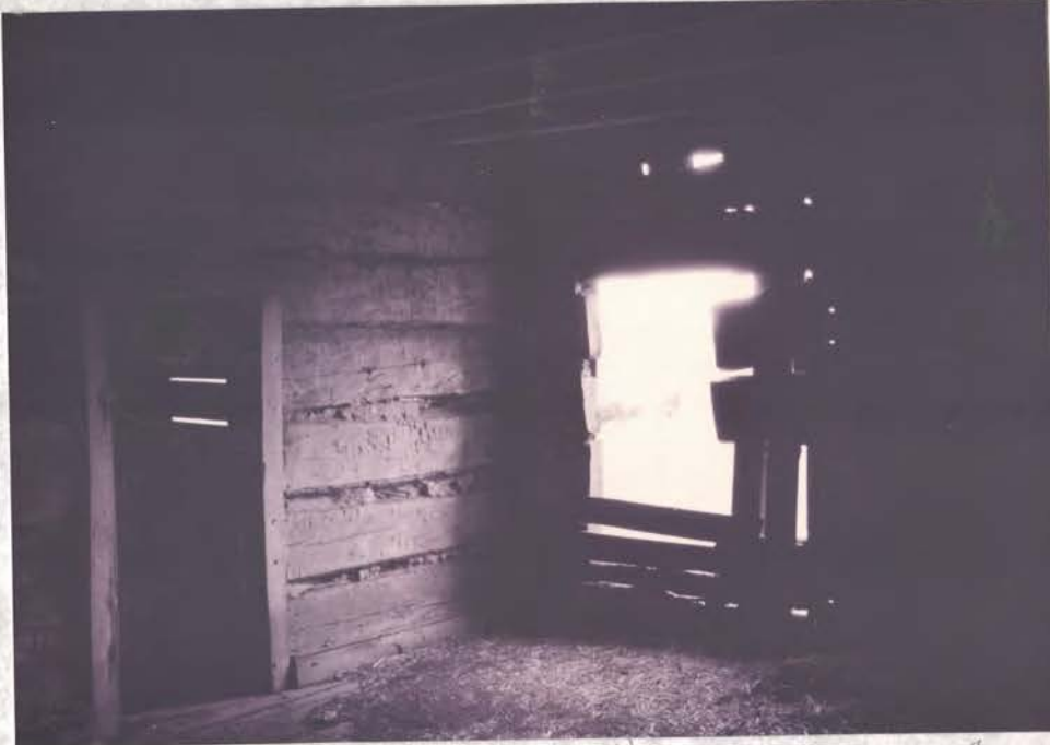
to mod. N.E. wing ← EAST PEN clay daubing → chimney (no mantel)
