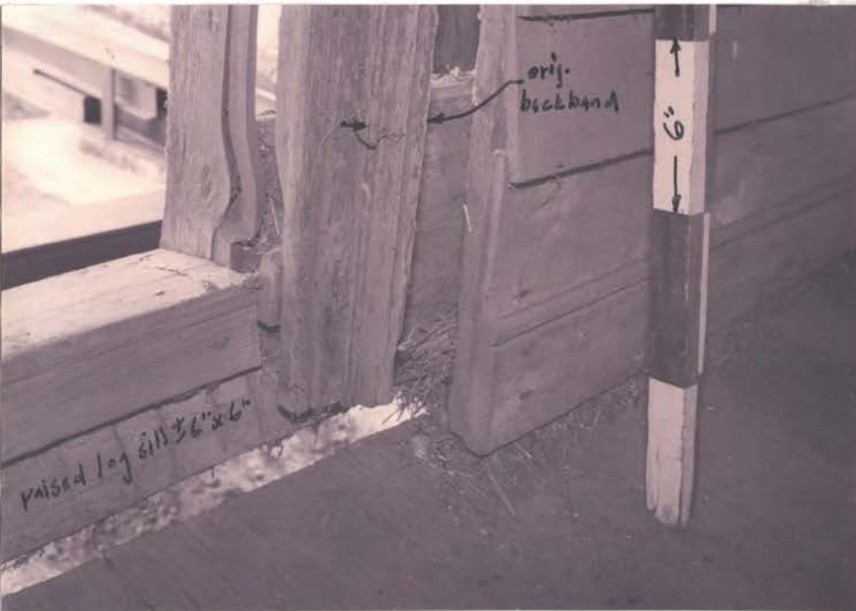
raised 6x6 log sill door frame
