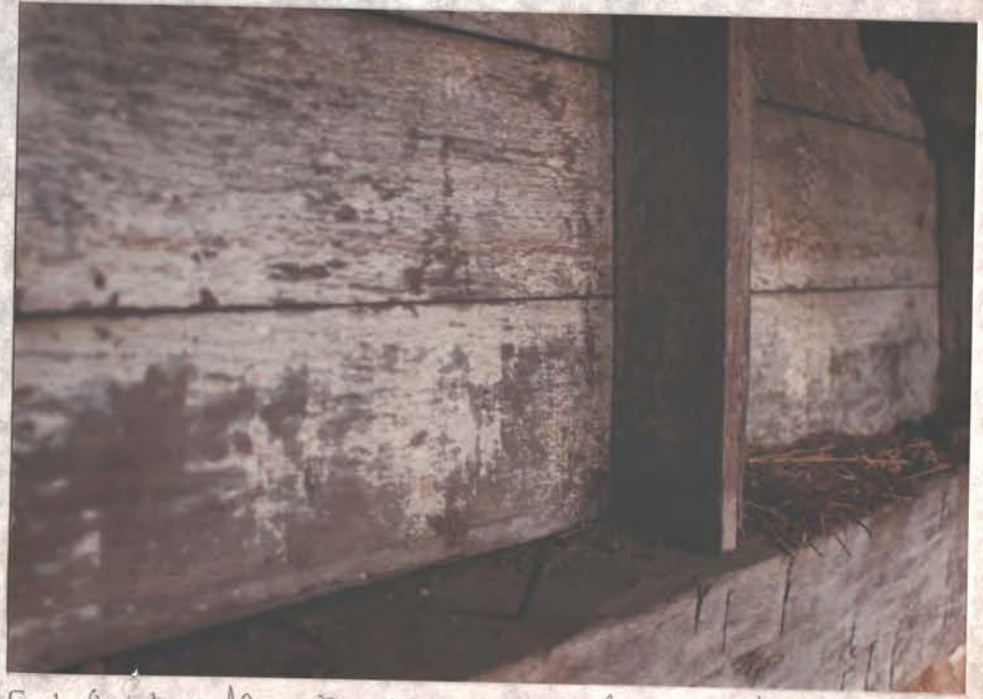
↑ ↑ ↑ ↑ E. Loft, W. wall, note rotary saw marks on stud
