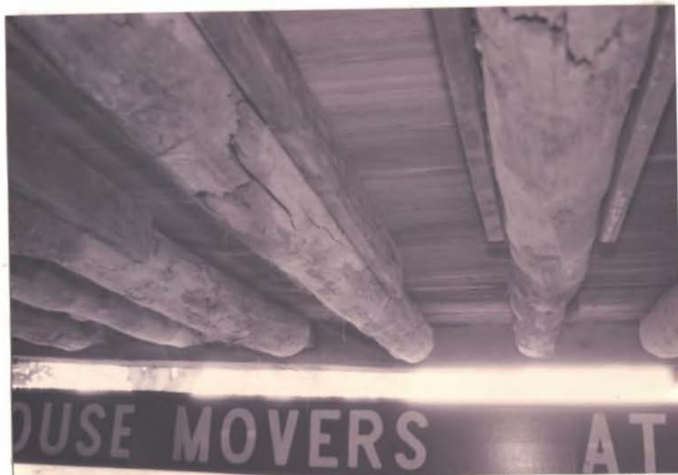
EAST WST, puncheon joists
