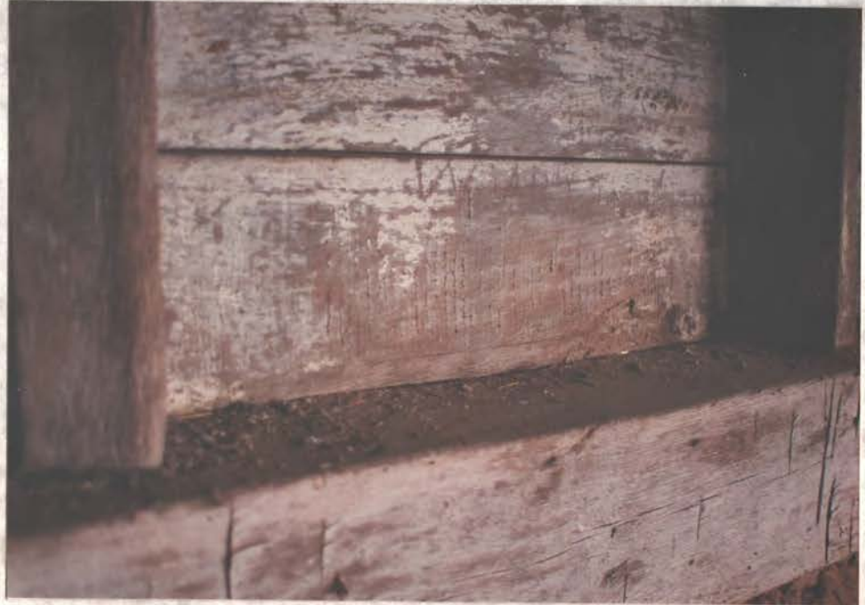
E. Loft, W. wall, note saw - saw marks
