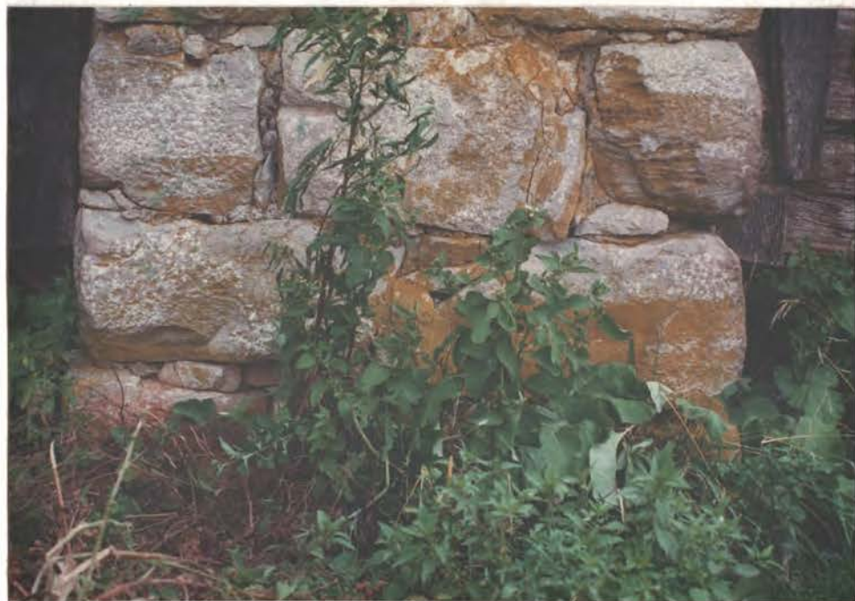
SIDE, BOTTOM (NORTH AT NEW SITE)
