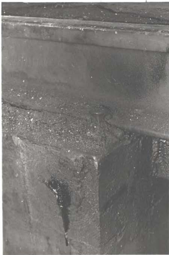
↑ Cross tie embedded in concrete
