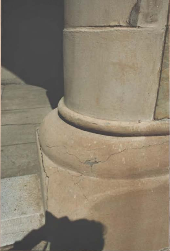
→ Main (west) entry Coating on stone deteriorated 1
