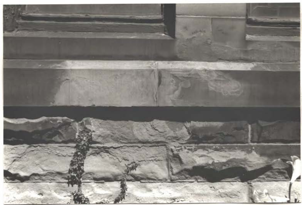
Spalled & patched stone South wall of Sanct. Portland cement re-point
