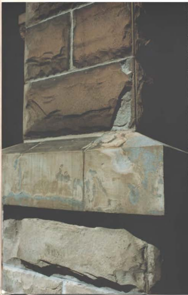
→ Main (west) entry Coating on stone deteriorated 1
