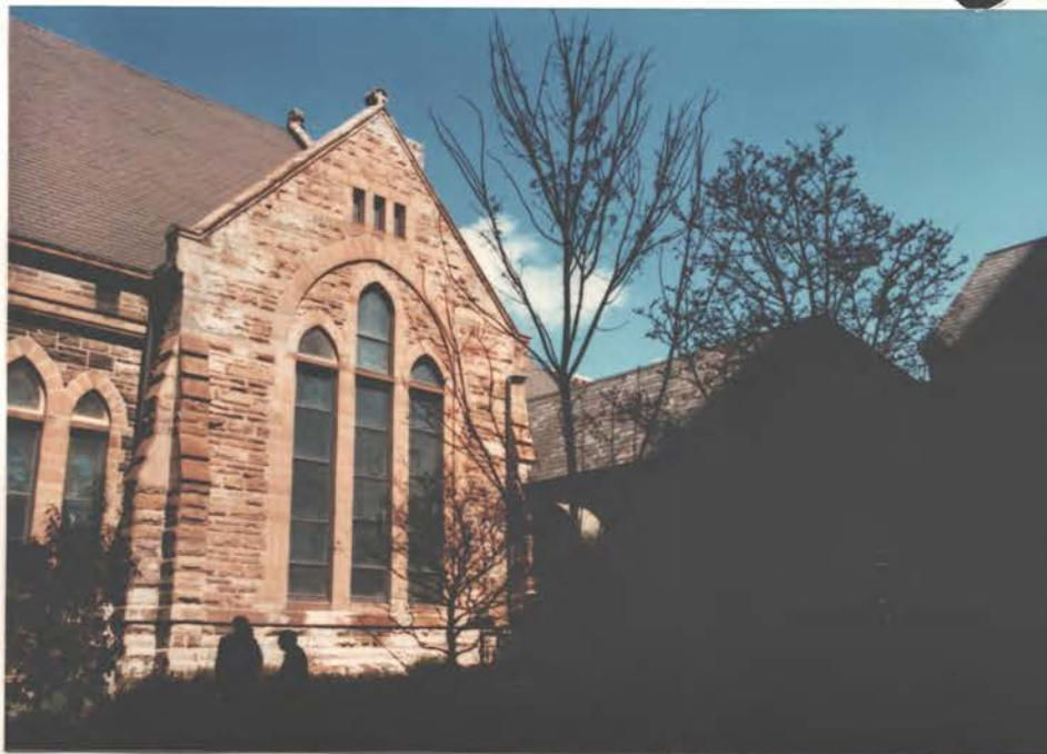
S. Wall at Garden 4 N+ 3
