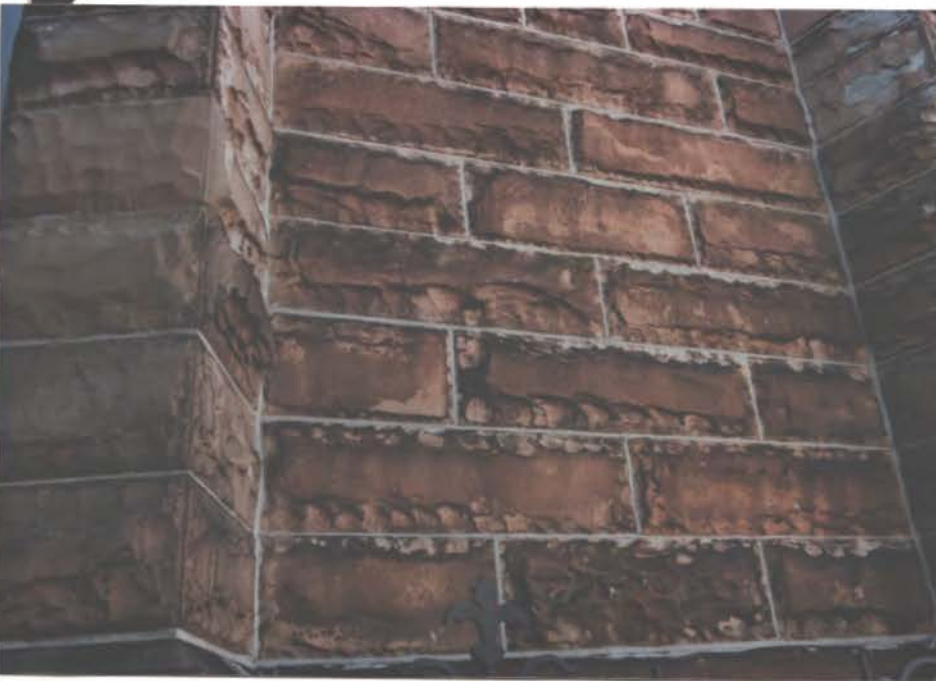
3 Portland cement re-pointing
