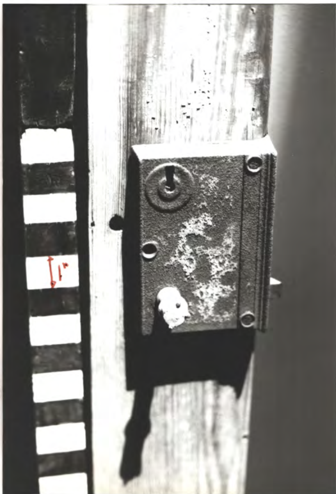
Stevens, Al. "Little Brick" Door Lock (typical of 1850's detailing) 1850's Knobs gone. Found in debris of bldg.
