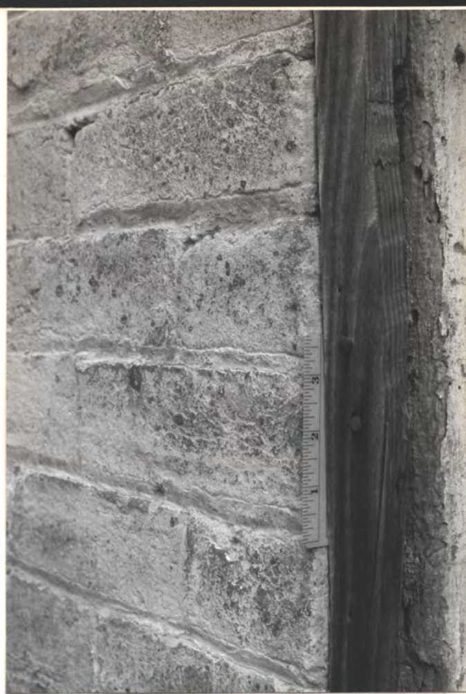
TYPICAL BRICK & MORTAR JOINTING, S. WALL
