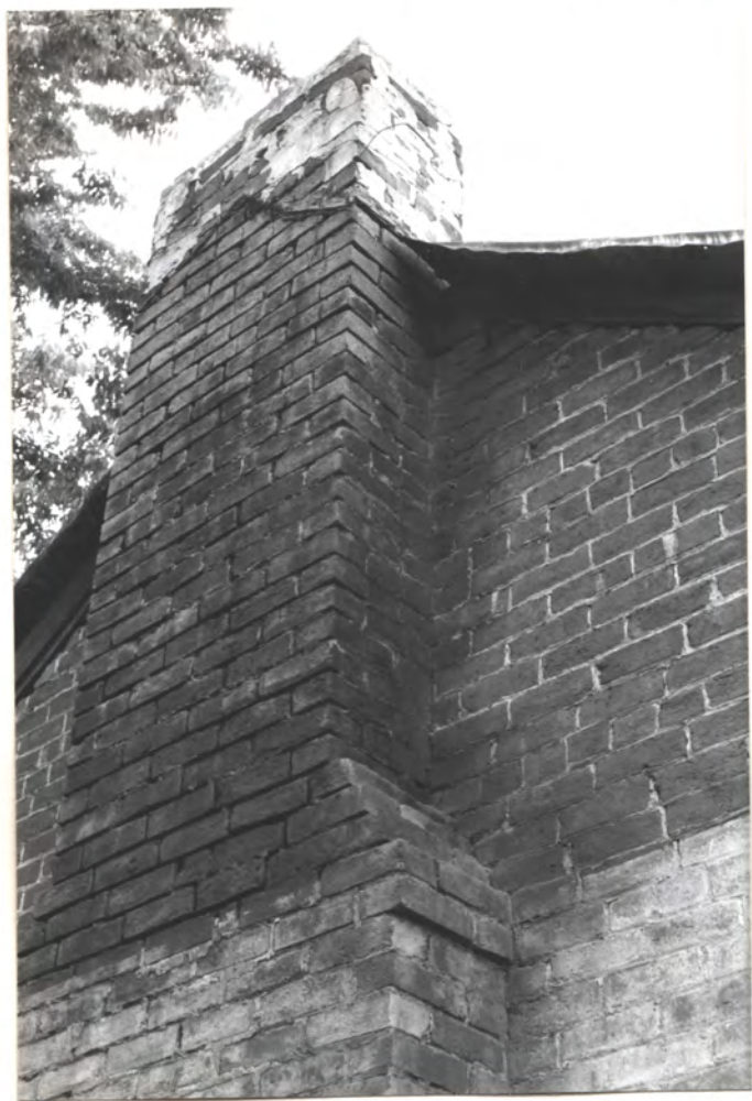
S. CHIMNEY (cap bobbed)
