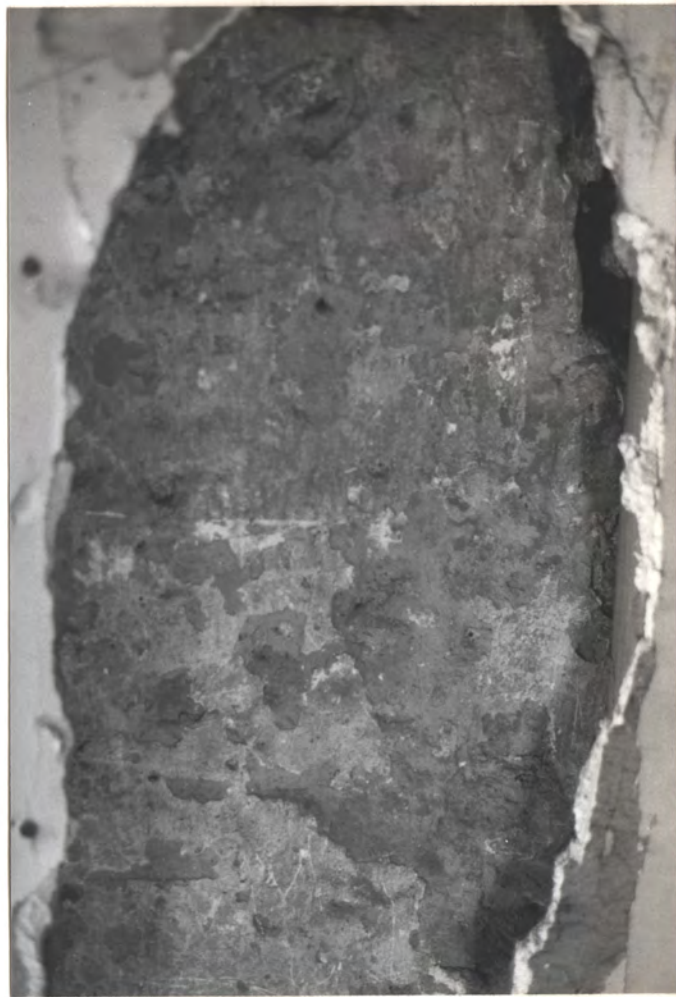
ROUGH BUT PAINTED PLASTER BEHIND WALL BD., BY E. DOOR (GREENISH PAINT ON BROWN COAT PLASTER, NO WHITE COAT)
