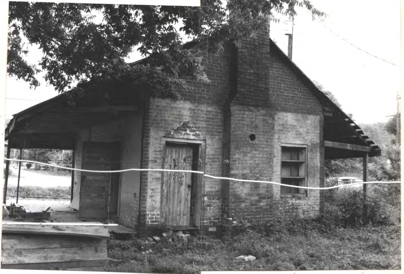
SOUTH WALL (sheds added, chimney bobbed)
