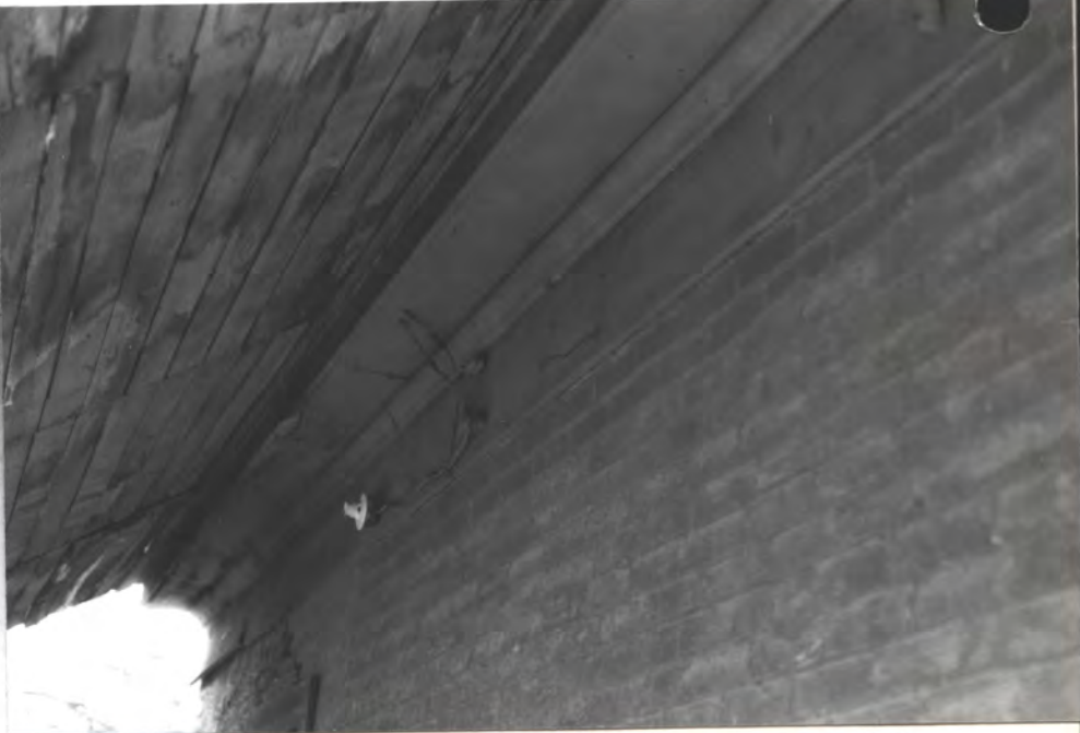
EAST WALL, ORIGINAL CORNICE + ADDED SHED-ROOF SOFFIT
