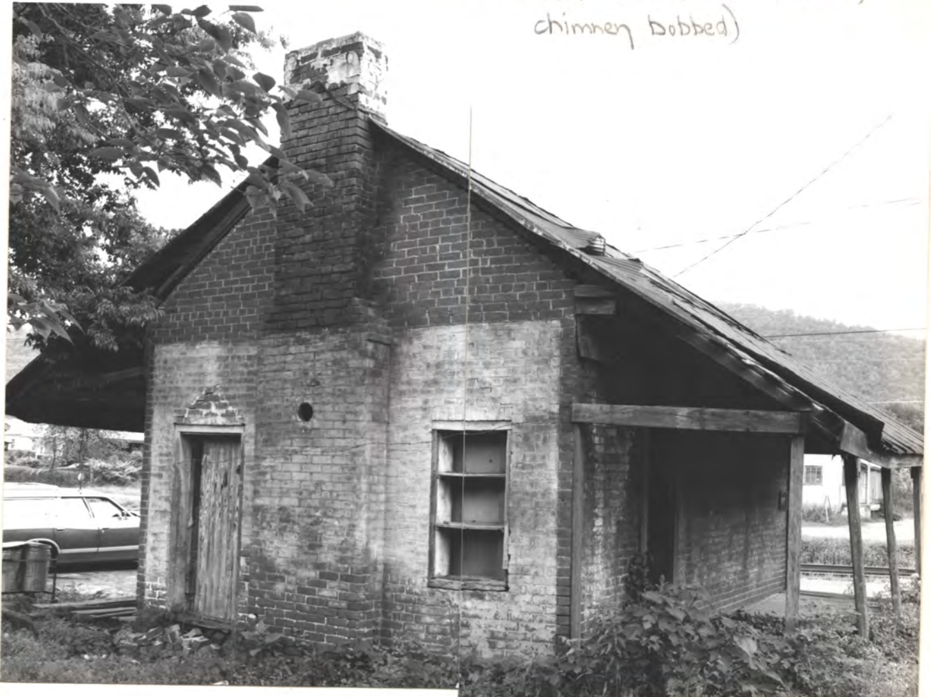
note roof "kicked up" for sheds
