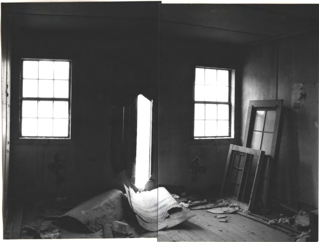
LOOKING N. TO ST. + R.R. TRACKS (FRONT)
