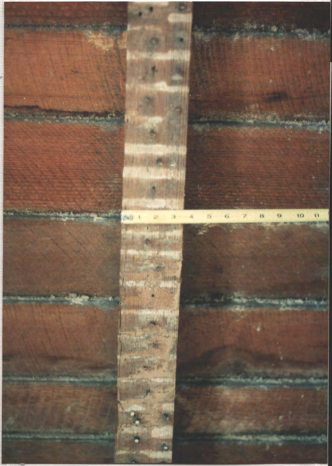
↑ TYPICAL STUD 1 2 3 4 5 6 7 8 9 10 11 * 13 1/2" * Note Rotary Sawn Clapbd indicates c. 1860 or later
