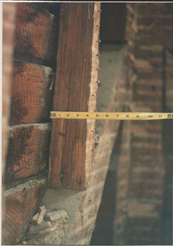
↑ TYPICAL STUD 1 2 3 4 5 6 7 8 9 10 11 * 13 1/2" * Note Rotary Sawn Clapbd indicates c. 1860 or later
