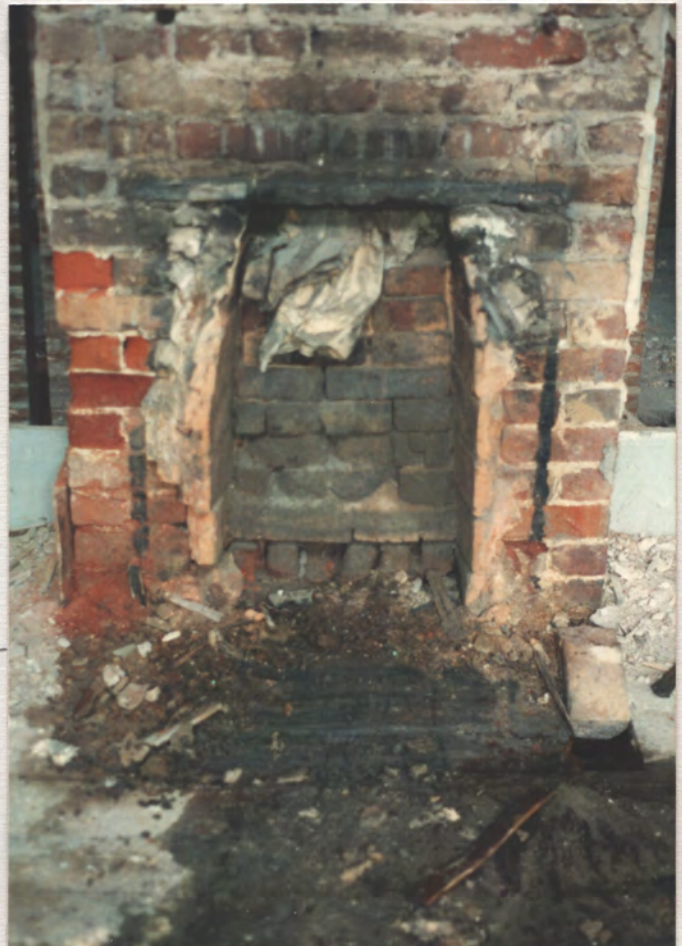
N.W. Rm F.P. — Lined w/ firebrick for small coal grate. Lining appears later. 566 p. 8
