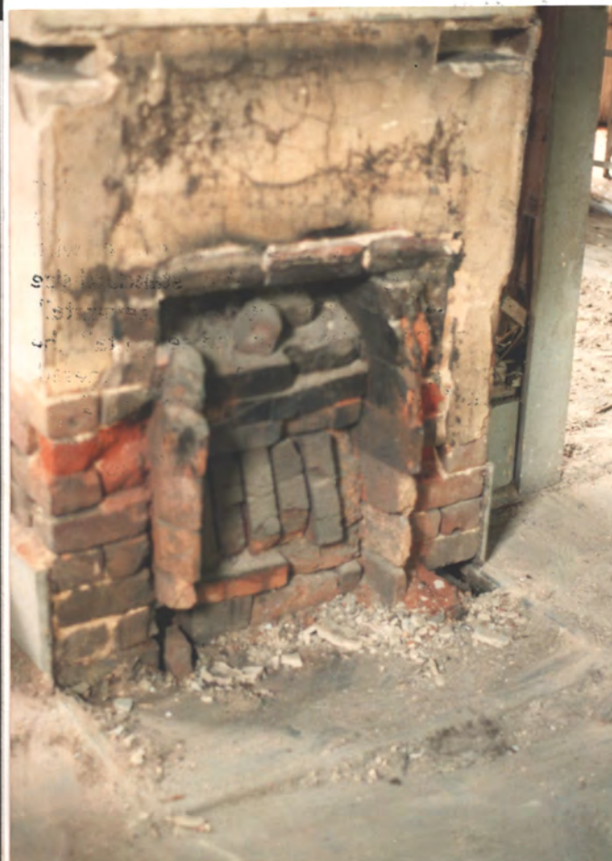
Front (S.E.) f.p. → N w) later coal grate lining (note worn edges of horiz. bricks)
