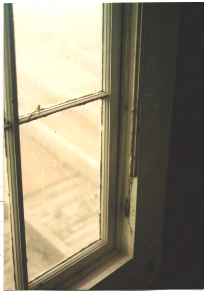
Front (east) sashes
