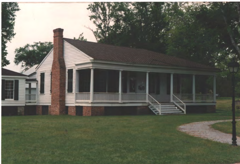
1991 photo - HJ - c. 1840 Iredell Vaughan 1751 Eutaw - JH Arch, AL
