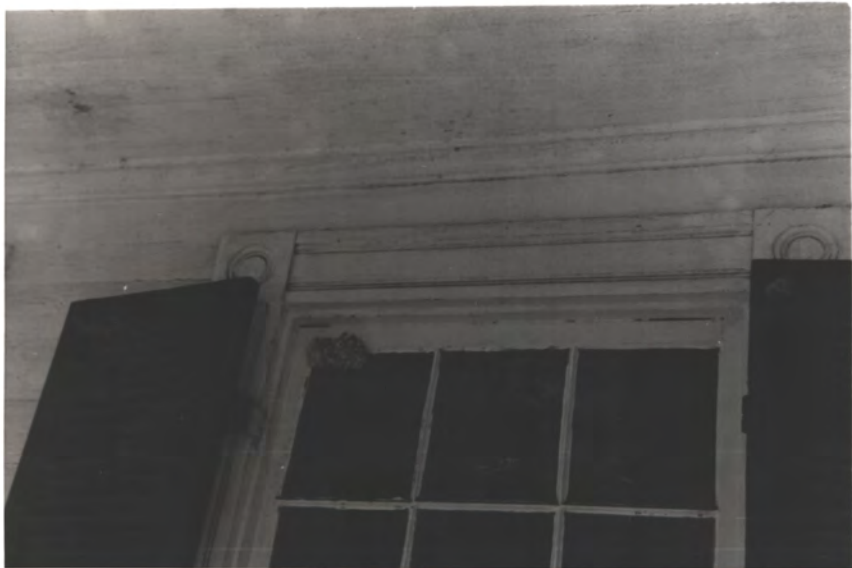
South of S.E. porch
