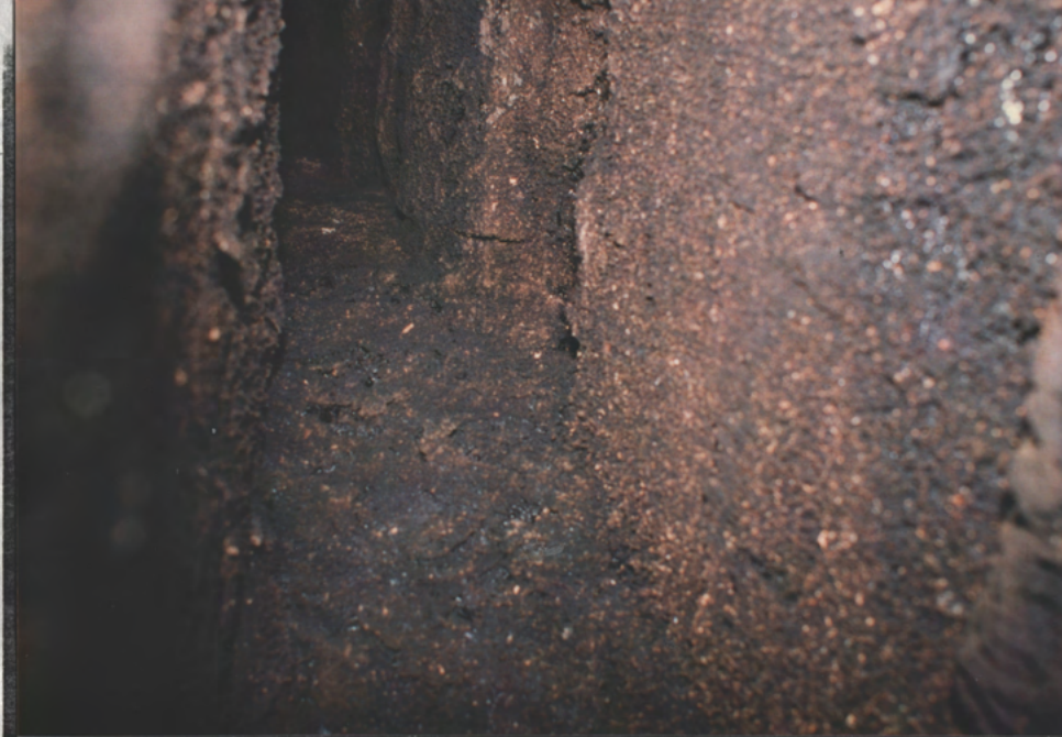
Cabin 7 - stone - flash, heavily coated w/ rosin = dangerous. Up to 3/4" thick.
