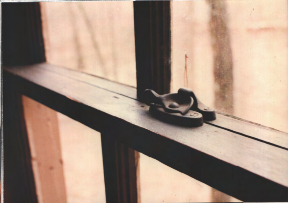
Narrow 4/4 sash w/ thick vert. center muntin (Vic. style, but appears 1930's-?) Moulded sash lock
