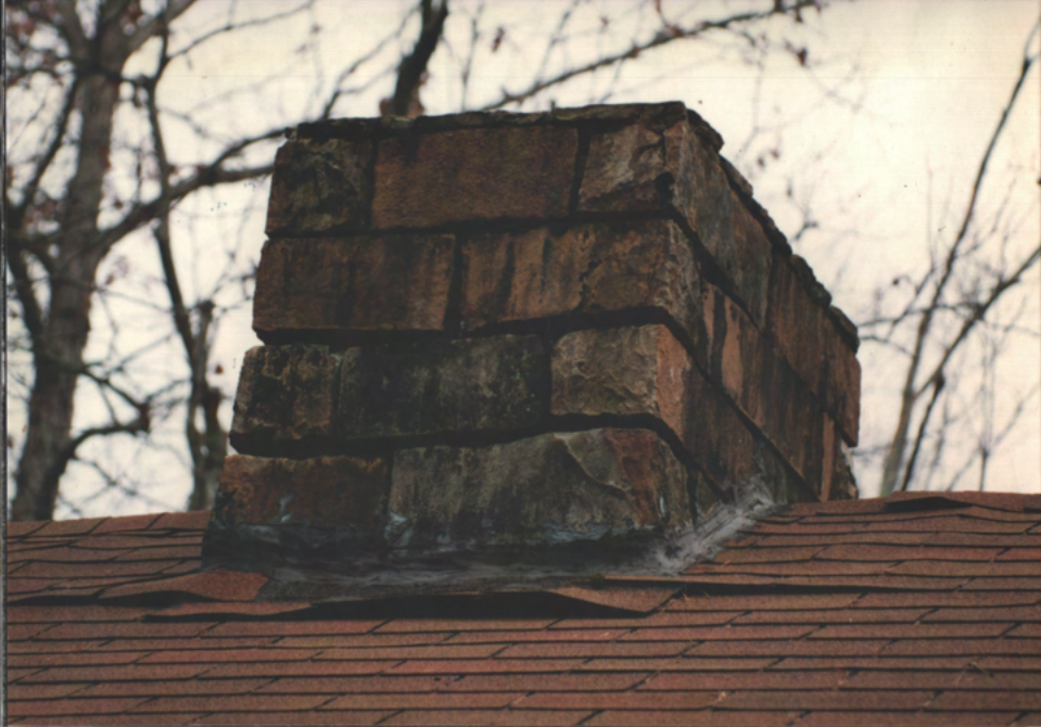
Cabin 11 - TYPICAL - g.W. flash, tucked into stone + black roofing cem, smeared Flash is buckled - up
