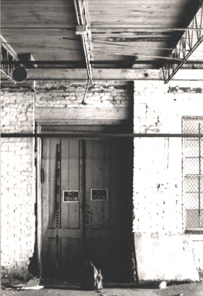
Later doors at W. wall of 1889 Bldg. onto Mod. loading dock This was a window in the 1889 photo. See front sect. of this book Doors originally were at the N.W. corner. These may be originals, moved south 2 or 3 bays
