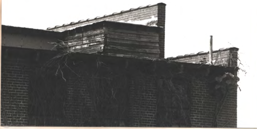
N. Parapet at Boarding Rm → N
