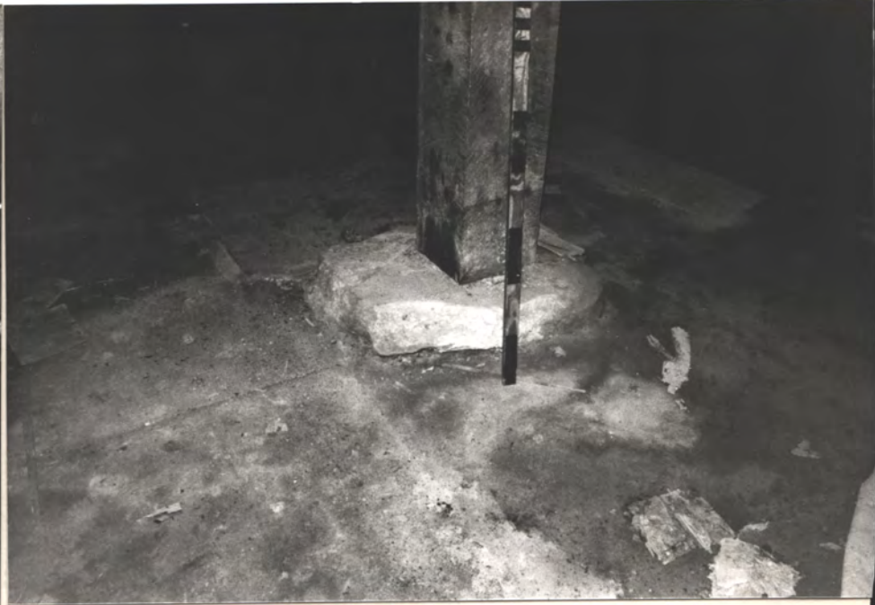
Col. base (stone footing) → N
