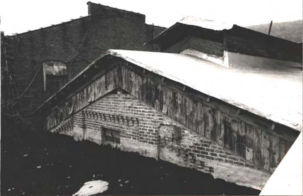
Later doors at W. wall of 1889 Bldg. onto Mod. loading dock This was a window in the 1889 photo. See front sect. of this book Doors originally were at the N.W. corner. These may be originals, moved south 2 or 3 bays
