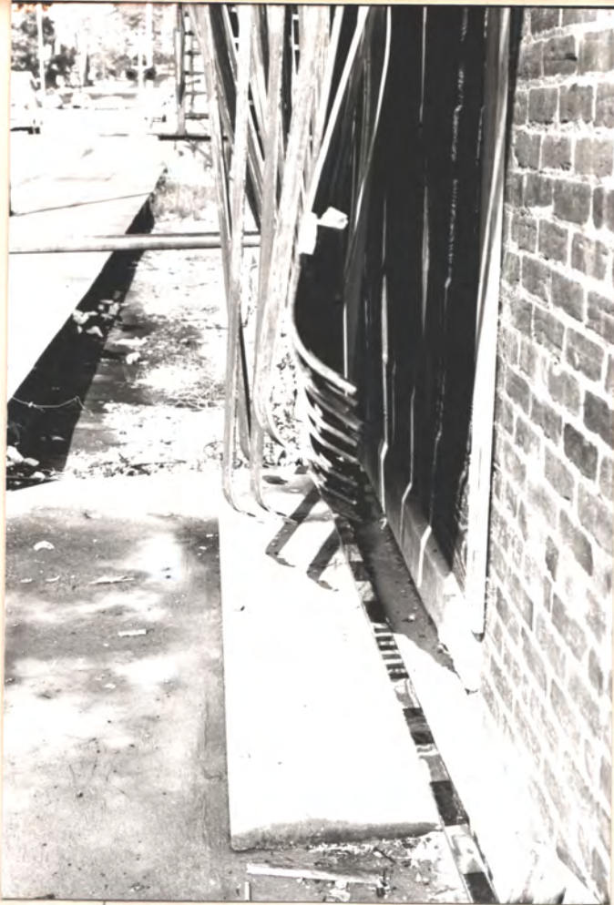
S.E. entry to 1889 Bldg (collapsed metal awning at front)
