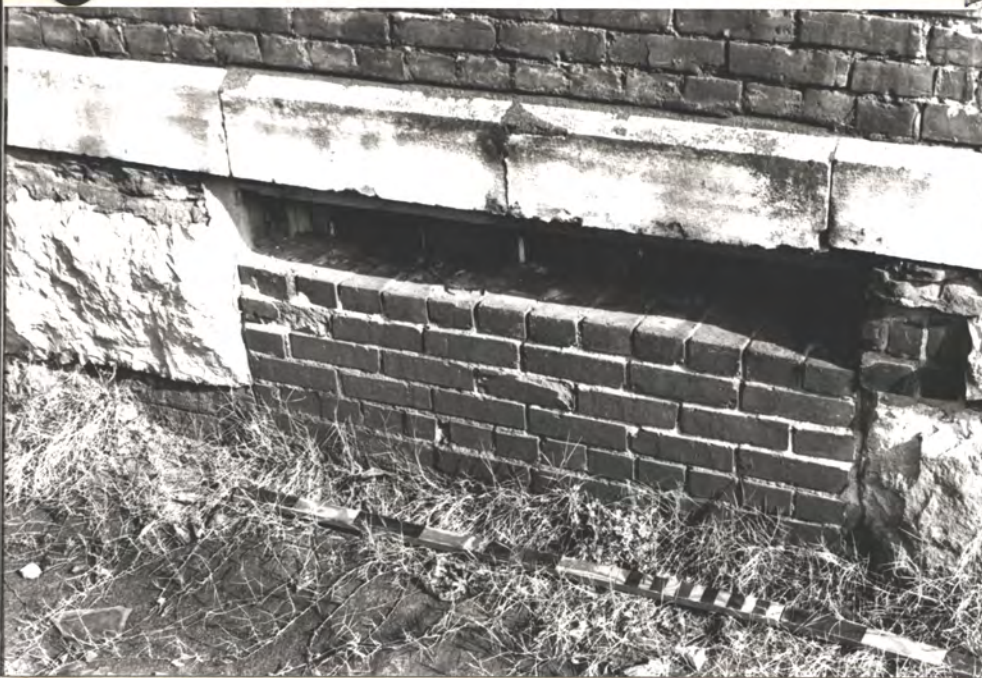
Basement wind. (not in 1889 photos, later bricked - mg)
