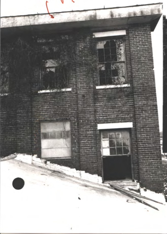
Later doors at W. wall of 1889 Bldg. onto Mod. loading dock This was a window in the 1889 photo. See front sect. of this book Doors originally were at the N.W. corner. These may be originals, moved south 2 or 3 bays
