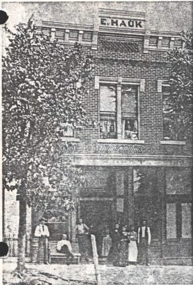
Cullman Ice Factory — E. Hauk came to Cullman in 1884 and operated a meat market until 1895 when he installed an ice factory on the first floor of this building on First Avenue East. Mrs. A. Dinckelburg bought the first ice on June 6, 1895.
