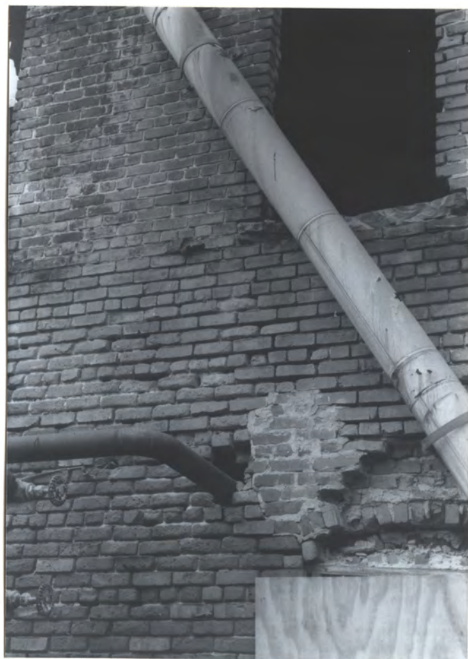
East rear, 2nd fl. window opening
