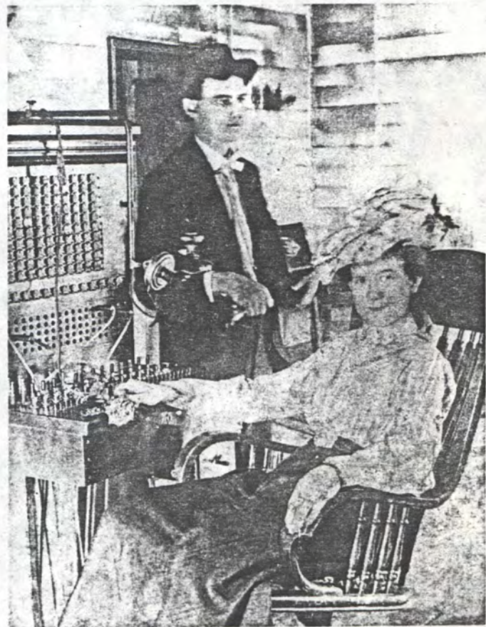
Telephone Operator — Miss Susie Graves (Mrs. Will Clark) sits at the switchboard of the Cullman Telephone Company office, as the manager, Mr. Simpson, looks on.
