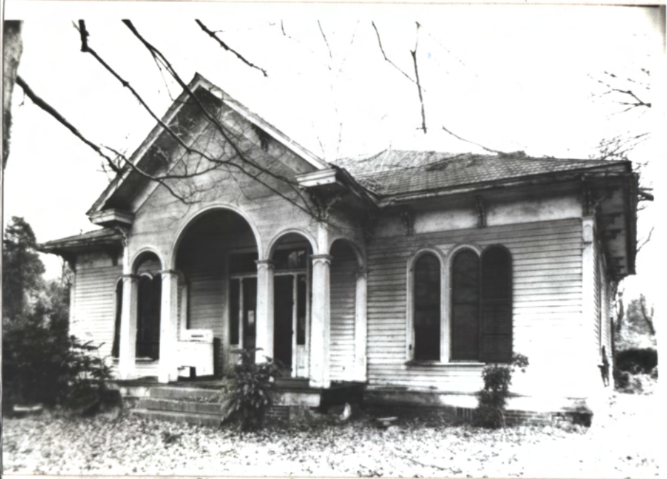
← 1978 H.K.B. photo just before Mandlins restor. Hx empty & vandalized
