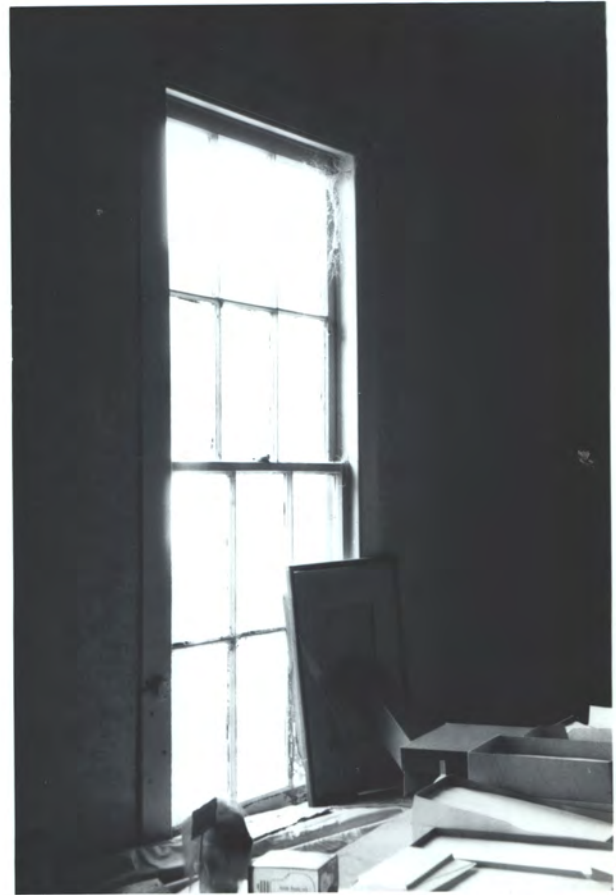
Look at left center rm. (Fed. sink moved from front Fed. rms) This is a later "Infill" room between Fed. front, & serv. bldg.
