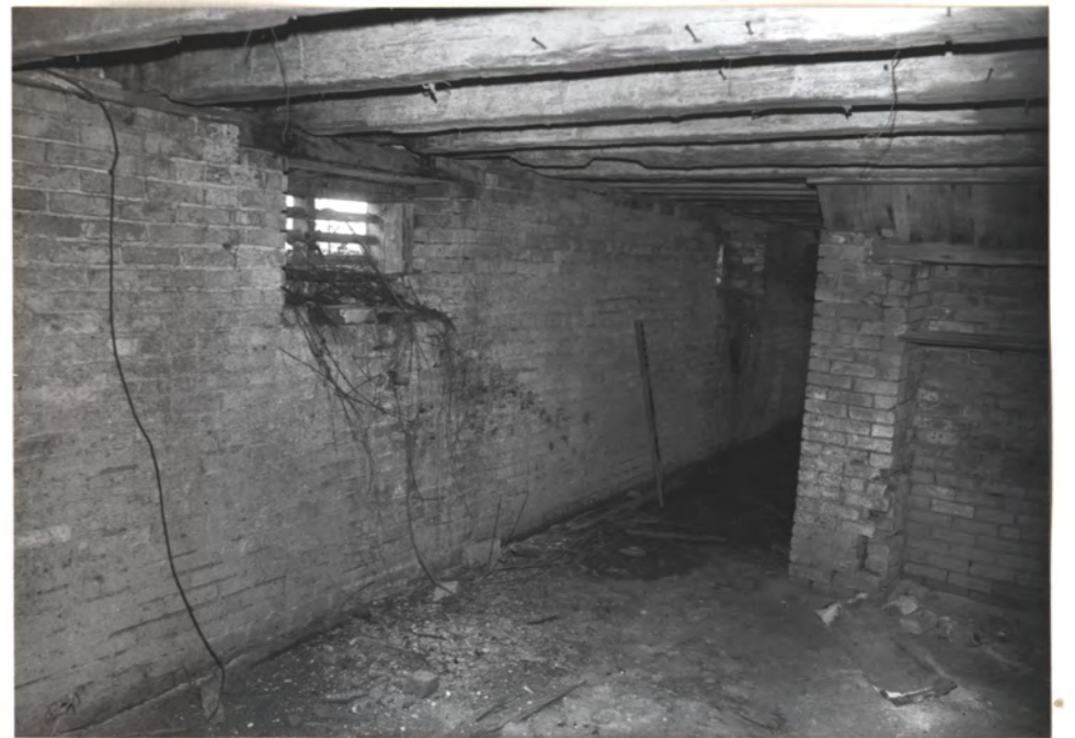
EAST CELLAR- EAST WALL (LOOKING SE.)
