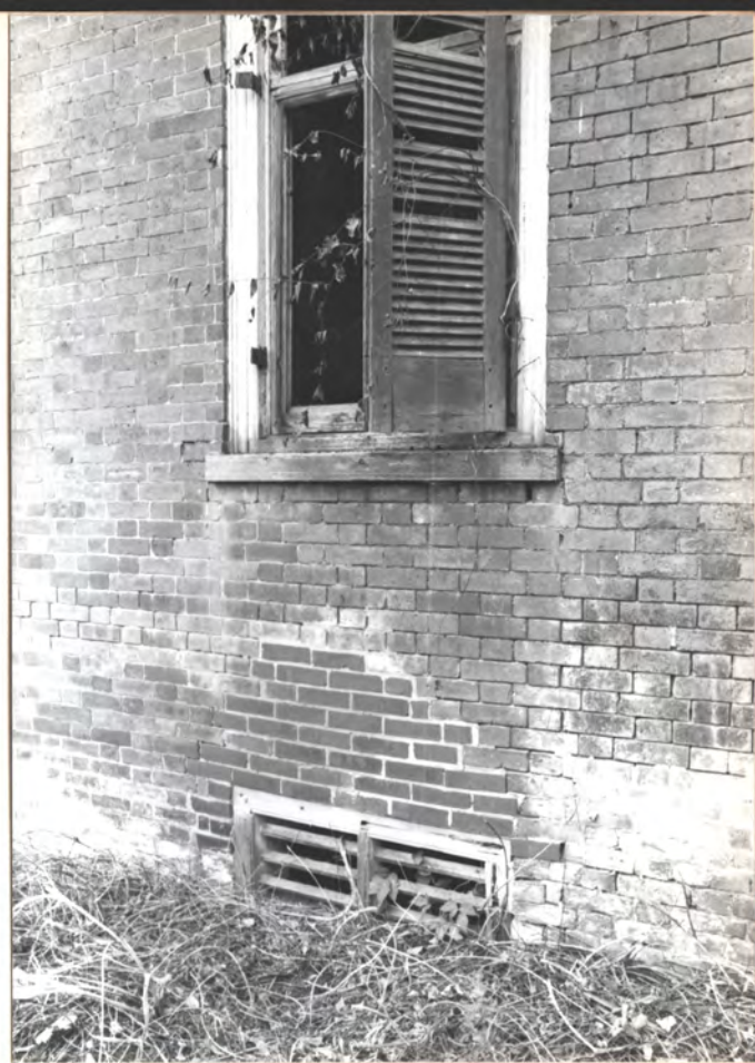
E. Wall, Center Rm. with 20th cent. brick over vent
