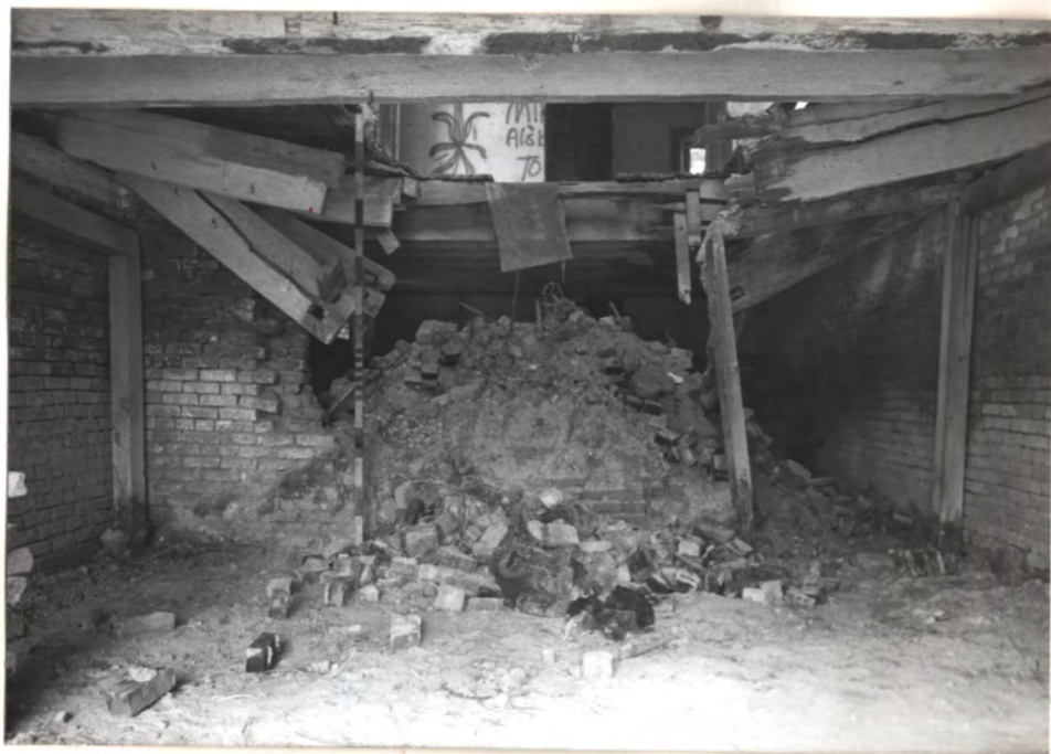
WEST CELLAR - LOOKING NORTH
