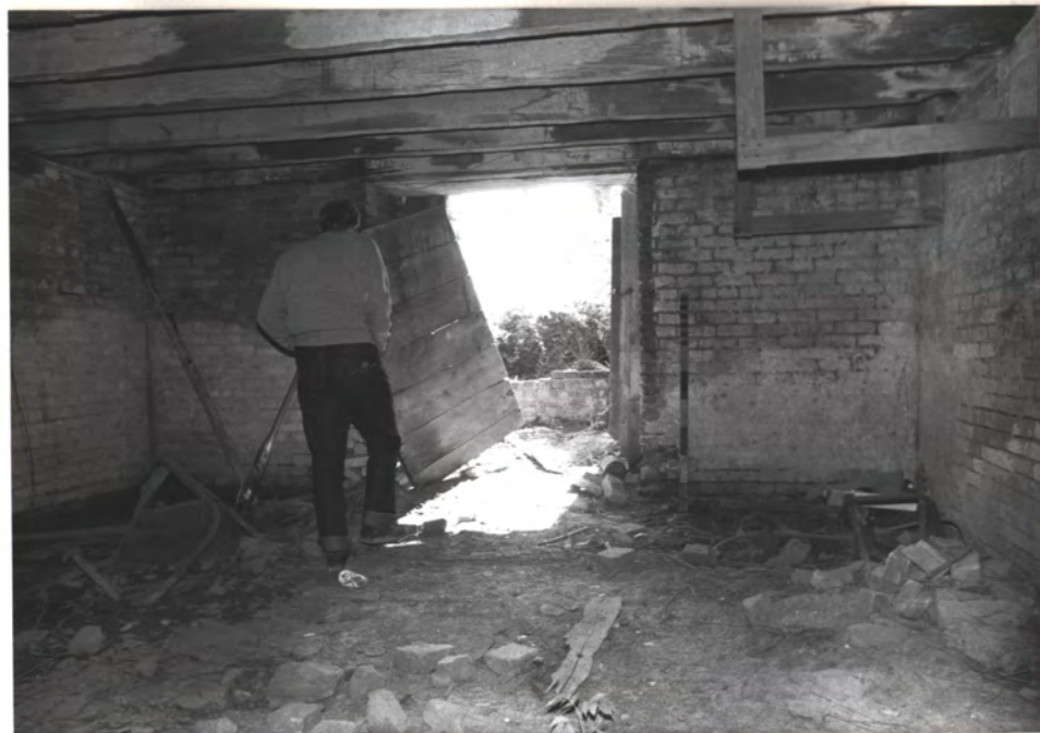
EAST CELLAR SOUTH END
