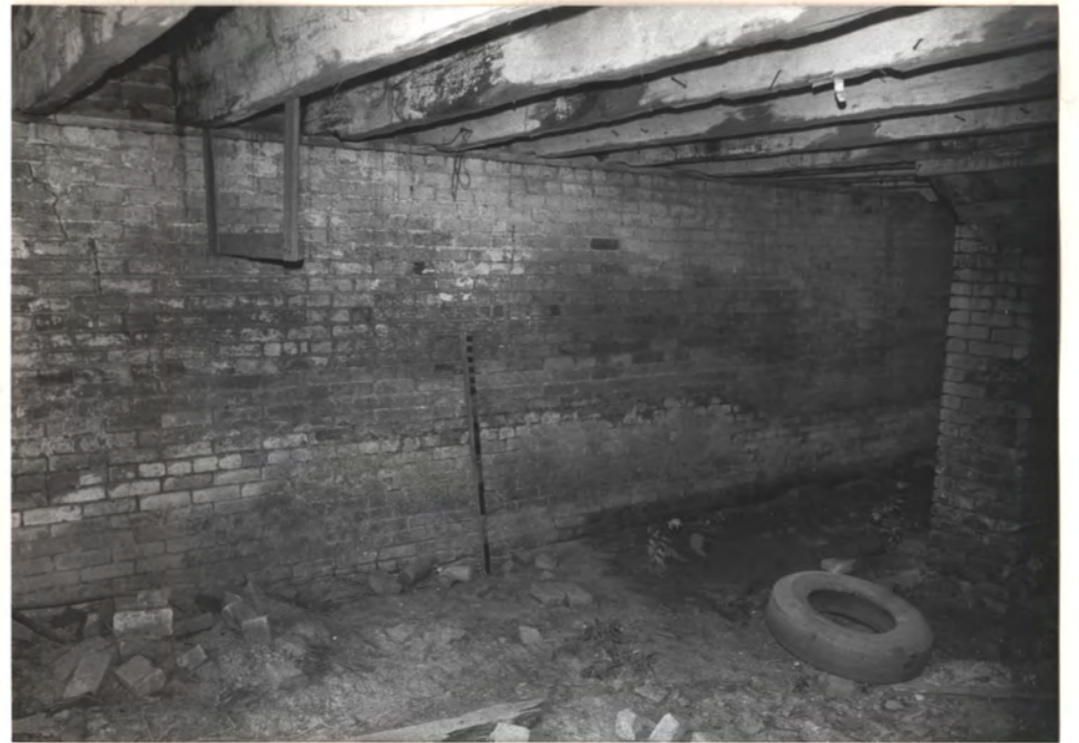
EAST CELLAR- WEST WALL
