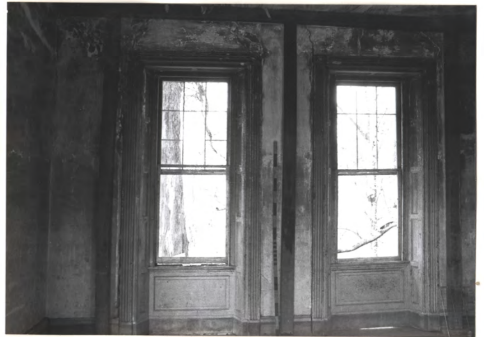
WEST WALL S.W. CORNER ROOM "BEDROOM 2"
