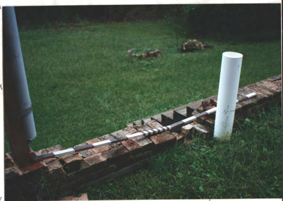
Retain. wall / 1984 PVC drainage stub
