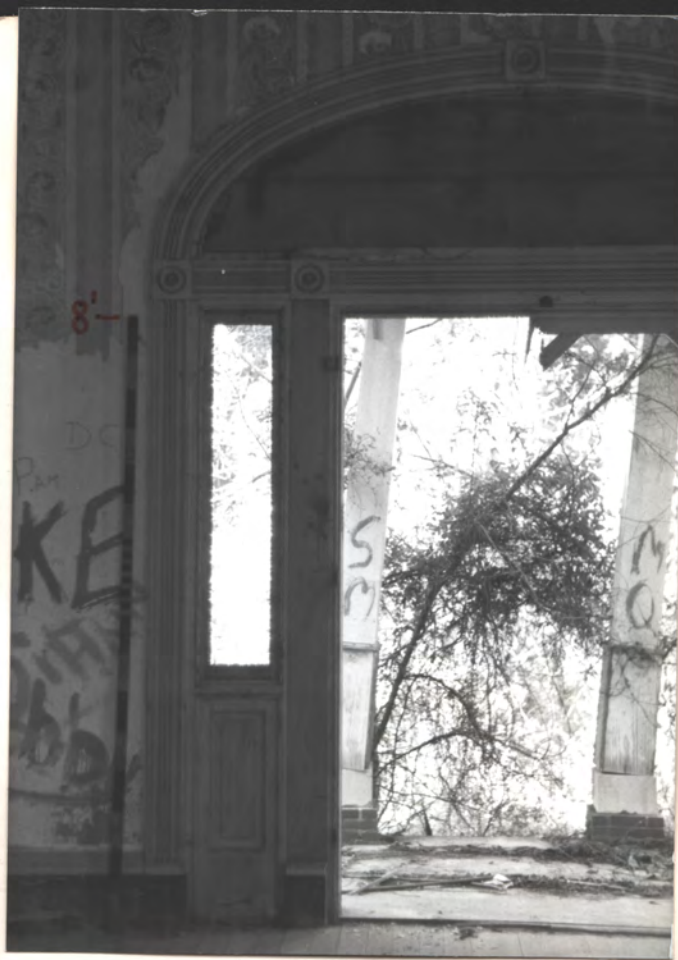
N. ENTRY TO PORTICO (MAIN LEVEL) COLS = SOLID WD., W/ ENTASIS (NOT STRAIGHT TAPER)
