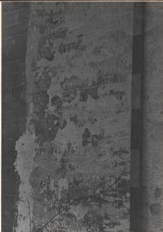
"PENCILLED" FALSE STONE JTS. ON STUCCO AT LOGGIA. STUCCO LOOKS MARBELIZED, REDDISH MOTTLE (UNCERTAIN)
