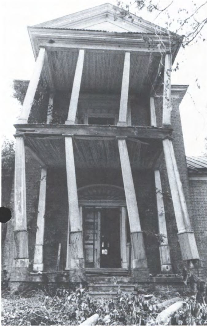
The unrestored portico was missing the second floor cornice as well as the first floor and steps. The HABS drawings and photos enabled a restoration that is at least very close to the original. The mansion now exudes the stately elegance it must have had in 1828. (Photos: Herrin & Jones, Architecture/Interior Design)
