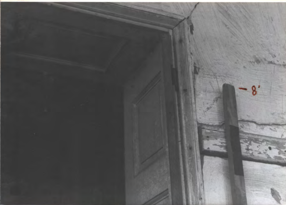
W. WALL DOOR AT LOGGIA. BD. IN STUCCO FOR HANGING ITEMS ON WALL
