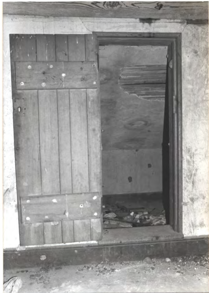
Door to stairs by stairs to partition roof
