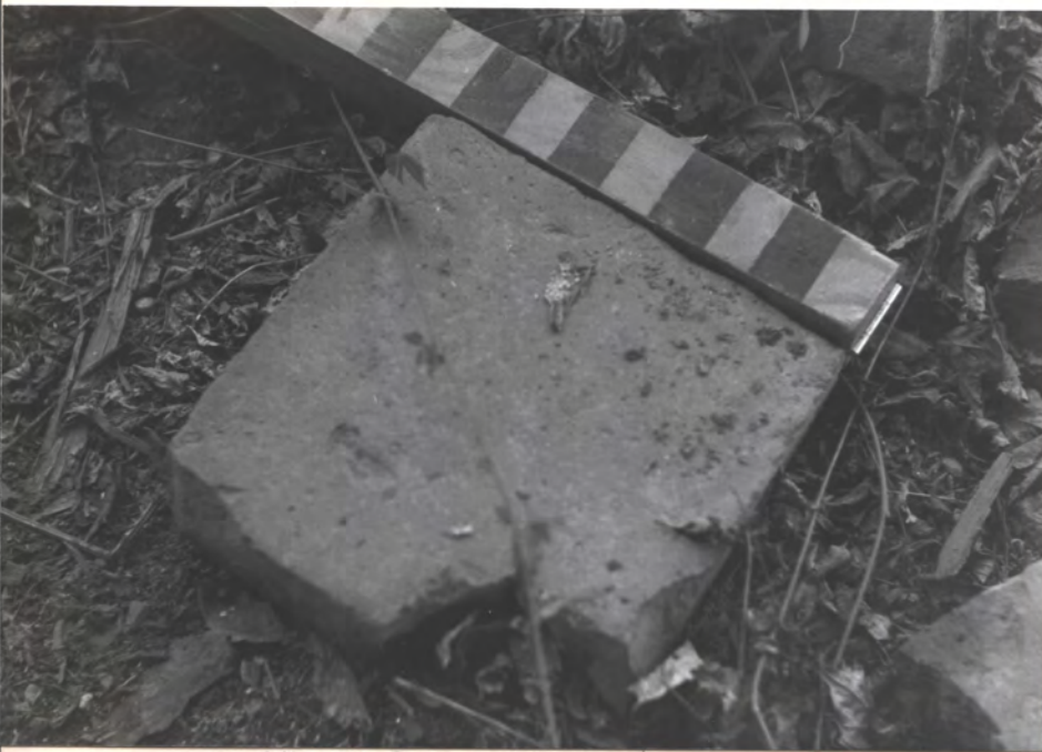
TYPICAL PATIO BRICK (MOST GONE) PATTERN IS 1/2 BOND PER H.A.B.G.
