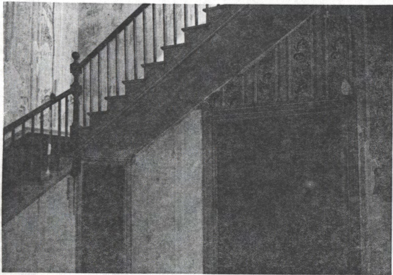
Main stair (c. 1966)
