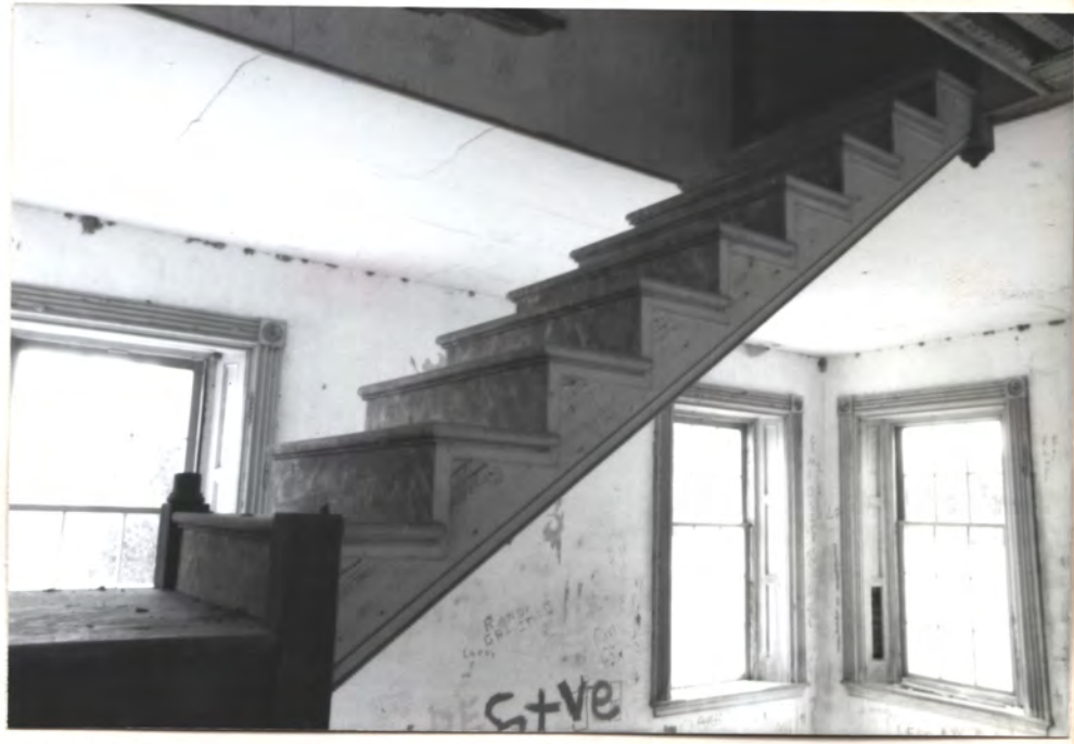
STAIR TO "ATTIC" → N
