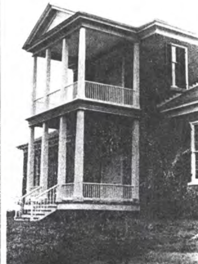
The Belle Mont portico was pulled back from the brink of collapse. Wherever possible, original material was kept — and repaired or patched as necessary.
