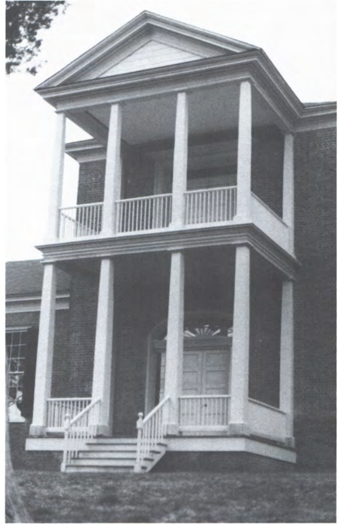
The unrestored portico was missing the second floor cornice as well as the first floor and steps. The HABS drawings and photos enabled a restoration that is at least very close to the original. The mansion now exudes the stately elegance it must have had in 1828. (Photos: Herrin & Jones, Architecture/Interior Design)
