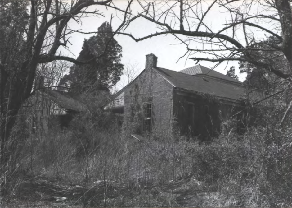
S. (REAR) WALLS FROM S.E. OF HSE.
