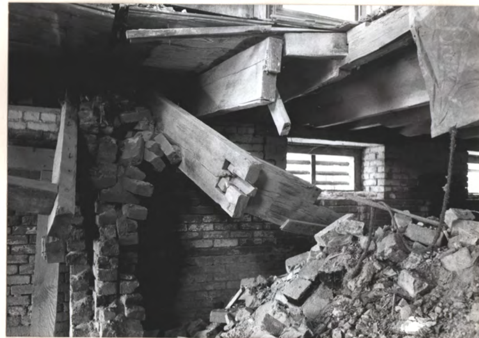
LOOKING WEST IN CENTER OF WEST CELLAR
