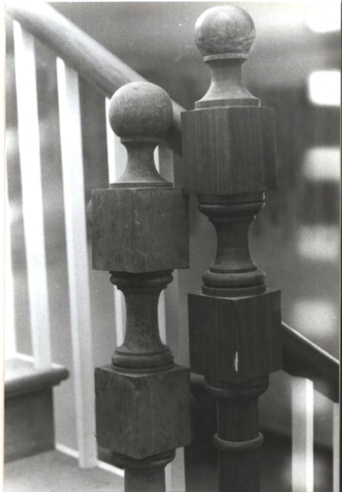
ORIG. REPRO. MAIN STAIR MID-LANDING
