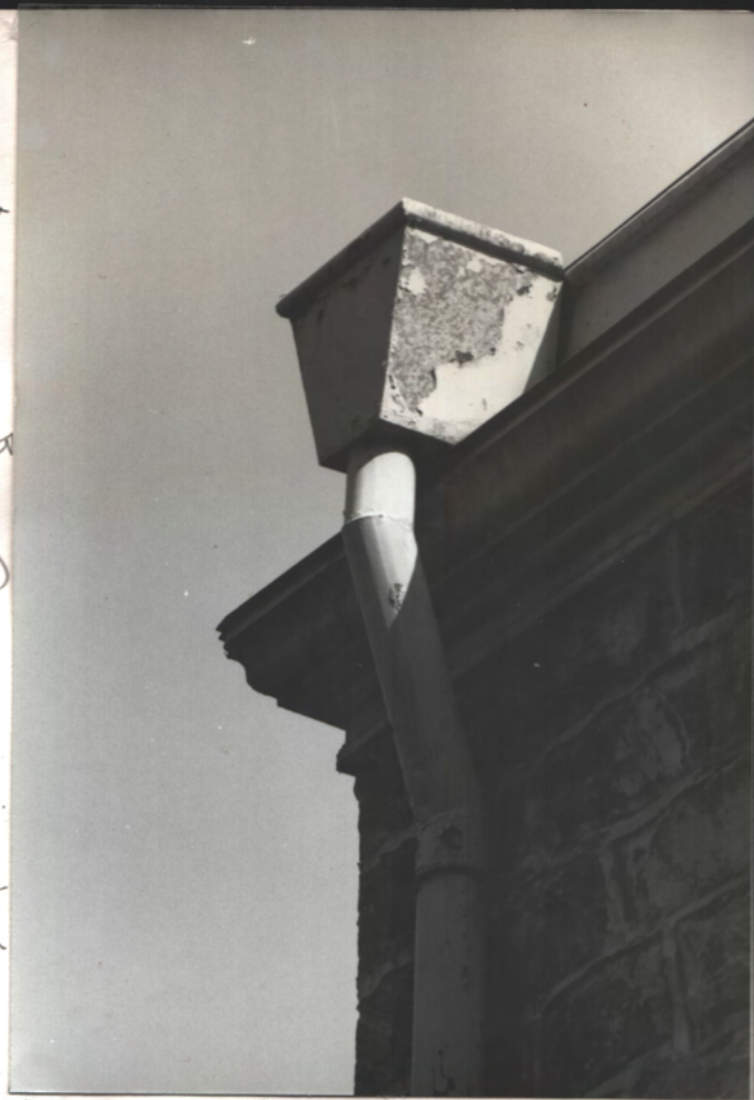
N.E. corner of S.E. - CR wing, typical leader-head ↓ Boston gutter
