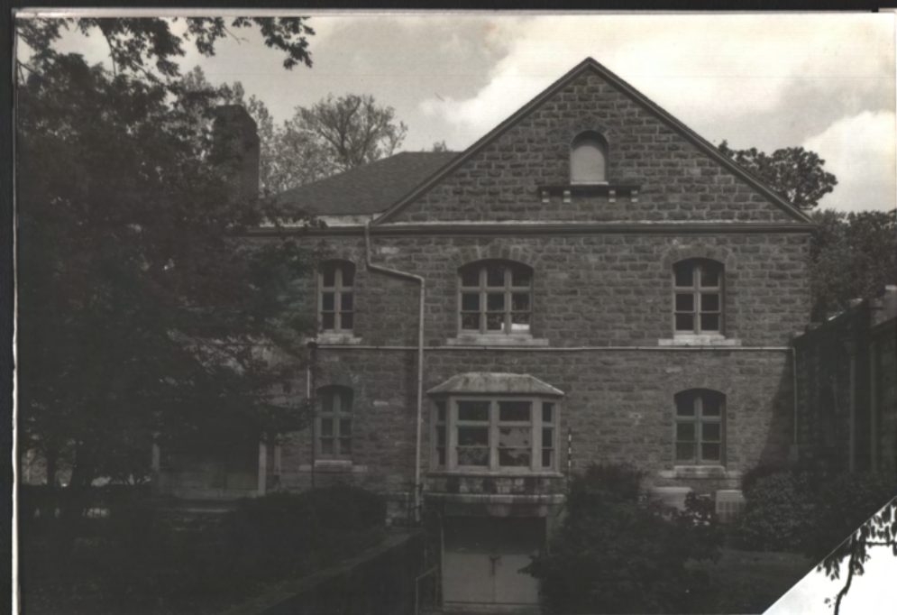
W. wall of N.E. Ad. Wing
