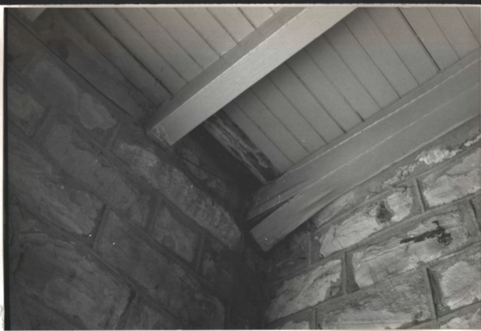
↑ not due to leaks in flat roof above + NW
