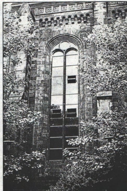
Protective plastic sheet glazing. Note how highly reflective this material is. The stained glass behind it is invisible.
