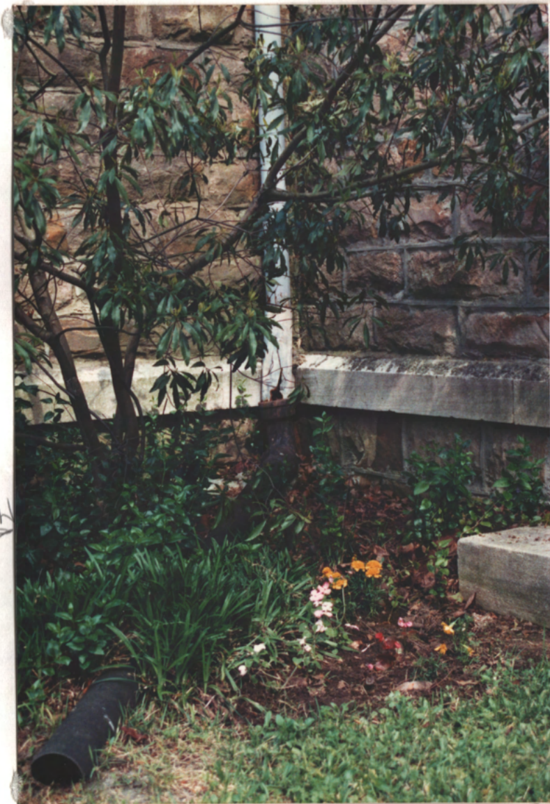
↳ plastic drain (soil forms a dam around bdy.)
