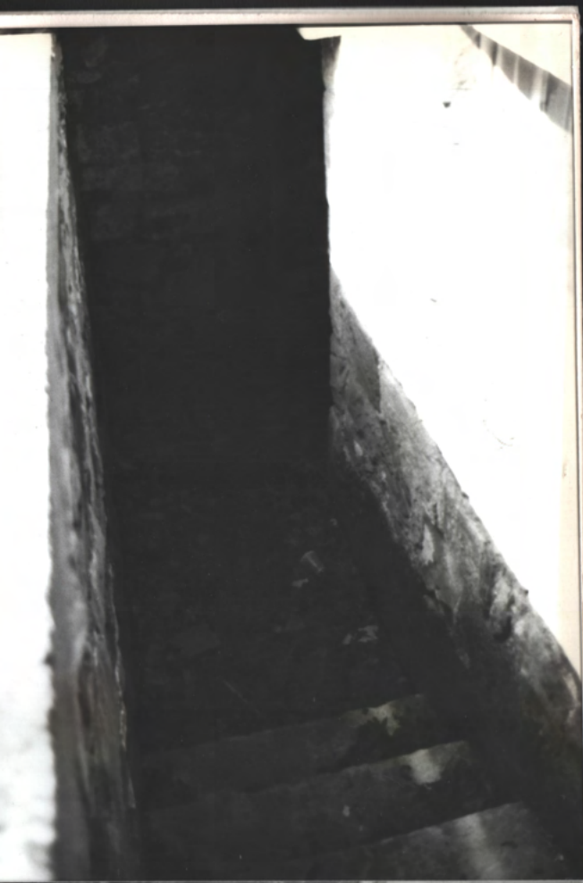
Open well at basement steps of N.E. Wing, Small - 28
