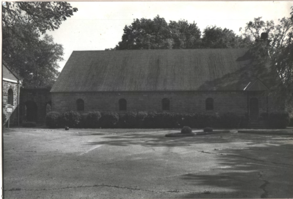
Parish Hall N. wall
