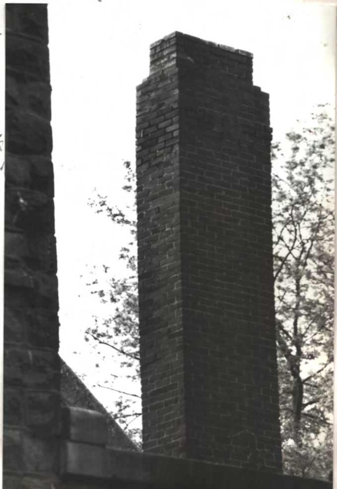
Chim. north of tower. Top 16" not like arch. drwg
