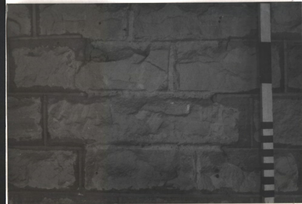
PN LM. mortar = original lt. buff color lime mortar. Dark mortar = c. 1960 portland cem.
