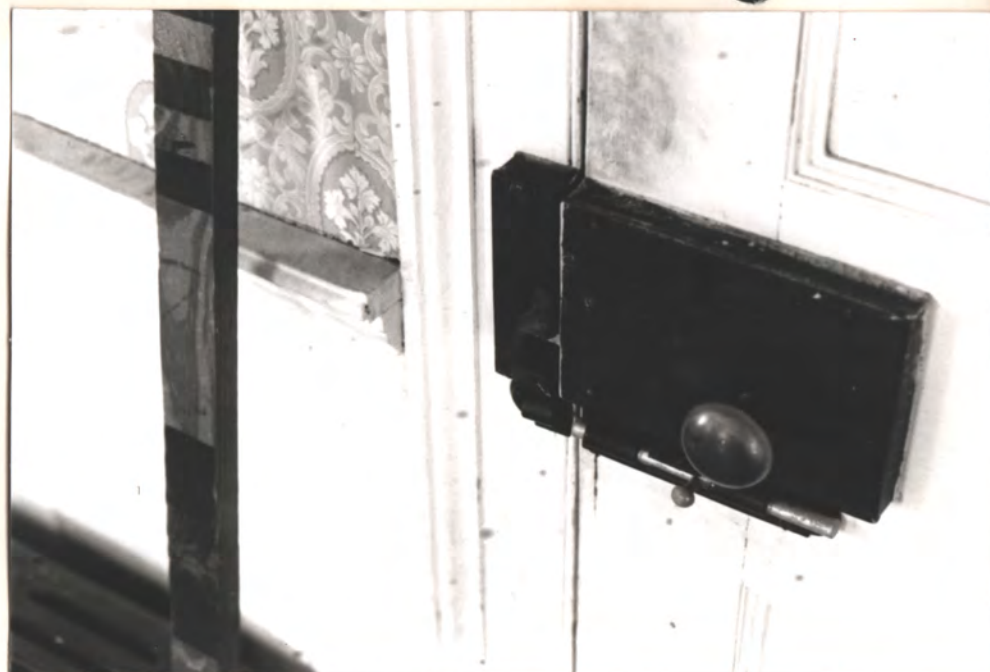
NW EAST DOOR ("Carpenter" brand lock) = Fed. slide-bolt = mod.
