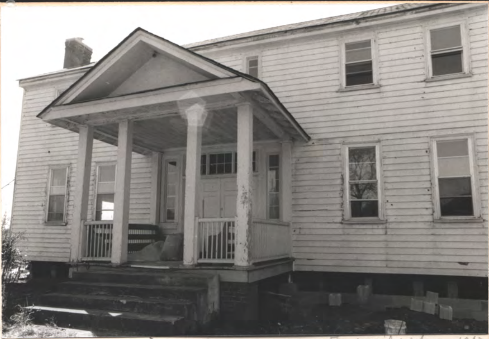
R corr steps = c. 1950's. Fl. + rail + col = c. 1840 SLOPED ROOF c. 1850's
