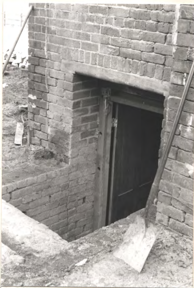
Heavily rotted (red.) Fram. under portico fl. → N
