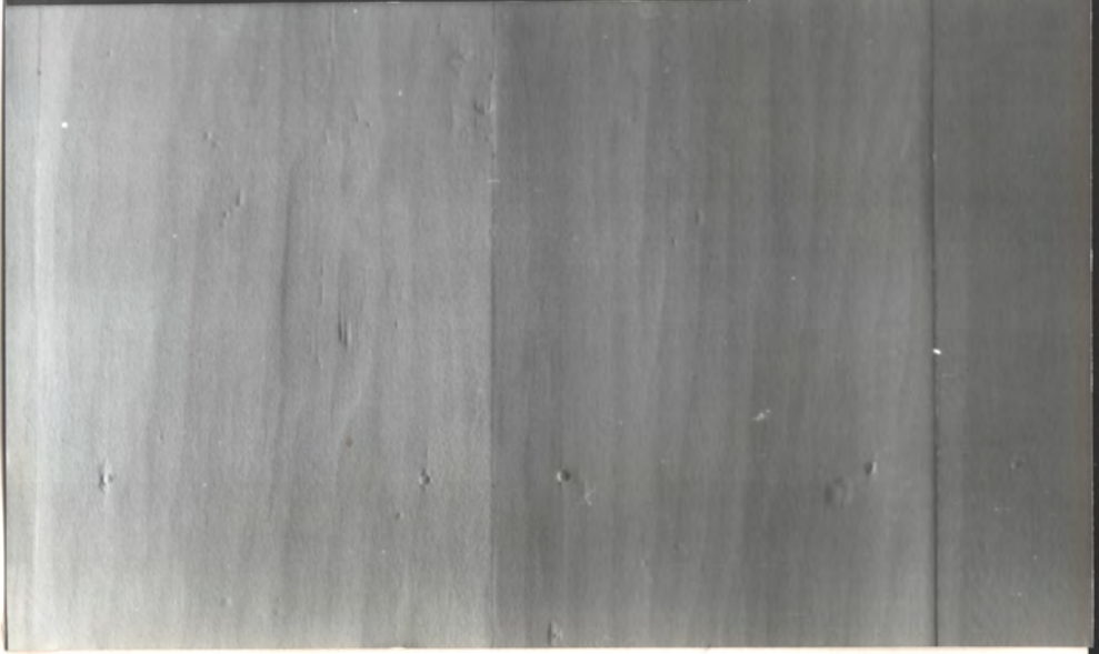
Board Ceil. in entry. Note jack-plane marks
