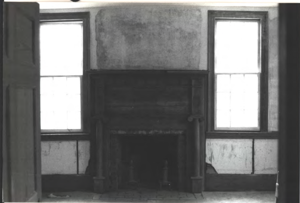
West Parlor. Note traces of missing decor. elements (side oval = sunburst, probably)
