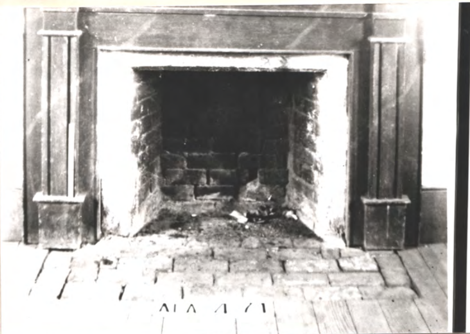
← Hearth detail - pattern = typical of 1800-1860 →
