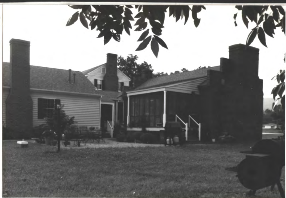
1990 Den ← * Orig. Din./Kitch → Step-gather rebuilt per 1930's HABS photos
