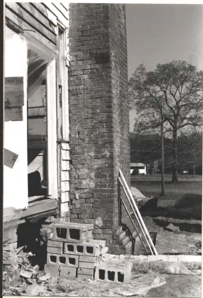
E. Chimney, Main Use, bad tech. cond. (bowed out)
