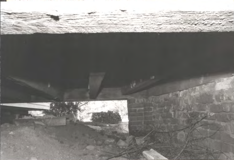
Heavily rotted (red.) Fram. under portico fl. → N
