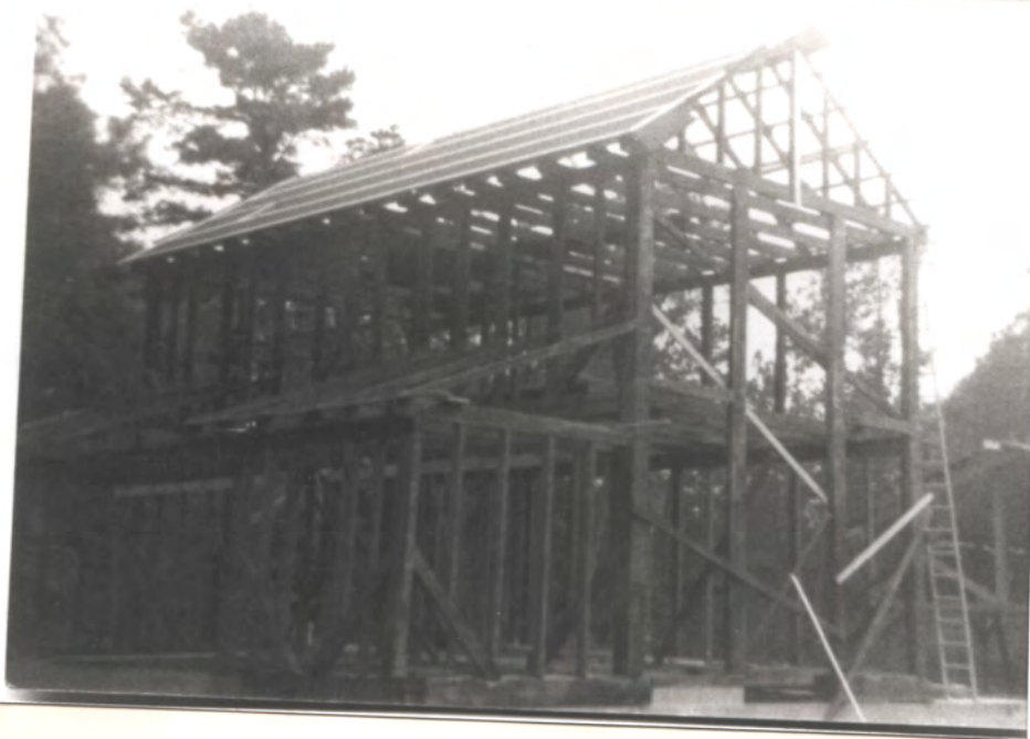
being re-erected on new site (great addn = new corner)
