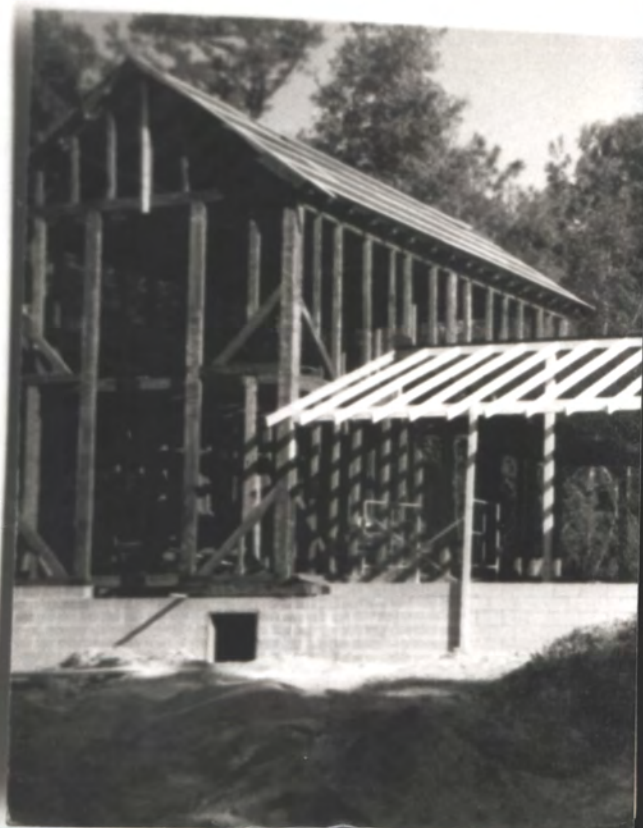
being re-erected on new site (great addn = new corner)
