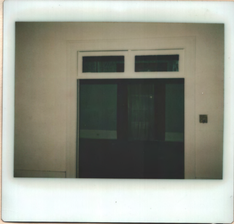
Door from west entry hall to S.W. Rm.
