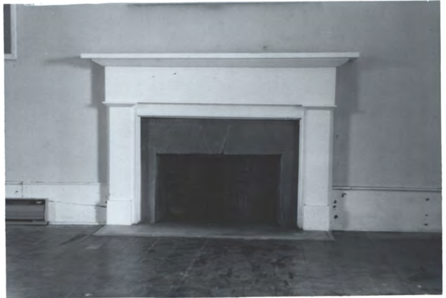
2nd fl. mantel (N. Rm) Stone facing has been sawed off to lower it (for coal-grate?) Compare w/ photo above & left.
