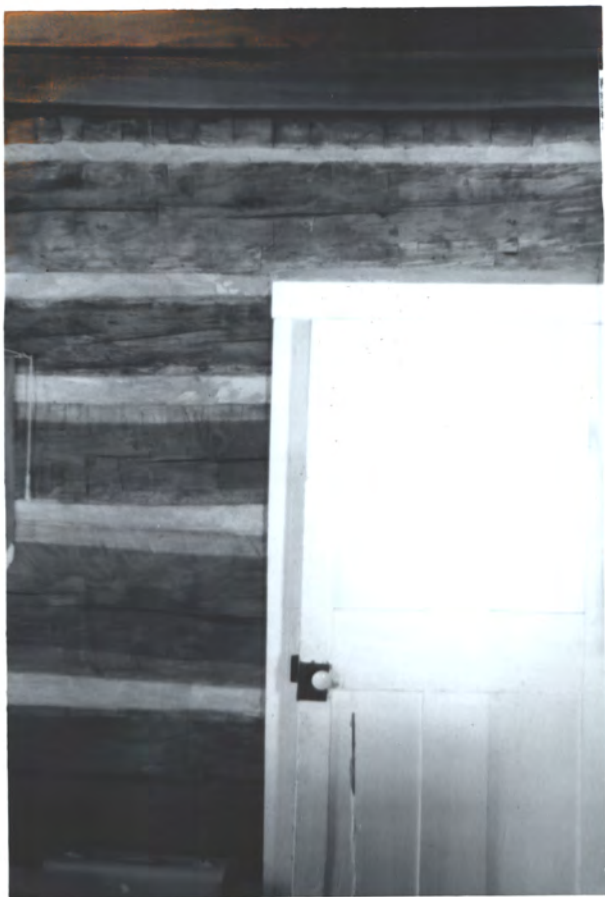
E. Wall of Log Rm. 6 pan. door, ± 8'2" h.
