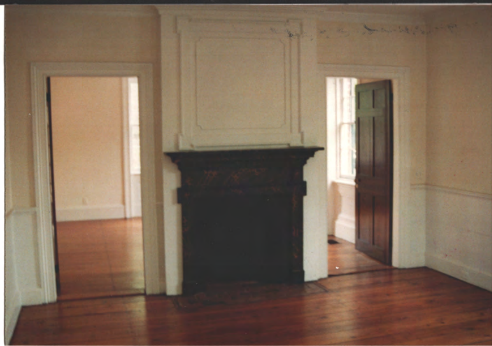
11 ← 1st fl. S.W. Corridor (c.1795) mantel & overmantel 2 doors = 1993 replace. of 2 Vic. doors & trim.
