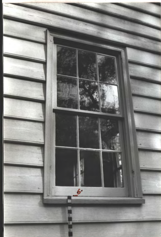
West front sash, fl. 1 S.W. Corn N ←
