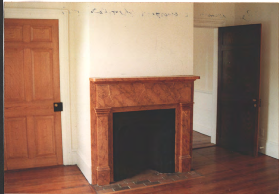
Fl. 1, SE. Rm, 1850's mantel. Door = 1993 replace. for vic. doors
