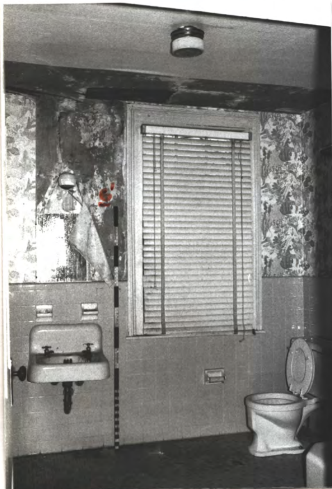
N & N.E. RM. (Remod. ca 1950's?)
