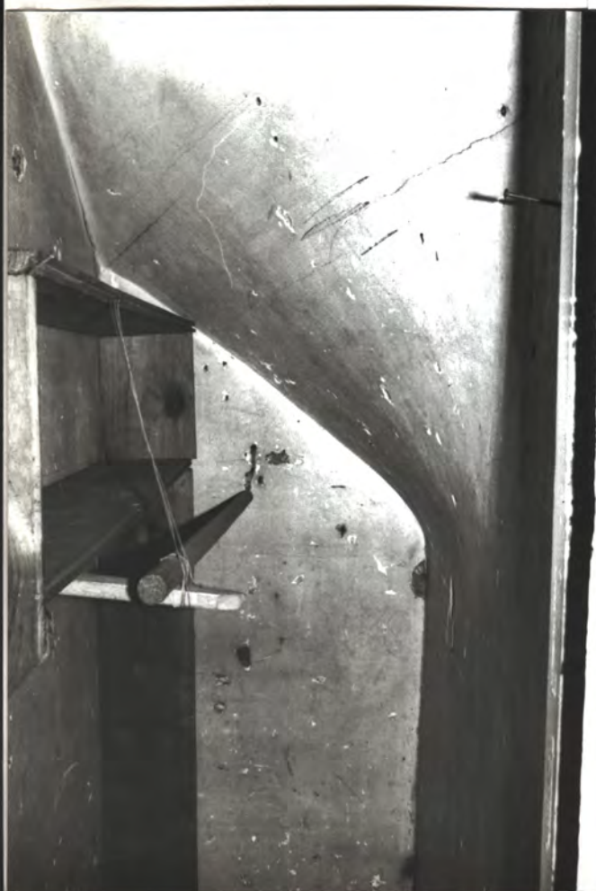
Chos. under attic stairs / note traces of Vic. modfy. to FIT Vic. Stairs
