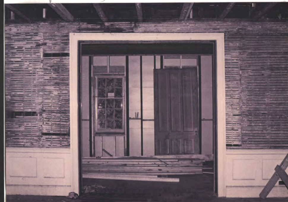
N. WALL Fed. Wainscot cut to FA Vic. door MACH. LATH AT ORIG. SASH LOC.
