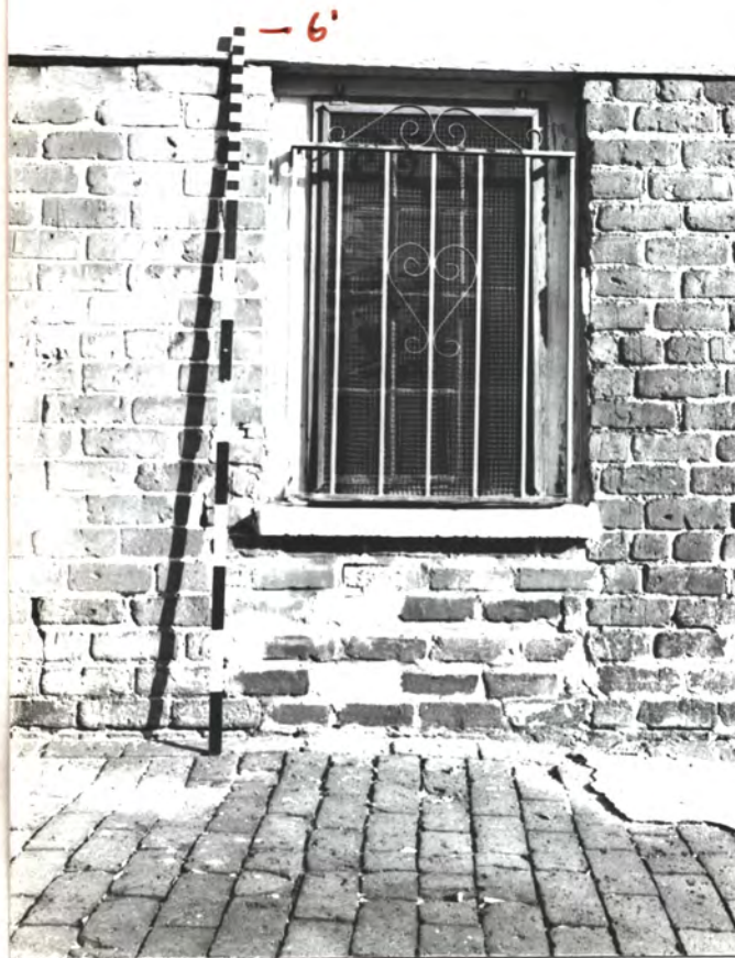
7 of 64 S. Window by S.C. corner. Was a door at some point
