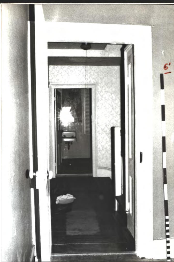
N ↑ S.E. RM., door to stair
