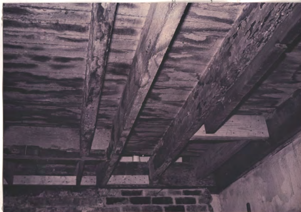
In later shed added. Narrower framing + smaller joints
