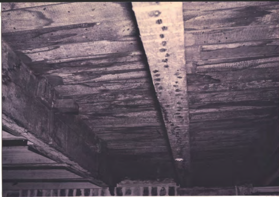
Note both of plaster traces Note pit-sawn pl. planks (some may be sash-sawn. Irregular = pit-sawn)
