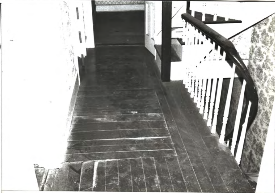
Chos. under attic stairs / note traces of Vic. modfy. to FIT Vic. Stairs
