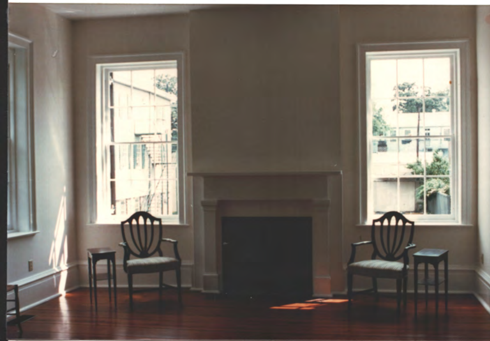
Level 2 S.E. parlor (mantel replicated from those on levels 3 & 4 = all same, except widths
