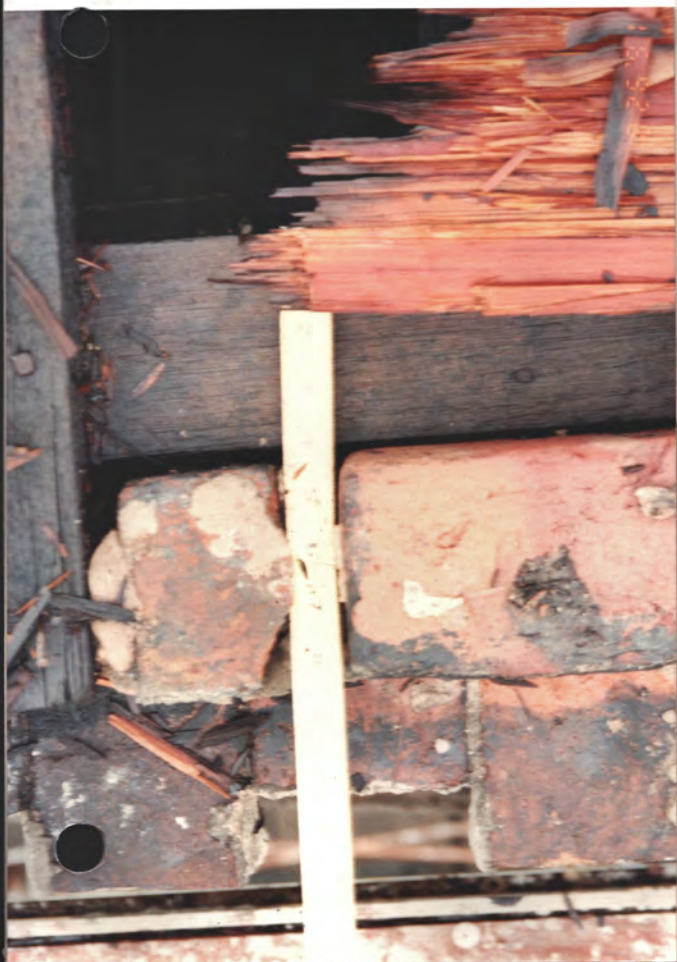
Rafter extn. over brick dentils
