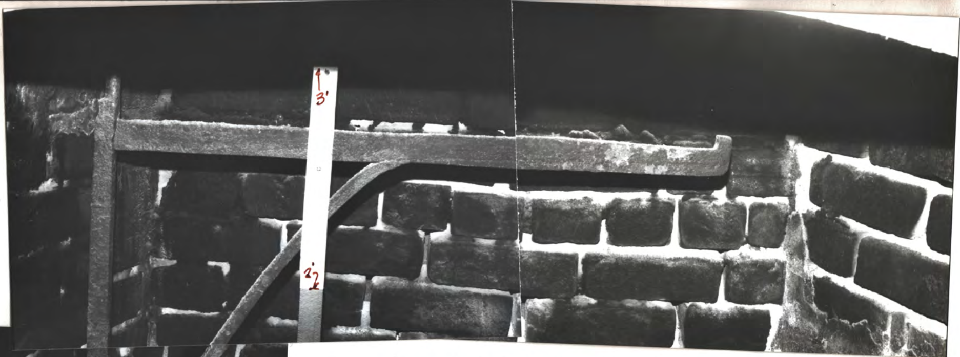
Level 1 S.E. Room fireplace Cooking crane looks original. F.P. bricks & mortar looks original
