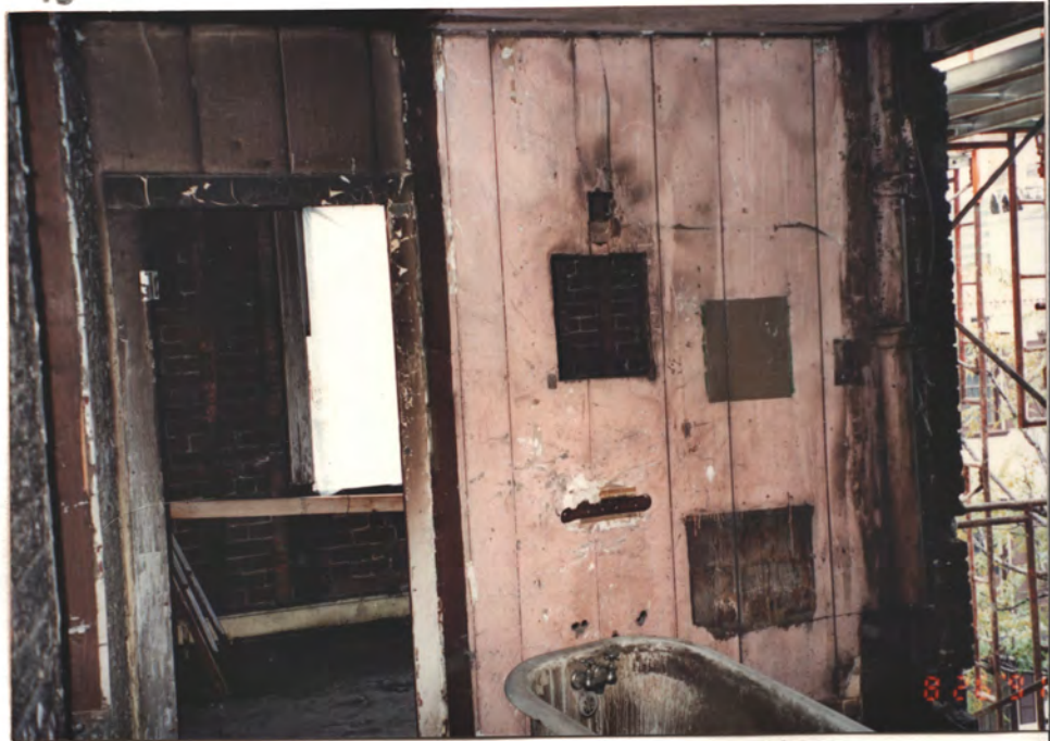
level 4 rear porch
