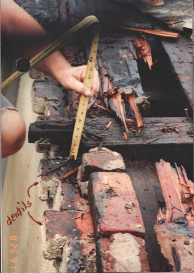
Rafter extn. over brick dentils
