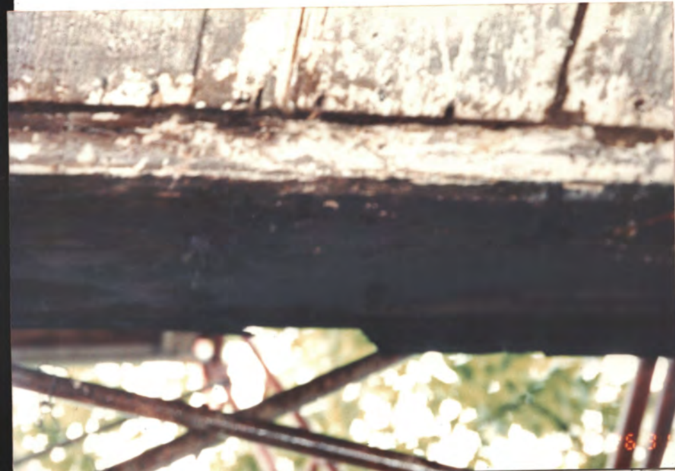
5 looking up at new porch w/d. beams → N
