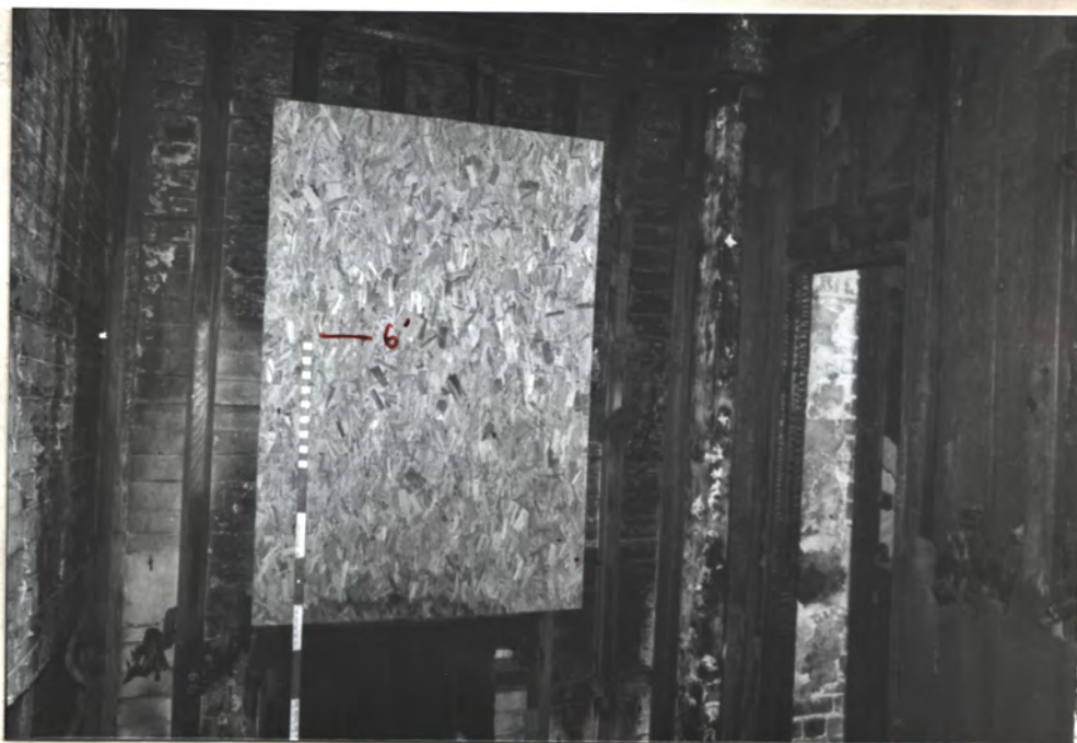
③ Enclosed back porch → N P to N.W. stair
