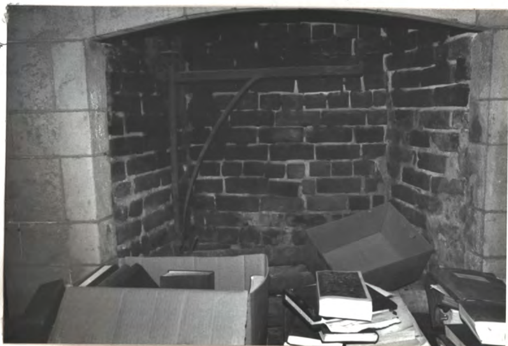
Level 1 S.E. Room fireplace Cooking crane looks original. F.P. bricks & mortar looks original
