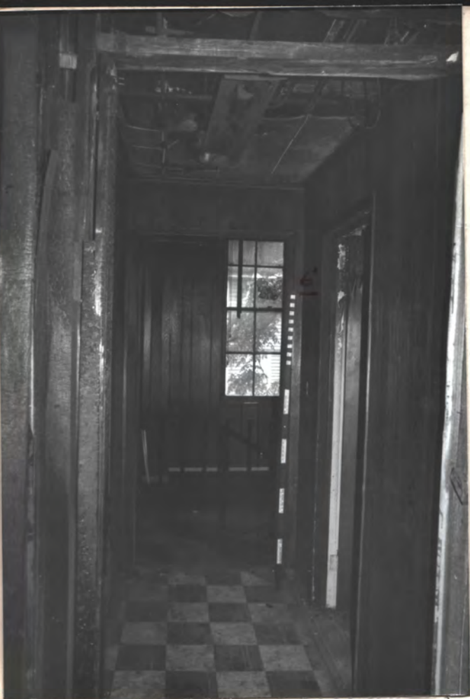
① ↑ to S.W. Rm., w/ c. 1960's spiral stair → N
