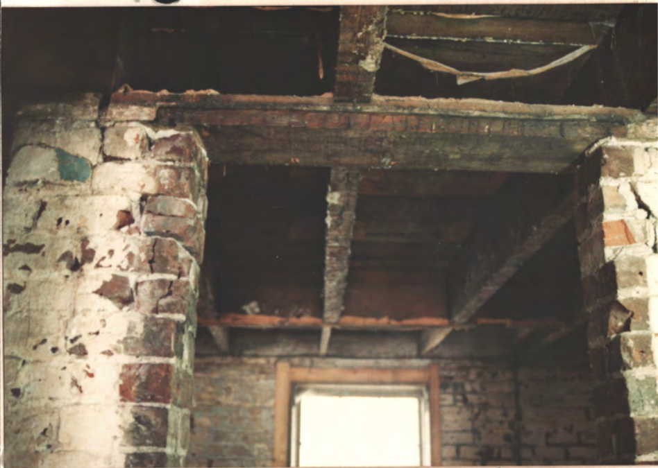
24 Typical beams between basement cols 26
