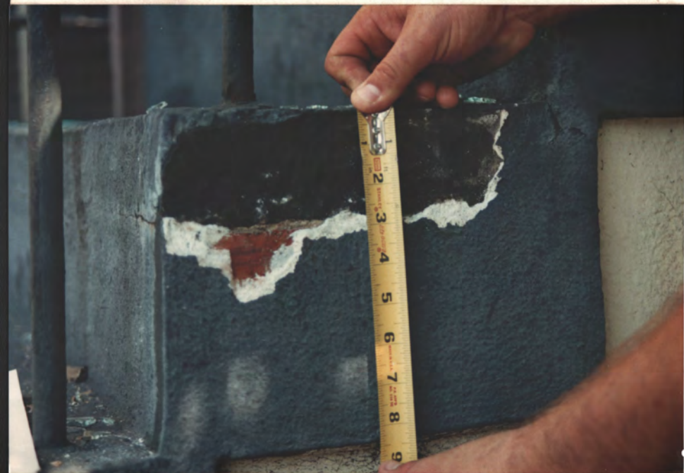
5 → H ± 2 3/4" stone trend on brick step behind c. 1960 "gunnite" stucco, Front stoop.
