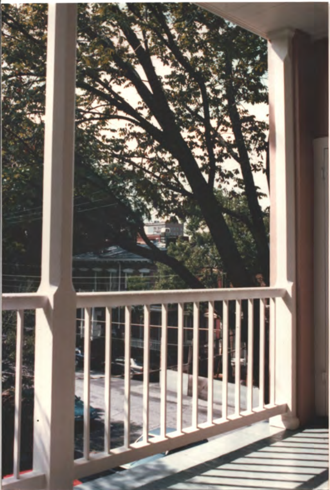
↘ NW Back west porch, level 3
