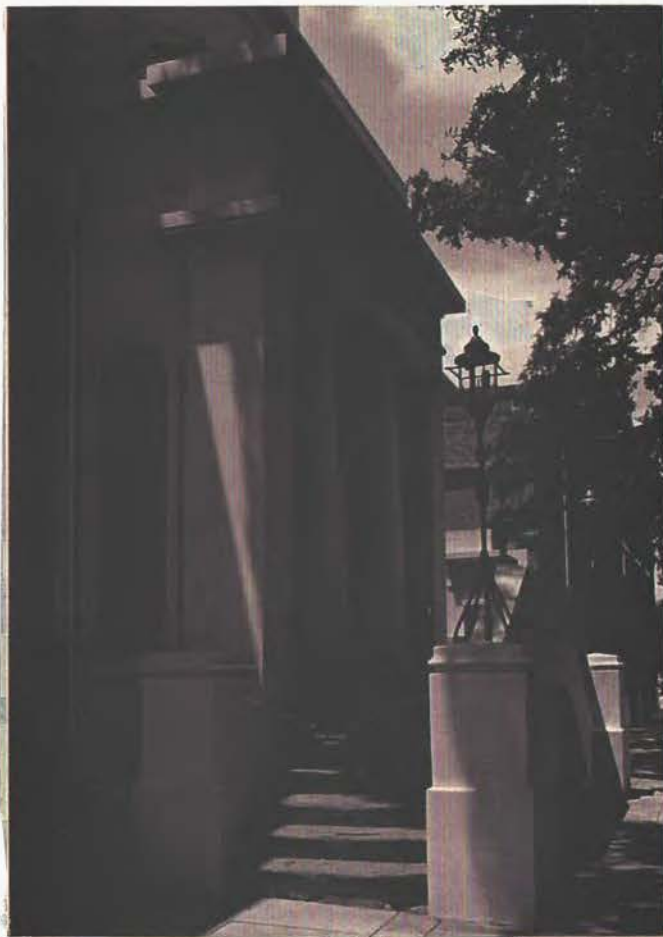
ext. restw. by HP Jones, FMB 1995-97 for "Ships of the Sea" Museum (MVA/Lane) (Int. by others) Lamps per a hist photo of Wm Jay's early bank in Savannah.
