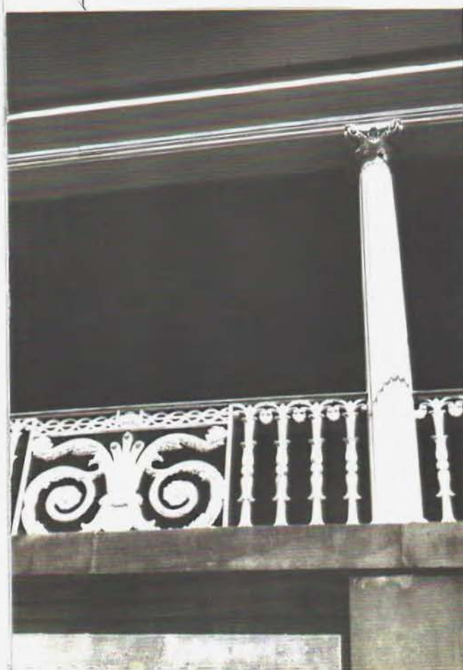
cast iron balcony railing
