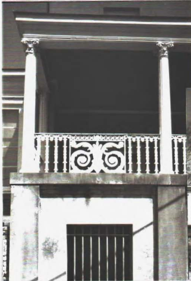
cast iron balcony railing
