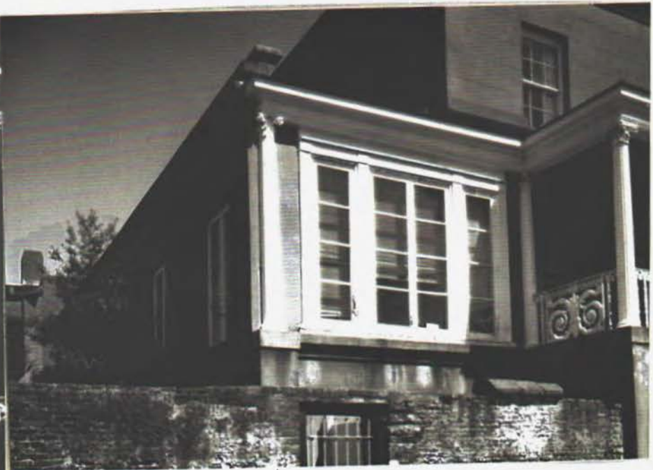
This col. not here originally (has slot for rail)
