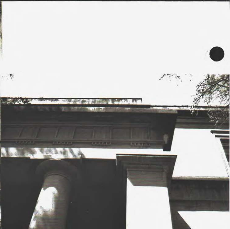
→ W balustrades of rail = c. 1972 material. Balustrades too far apart - probably not original design
