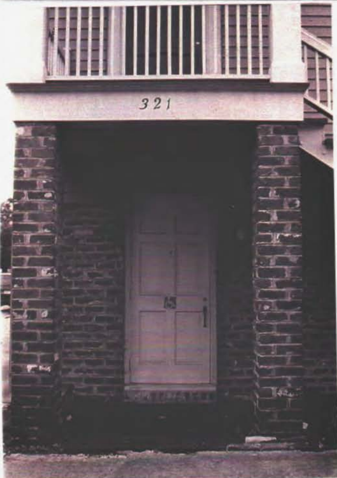
1920's brick - entire level & work NW
