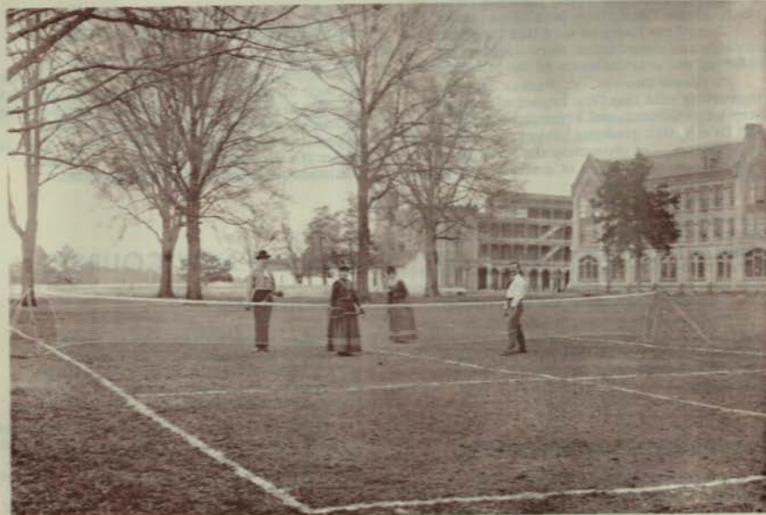
photograph courtesy Oil and Gas Board
